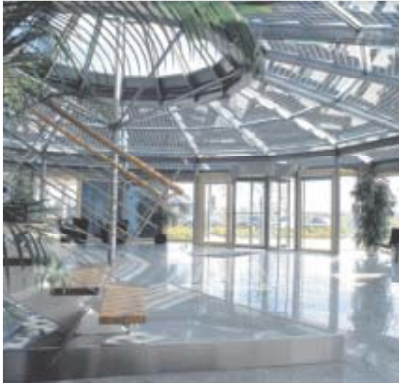
PV roof-lights at the JPS - Presse and Vertriebs GmbH buildings in Meckenheim, Germany
