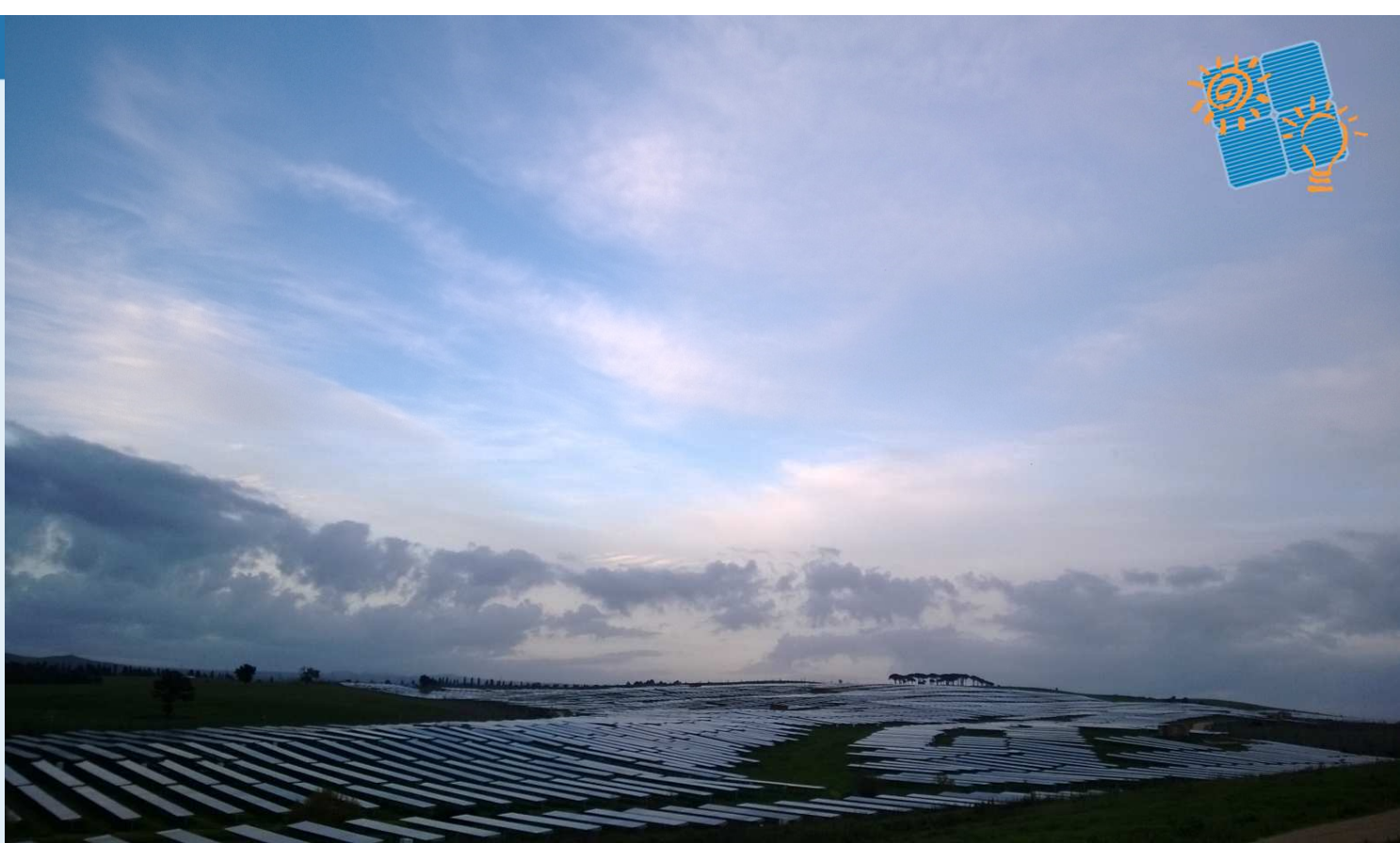
Front Photo © TÜV Rheinland Energy
