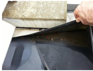
Fig. 17: Localized low spot for water [7].
