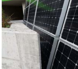
Fig. 10: Shading due to poor design [3].
