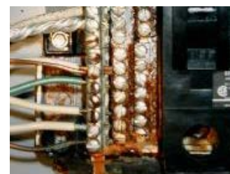
Fig. 8: Corroded interconnection [12]
