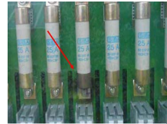
Fig. 27: Triggered string fuse [4].
