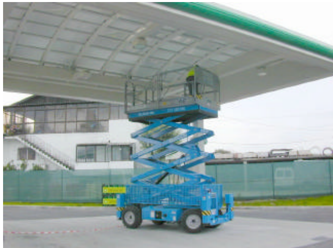
Photo 1. - Thin film photovoltaic modules integrated into BP filling station
