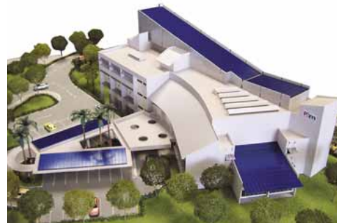
PTM's showcase Zero Energy Office in Malaysia incorporates 91 kW of PV into various roofing elements. The project is due for completion in first quarter 2007.
