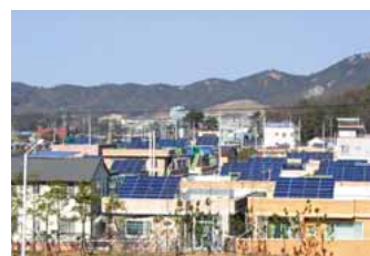
'Green Village' with 97 kW on 46 homes in Kwangju Metropolitan City under Korea's 100 000 Rooftop Programme.
