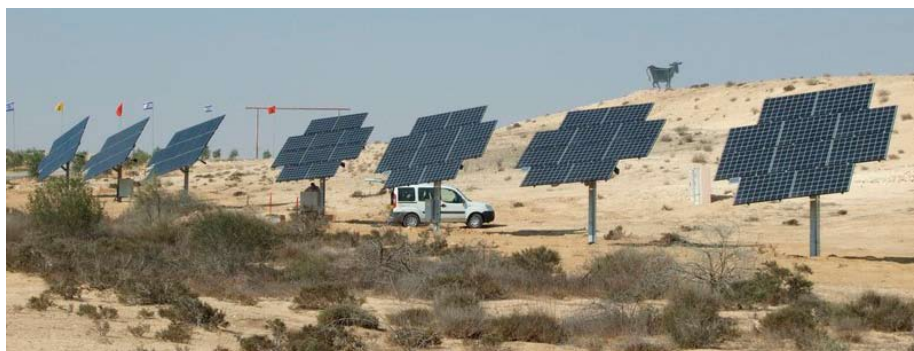
16 kW tracking system at a farm in the Negev.
