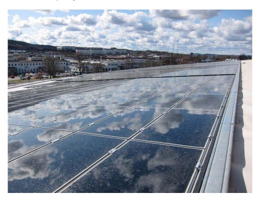
Figure 4: A thin film PV system installed at the roof top of the public bath Rosenlundsbadet, Jönköping (Courtesy Glacell)
