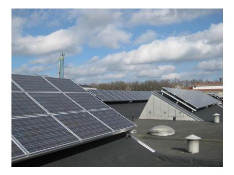
Figure 1: An example of a grid-connected roof top mounted PV system located at Kungsmadskolan, Växjö (Courtesy Mats Andersson)
