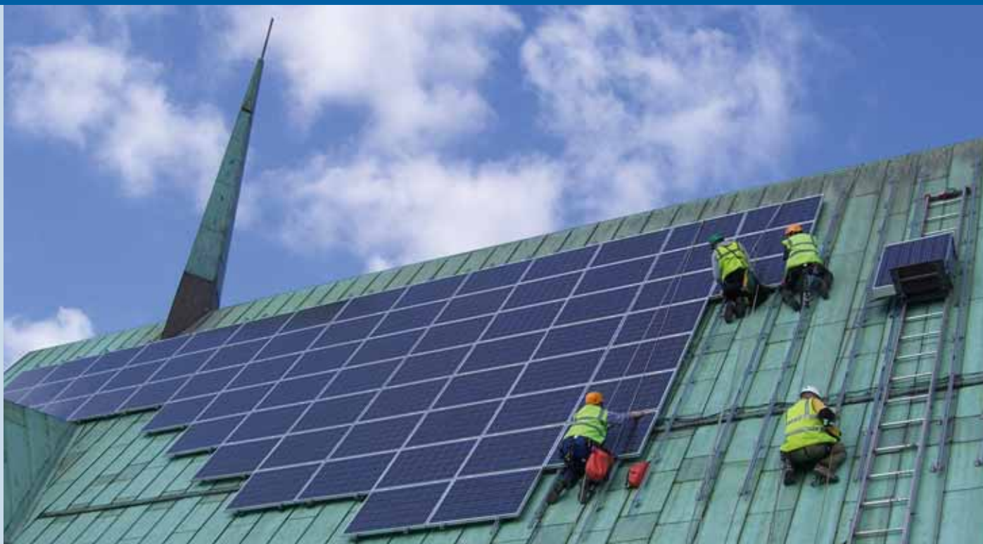
Fig. 1 - Finalising a 18,4 kWp at St. Francis of Assisi Church in Rochester (photo: Solstice Energy Ltd).
