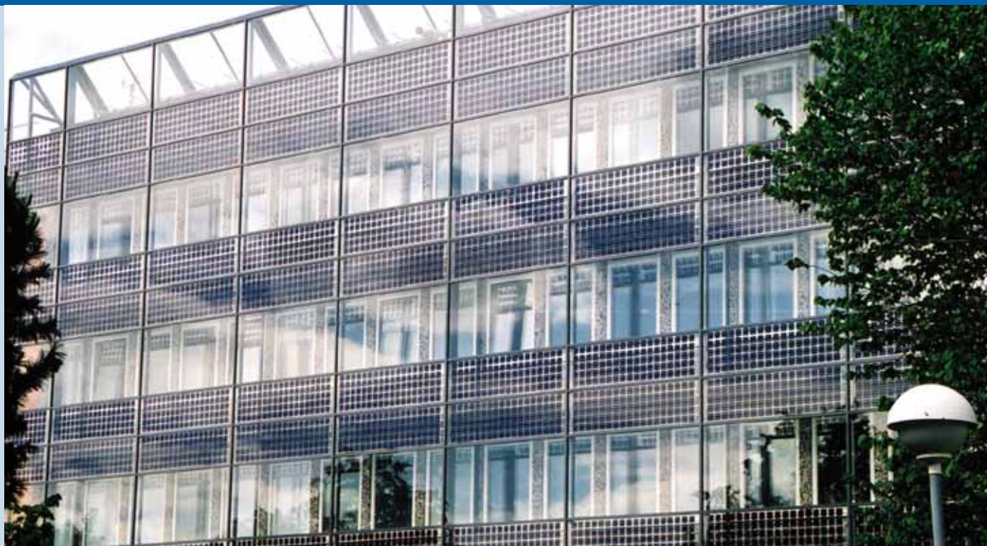
Fig. 1 - Solar panelled wall at NTNU in Trondheim. Although central Norway is only about 500 km south of the Arctic Circle, solar energy may be a viable energy source for more than just isolated log cabins even in these high latitudes. To test this on large-scale buildings a double facade with photovoltaic (PV) panels has been built on the campus of the Norwegian University of Science and Technology in Trondheim. A monitoring programme has been started to evaluate the performance of the PV panels and their influence on the indoor air climate.
