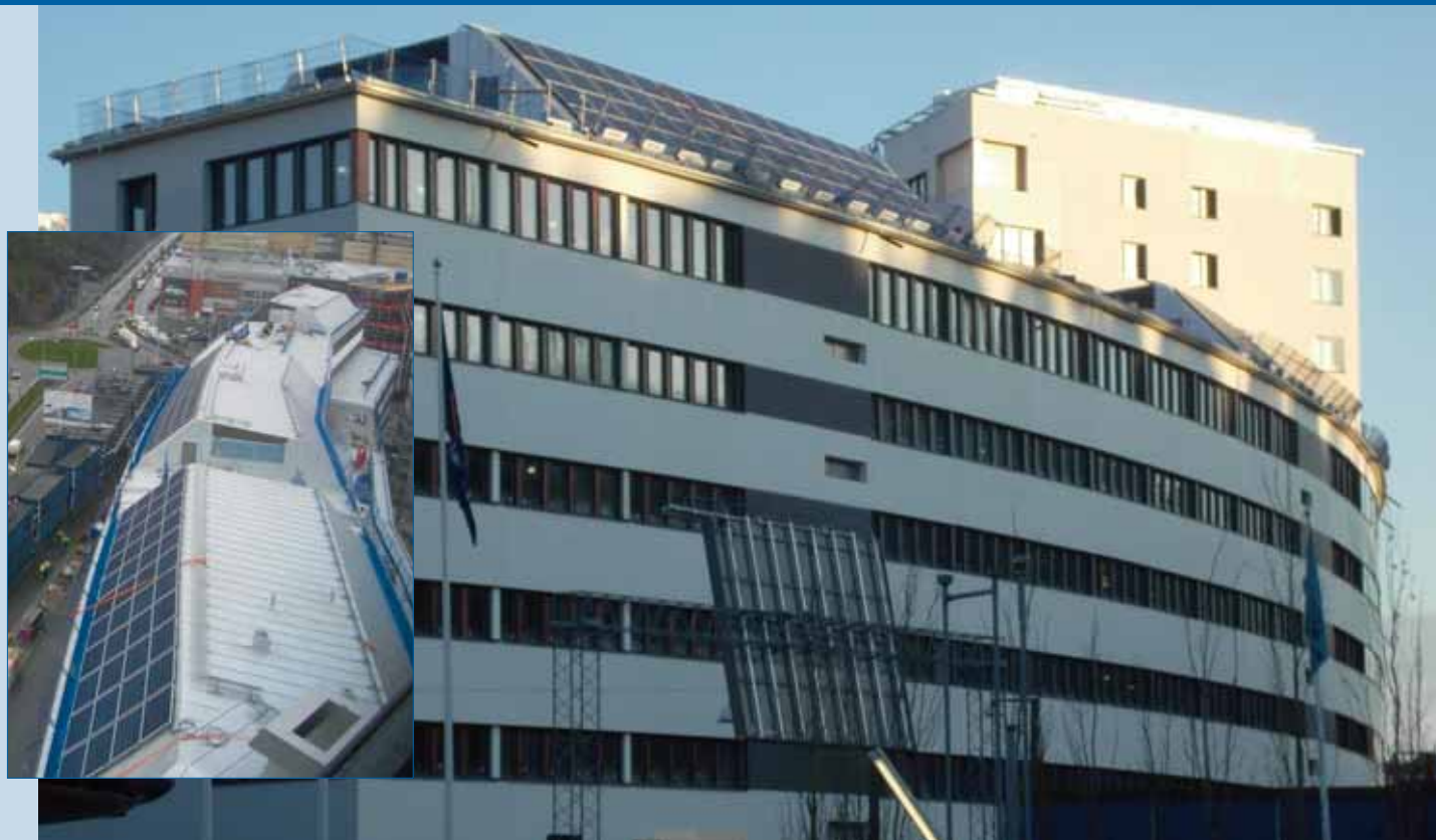
Fig. 1 - Roof top PV system on new office building in Hammarby Sjöstad, Stockholm (photo: Fasadglas AB).
