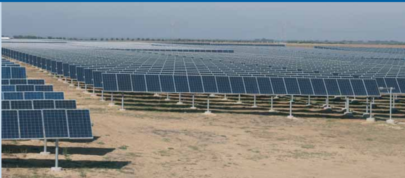
Fig. 1 - 10 MW one-axis tracking c-Si Power Plant in Ferreira (photo Tecneira).
