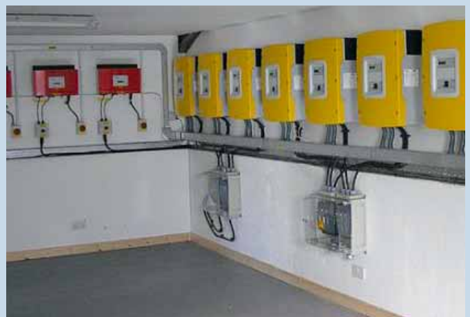
Fig. 1 - The power generation system of the Isle of Egg, Scotland, consists of 10 kWp PV, 3 hydro plants (100 kW, 2 x 6 kW), 4 Wind turbines (4 x 6 kW) and 2 Diesel gensets (2 x 80 kVA). Each of these sources has been sensitively sited to cause minimum visual and physical impact upon the island's landscape. Twelve Sunny Island 5 kW inverters are used connected in four three phase clusters to provide a total output rating of 60kW. A Multicluster Box enables the communication among the inverters and provides contactors for the connection to the island grid, to the PV and Wind inverters and the back-up gensets. Each cluster is connected to a 48V 2242 Ah (C10) battery bank consisting of 24 batteries. 87 inhabitants owning 37 residential and 5 commercial properties must be supplied by the system. The peak demand has been limited with the approval of the residents; domestic and small business supplies have been restricted at 5kW, and larger business supplies at 10kW.
