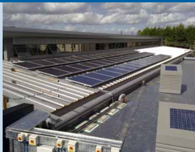
Fig. 5 - 9,7 kWp PV installation - Hamworthy Library, Poole (photo: Sustainable Energy Installations Ltd).
