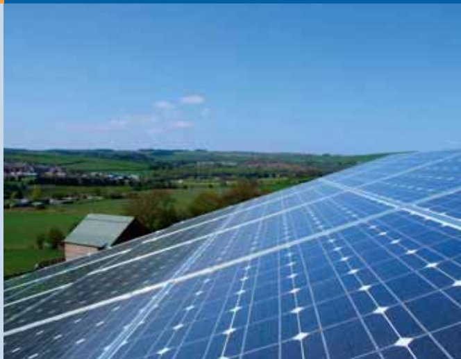
Fig.6 - 4.3 kWp retrofit domestic roof installation, County Durham (photo: Cleaner Air Solutions Ltd).
