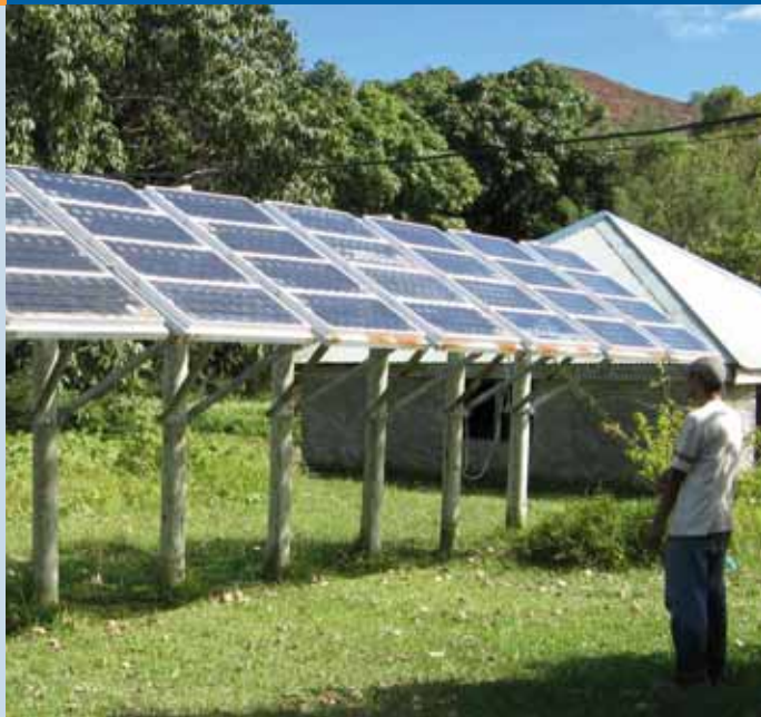
Fig. 5 - Solar Panel array for a community PV service system on Wallis and Futuna, substitution for diesel consumption (photo IED 2009).
