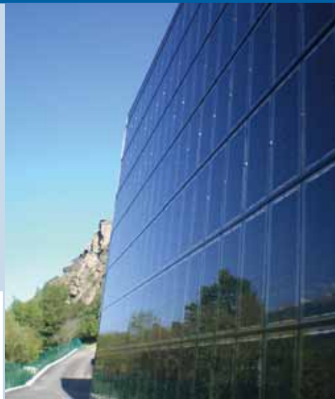
Fig. 3 - 49 kW PV system installed on the façade, Laces (BZ).
