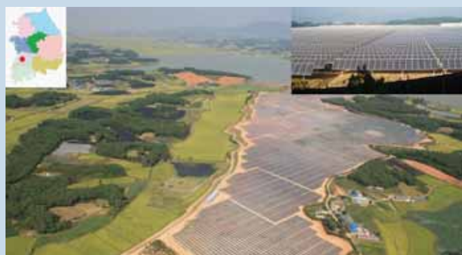
Fig. 3 - The 15 MW PV power station installed in Gochang-gun, Jeolla North Province in September 2008 under the FIT program. The systems are operating by tracking mode.
