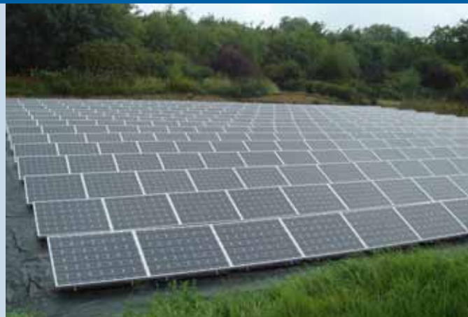
Fig. 3 - 70 kWp Ground Mounted PV system near Cheltenham (photo: Apollo Renewables).
