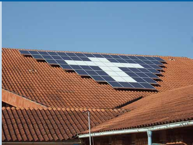
Fig. 2 - Solar generator: 81 solar modules of 100 Wp, Schott GT-FT 100; Inverter: Sunny Boy 3 800 and Sunny Island 4 548, in total 6 units, SMA; Battery: 3 banks of 800 Ah, 48 Volt, OPzS Hoppecke, at the Community of the Vincentian Sisters in Mbinga, Tanzania.
