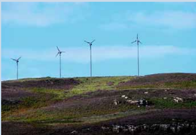
Fig. 1 - The power generation system of the Isle of Egg, Scotland, consists of 10 kWp PV, 3 hydro plants (100 kW, 2 x 6 kW), 4 Wind turbines (4 x 6 kW) and 2 Diesel gensets (2 x 80 kVA). Each of these sources has been sensitively sited to cause minimum visual and physical impact upon the island's landscape. Twelve Sunny Island 5 kW inverters are used connected in four three phase clusters to provide a total output rating of 60kW. A Multicluster Box enables the communication among the inverters and provides contactors for the connection to the island grid, to the PV and Wind inverters and the back-up gensets. Each cluster is connected to a 48V 2242 Ah (C10) battery bank consisting of 24 batteries. 87 inhabitants owning 37 residential and 5 commercial properties must be supplied by the system. The peak demand has been limited with the approval of the residents; domestic and small business supplies have been restricted at 5kW, and larger business supplies at 10kW.
