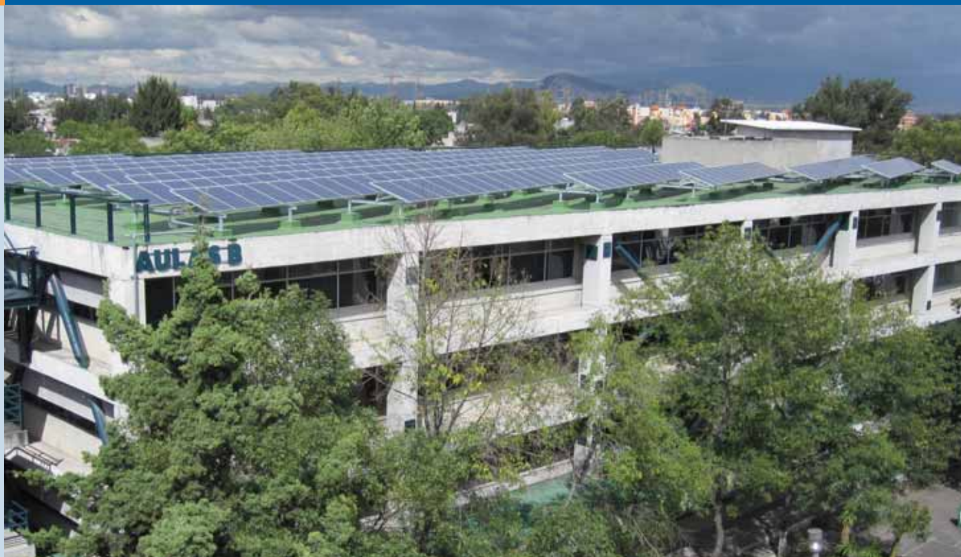
Fig. 2 - 60 kWp Grid Connected System at the Autonomous Metropolitan University Campus Iztapalapa (photo: UAM-I).
