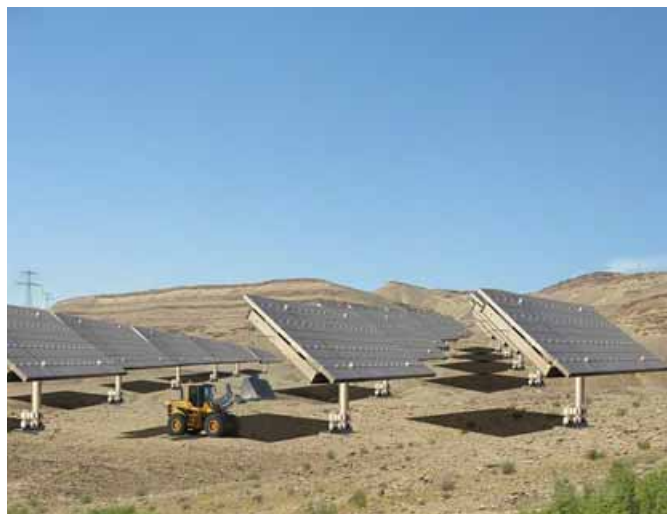
Fig. 2 - Simulation of MST solar power plant on rocky and unleveled terrain.
