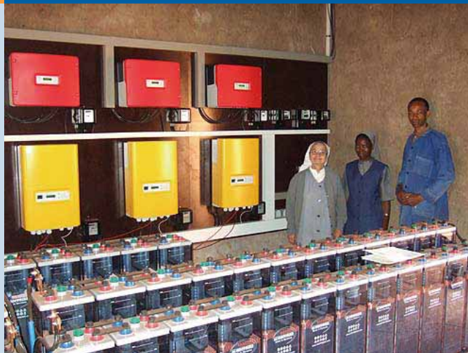
Fig. 2 - Solar generator: 81 solar modules of 100 Wp, Schott GT-FT 100; Inverter: Sunny Boy 3 800 and Sunny Island 4 548, in total 6 units, SMA; Battery: 3 banks of 800 Ah, 48 Volt, OPzS Hoppecke, at the Community of the Vincentian Sisters in Mbinga, Tanzania.
