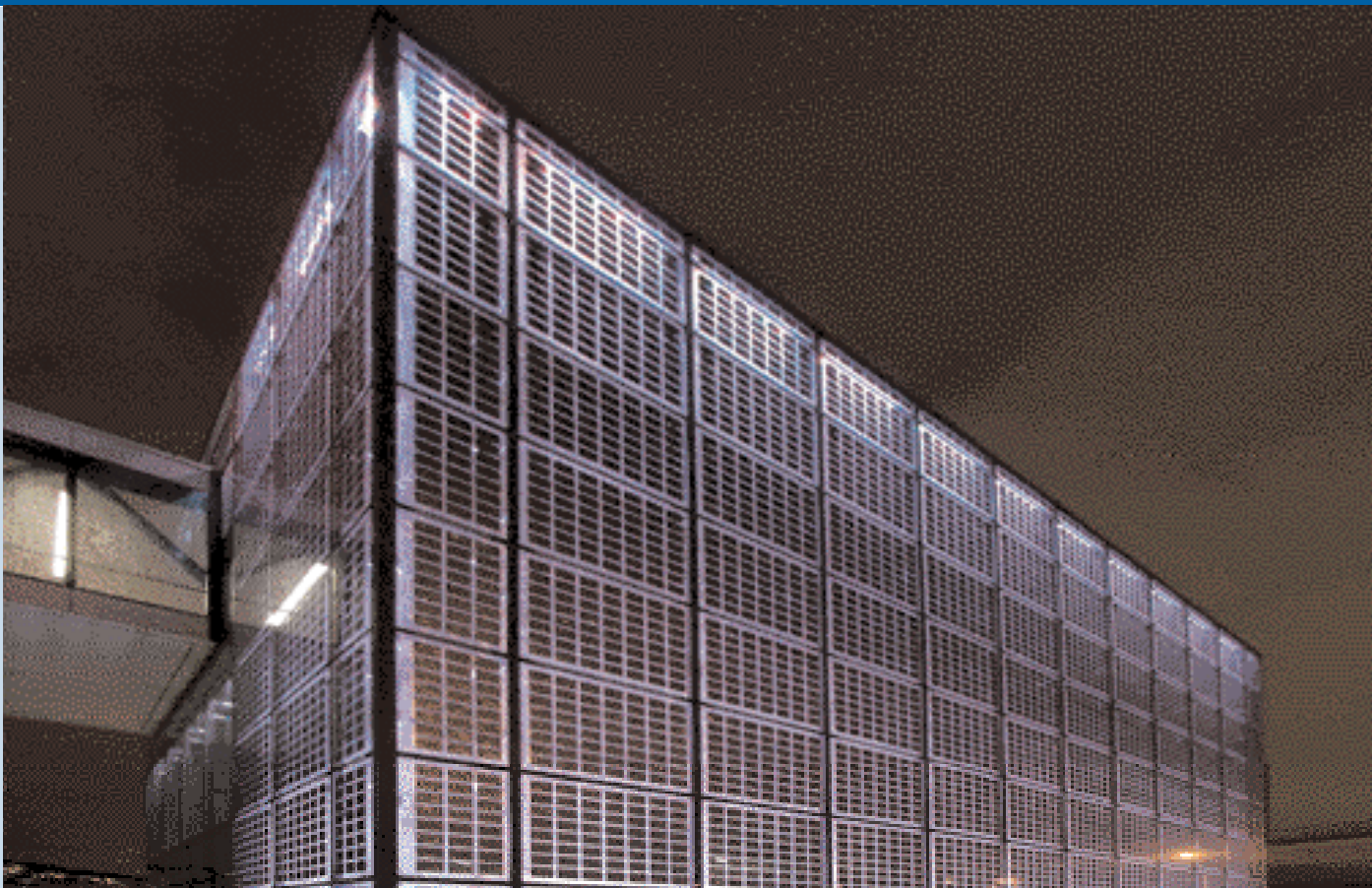
Fig. 1 - Photovoltaic Facade in Zurich. The corporate building of Migros cooperative in Zurich comprises a successful building integration of a 38 kW facade system (photo + project: energiebüro@ag / Zurich / Switzerland - for solar power plants).
