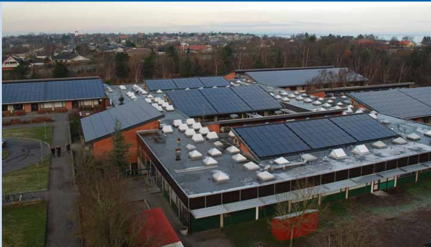
Fig. 1 - School in the Skive municipality, 300 kWp single crystalline modules integrated in the roofs.
