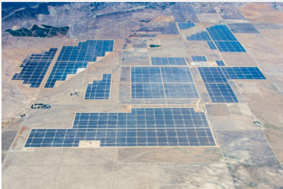
Topaz Solar Farm, CA, USA (550MW AC , CdTe) (©First Solar, Inc.)
