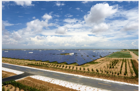
Longyangxia, Qinghai, China (520MW DC/AC , c-Si) (©Yellow River Hydropower Company)
