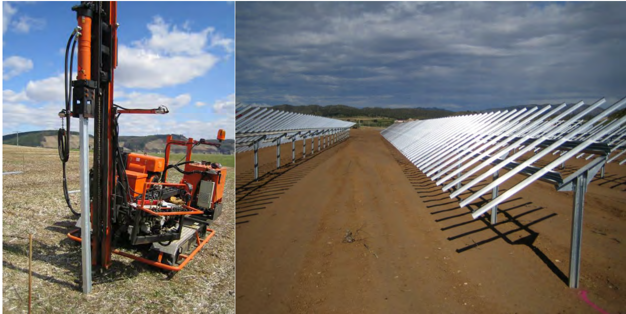
Fig. 1.1-20 Static-Pressure Poles
