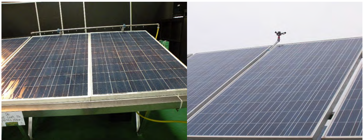
Fig. 1.1-14 Cleaning by water pipes
