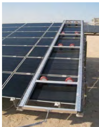
Fig. 1.2-4 Manual dry brush trolley cleaning method deployed in the Middle East 12)
