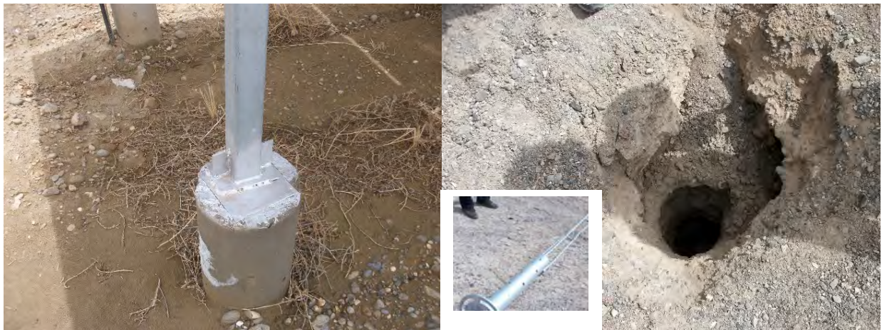
Fig. 1.1-21 Concrete poles by digging a hole and putting a pole
