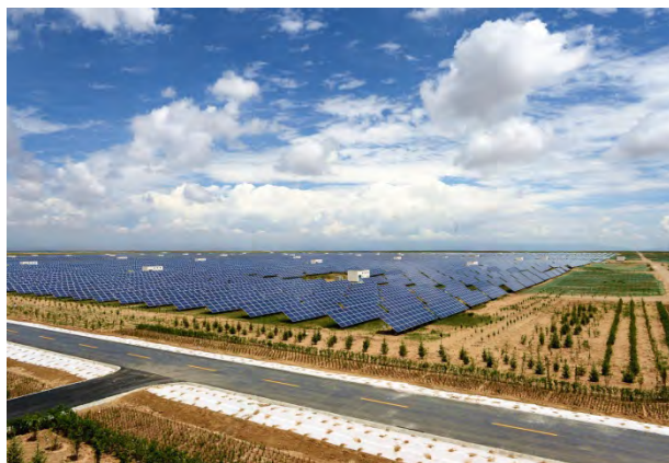
Fig. 1.1-3 The largest PV power plant in Gonghe, Qinghai, 520 MW (courtesy of Yellow River Hydropower Company)
