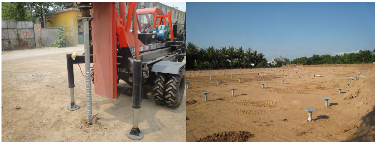
Fig. 1.1-19 Screw-drilling poles
