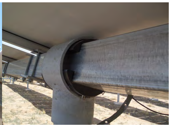
Fig. 1.1-11 Details of the Bearing-Free Turning Axis at APS Test Field
