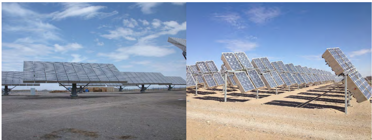
Fig. 1.1-6 10 MW 500x CPV and 60 MW 1000x CPV Power Plan in Qinghai
