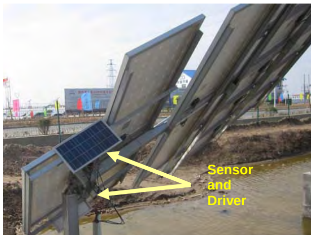
Fig.1.1-9 Passive Drive Sun-Tracker
