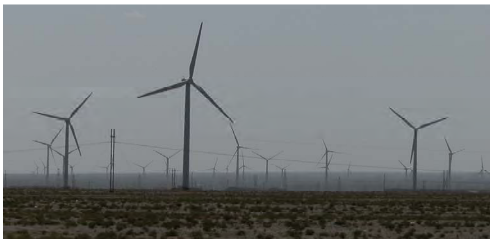
Fig. 6.1-7 Part of a 1.74 GW VLS-Wind plant at Yumen, Gansu Province, China (Photographed by DF in July 2012)
