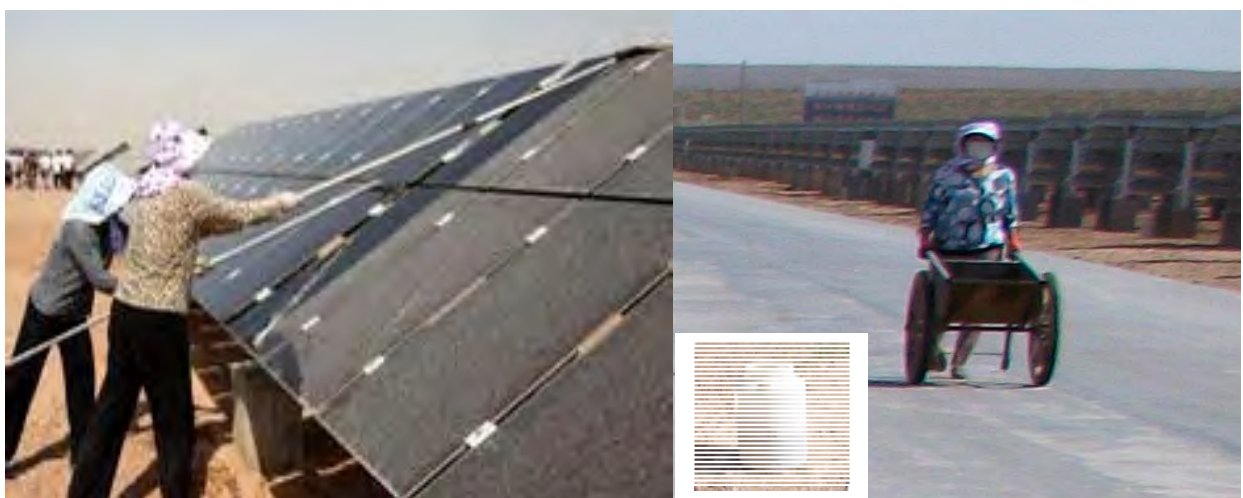
Fig. 1.1-17 Cleaning by three-women solution
