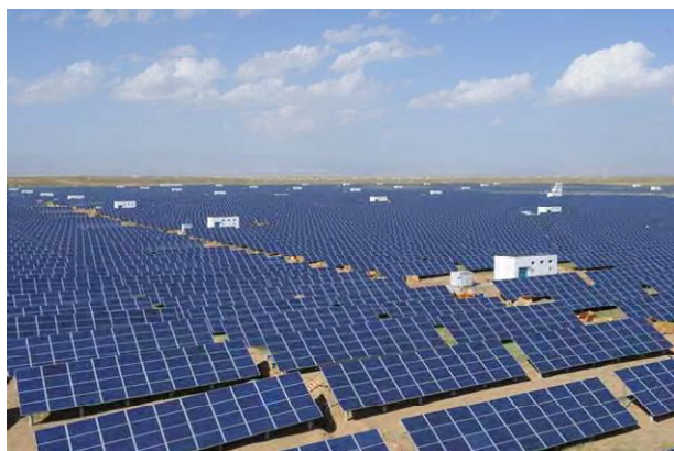
Fig. B.1-7 Longyangxia dam, Qinghai, China (520MW DC/AC , c-Si) combined with 1,28 GW Hydro power
