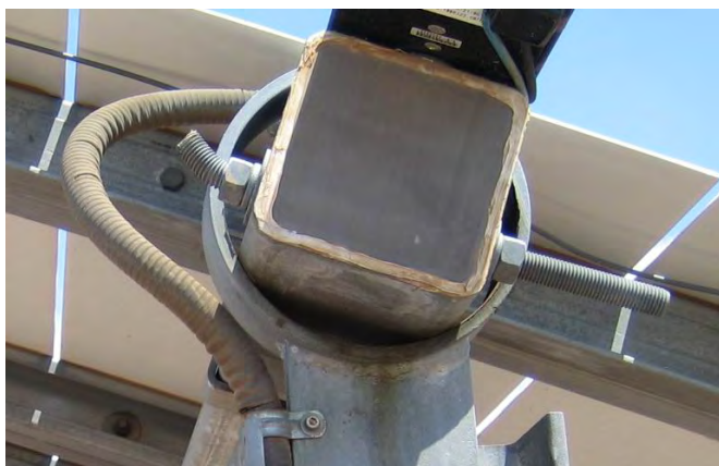
Fig. 1.1-11 Details of the Bearing-Free Turning Axis at APS Test Field
