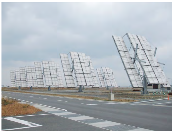
Fig. 4.1-5 A 160 kWp Daido Steel CPV system on Kyushu Island [Courtesy of Daido Steel ]
