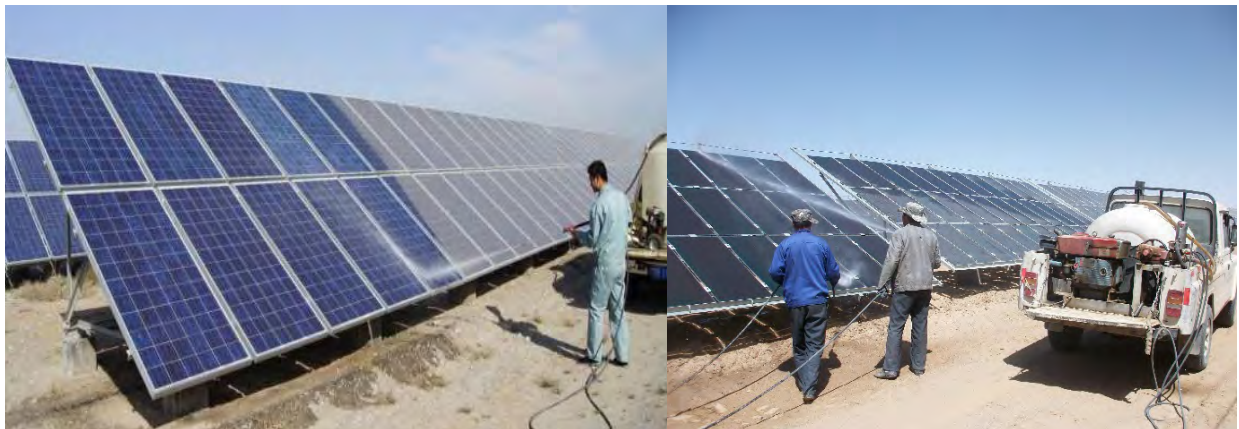
Fig. 1.1-13 Cleaning by flashing water
