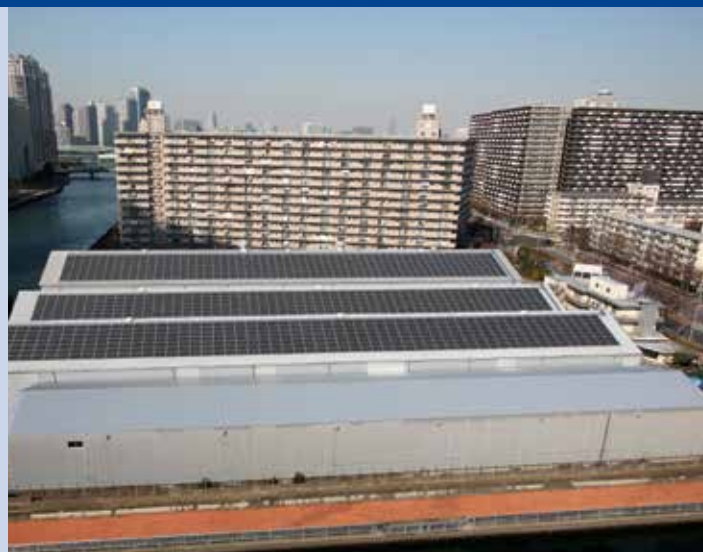
Fig. 1 - TETSUSO's Rental Storage Facilities (Koto Ward, Tokyo). Single-crystalline silicon PV module (by Mitsubishi Electric) 2,9 MW.
