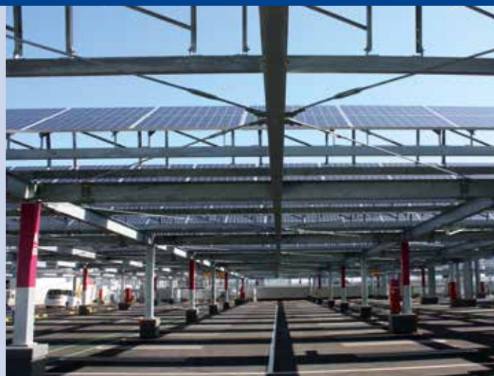
Fig. 2 - AEON Mall Makuhari New City (Mihama Ward, Chiba City, Chiba Prefecture). 242-W multicrystalline silicon PV module (Kyocera). Total: 1,75 MW, of which, parking area: 1 MW.
