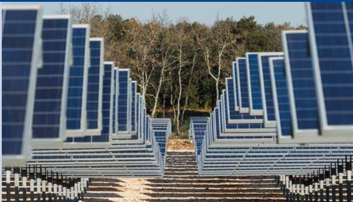
Fig. 2 – Photovoltaic power plant with horizontal single-axis tracker, 4,7 MW, Vallérargues (Gard Dpt), Urbasolar/Exosun (Photo: Christophe Ruiz).
