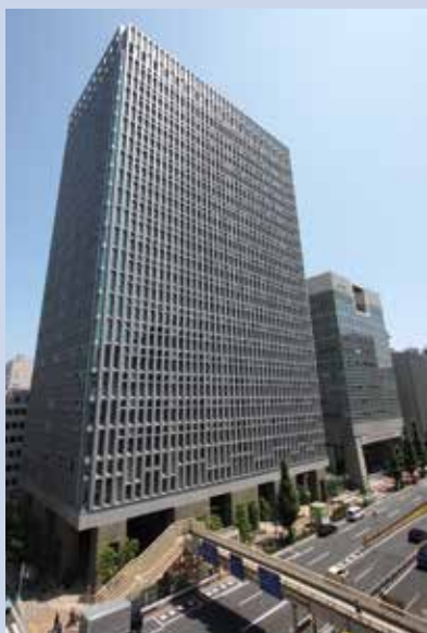
Fig. 3 - Shimizu Corporation headquarters building (Kyobashi, Chuo Ward, Tokyo). 150 kW Multicrystalline silicon PV module. 368 modules: 110 kW (by Sharp). Light-through thin-film silicon PV module 594 modules: 40 kW (by Sharp).
