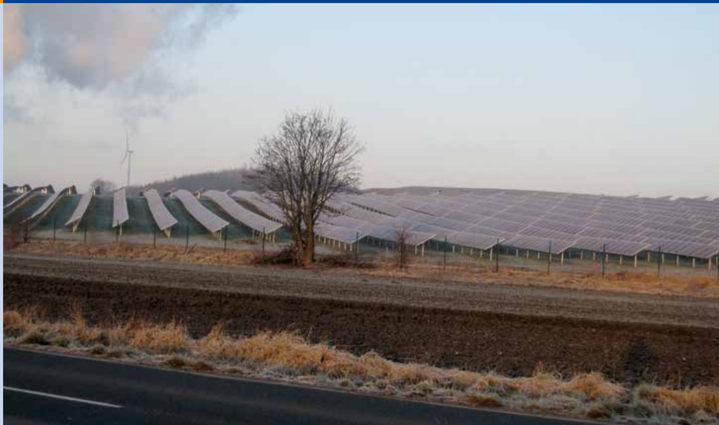
Fig. 2 - Ground mounted photovoltaic installation with 3,9 MW peak power on a former landfill site (Photo: Klaus Prume).
