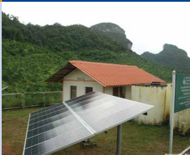
Fig. 2 - Solar PV Off-Grid System 2 kWp at Koh Phaluai School by Department of Alternative Energy Development and Efficiency, at Phaluai Island (Green Island), Suratthani, Thailand.
