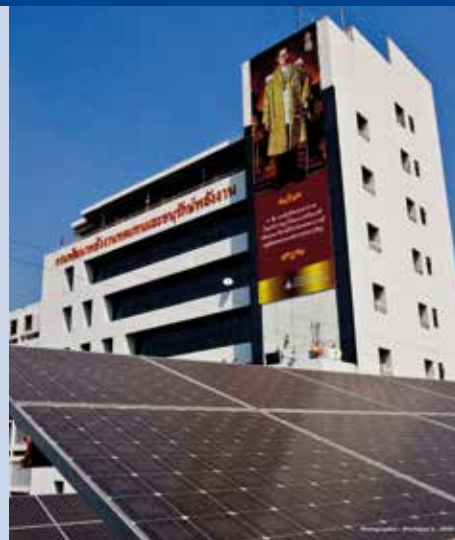
Fig. 3 - Solar PV Rooftop System 5 kWp at Department of Alternative Energy Development and Efficiency, Bangkok, Thailand.
