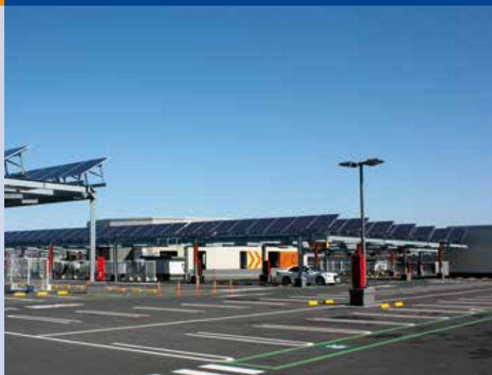
Fig. 2 - AEON Mall Makuhari New City (Mihama Ward, Chiba City, Chiba Prefecture). 242-W multicrystalline silicon PV module (Kyocera). Total: 1,75 MW, of which, parking area: 1 MW.
