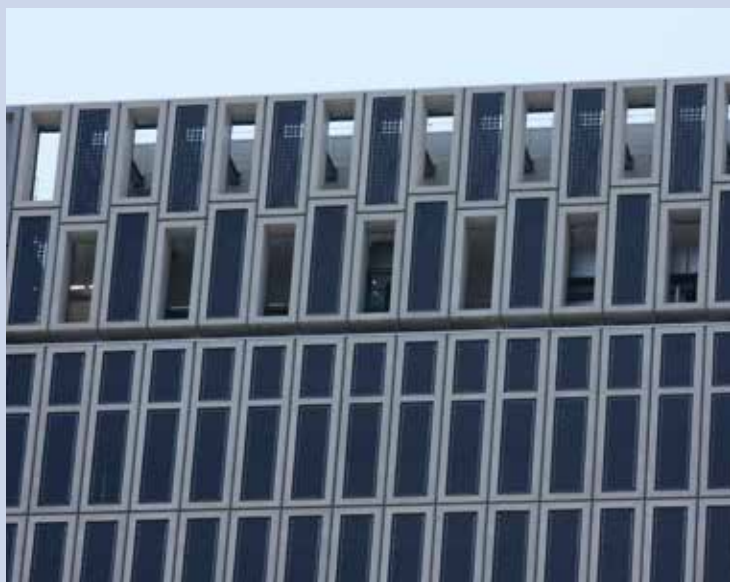
Fig. 3 - Shimizu Corporation headquarters building (Kyobashi, Chuo Ward, Tokyo). 150 kW Multicrystalline silicon PV module. 368 modules: 110 kW (by Sharp). Light-through thin-film silicon PV module 594 modules: 40 kW (by Sharp).
