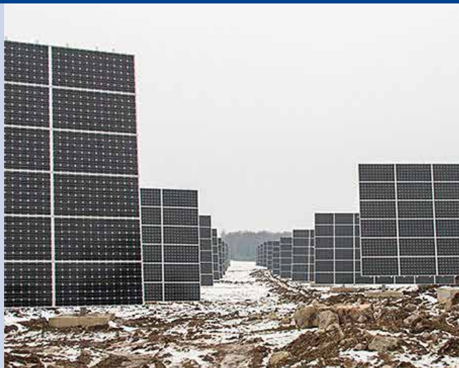
Fig. 1- The first Swedish MW-installation was constructed during 2013. Solar trackers are rather untypical for Sweden, and the site is participating in a monitoring study (Photo: Bengt Stridh, ABB/Mälardalens högskola).
