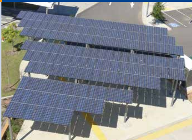
Fig. 2 – Shade shelter at bus and taxi rank, Townsville RSL Stadium. The 20 kW array (153 x Kyocera KD135W modules) is part of the Townsville Queensland Solar City Project (Photo: Ergon Energy).
