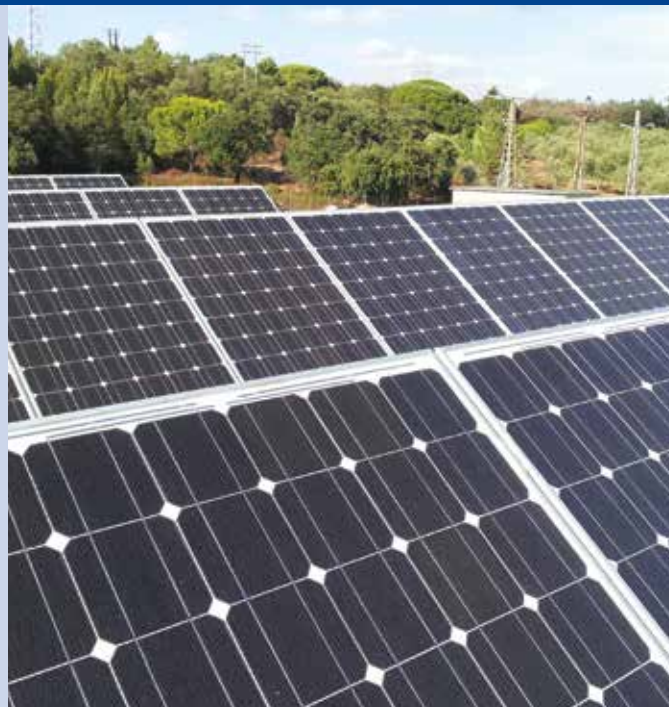
Fig. 1 - 5 kWp residential microgeneration project.
