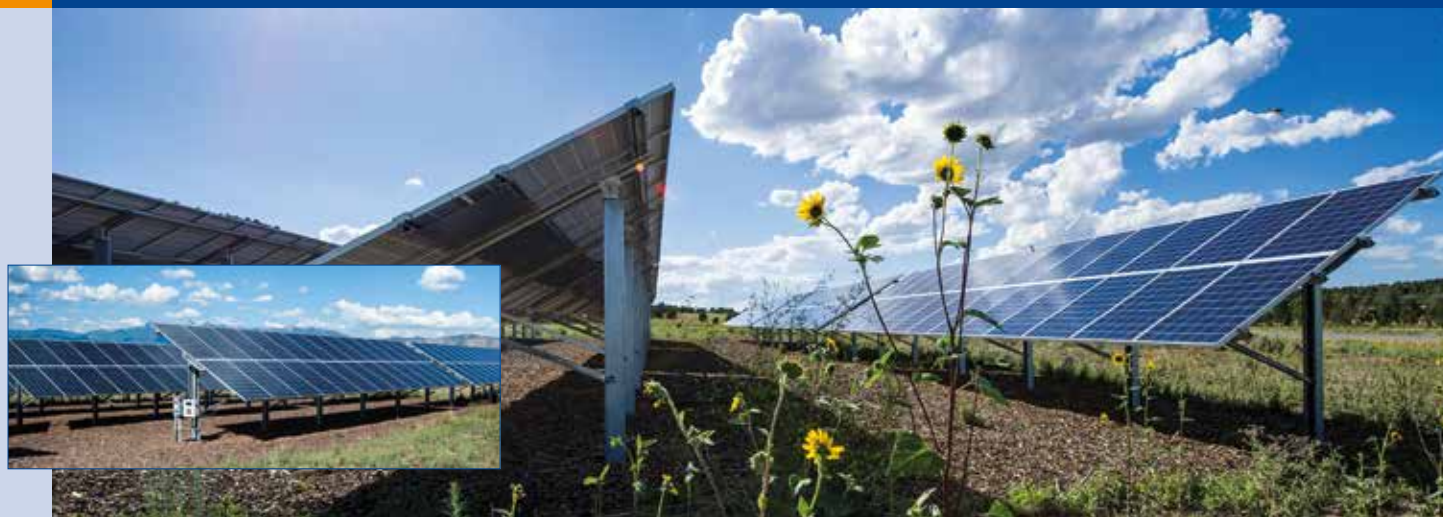
Fig. 3 - 67 kW (STC rating) photovoltaic array at the Mesa Verde Visitor and Research Center in Montezuma County, Colorado. The array consists of 286 Schott Poly 235 watt solar modules (13,8 % efficiency) wired in 22 series strings of 13 modules per string. Coupled with a micro-hydro system and solar water heating, the on-site renewable energy systems are capable of providing 95 % of the building energy requirements (Photo: Dennis Schroeder / NREL).
