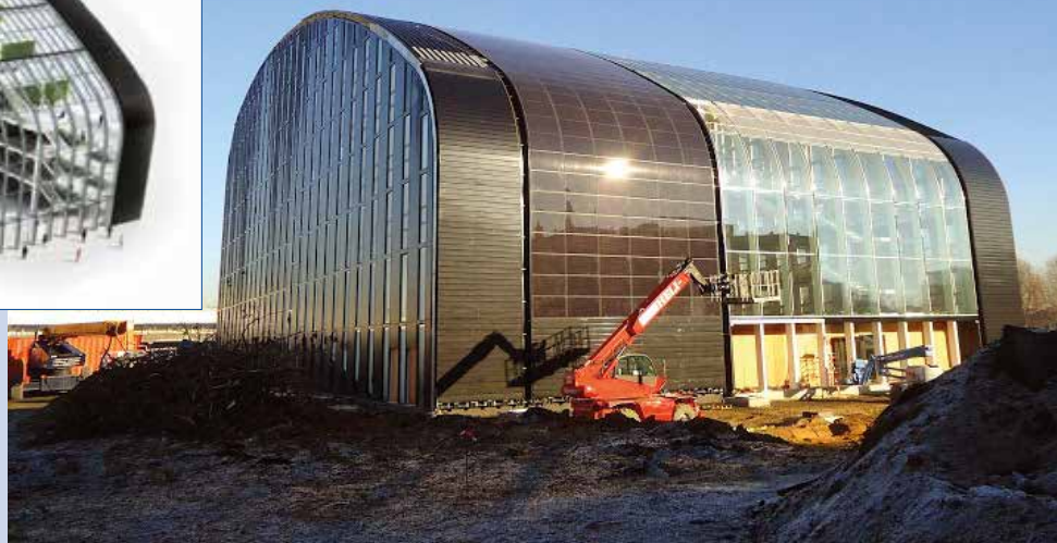
Fig. 1a & Fig. 1b – Bruxelles Environnement. The new Brussels Environment and Energy Administration Headquarters will be the largest passive office building in Europe and will include 700 m 2 of BIPV ISSOL modules (Photos: Copyright CEPEZED, ISSOL for Fig. 1a and ISSOL for Fig. 1b).
