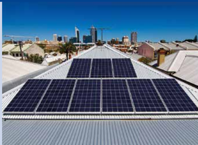
Fig. 3 – 2,1 kW residential array in Perth, using Hanwha Q.Cell's Q.Pro-G2 modules (Photo: Hanwha Q.Cells Australia).
