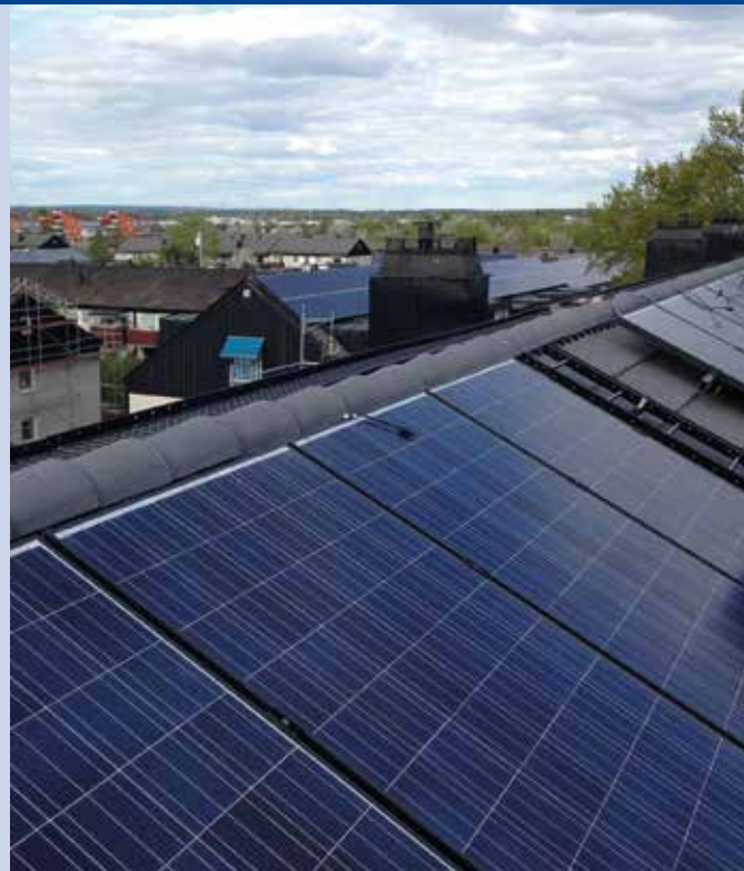
Fig. 4 - PV modules on several apartment buildings. 624 kW in total (Photo PPAM.se Sweden AB).
