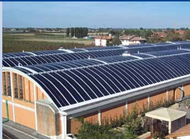
Fig. 2 – 123 kWp PV plant at Argenta (FE), using DERBISOLAR flexible modules (thin film on flexible support) (Photo: GSE, Gestore del Sistema Elettrico).
