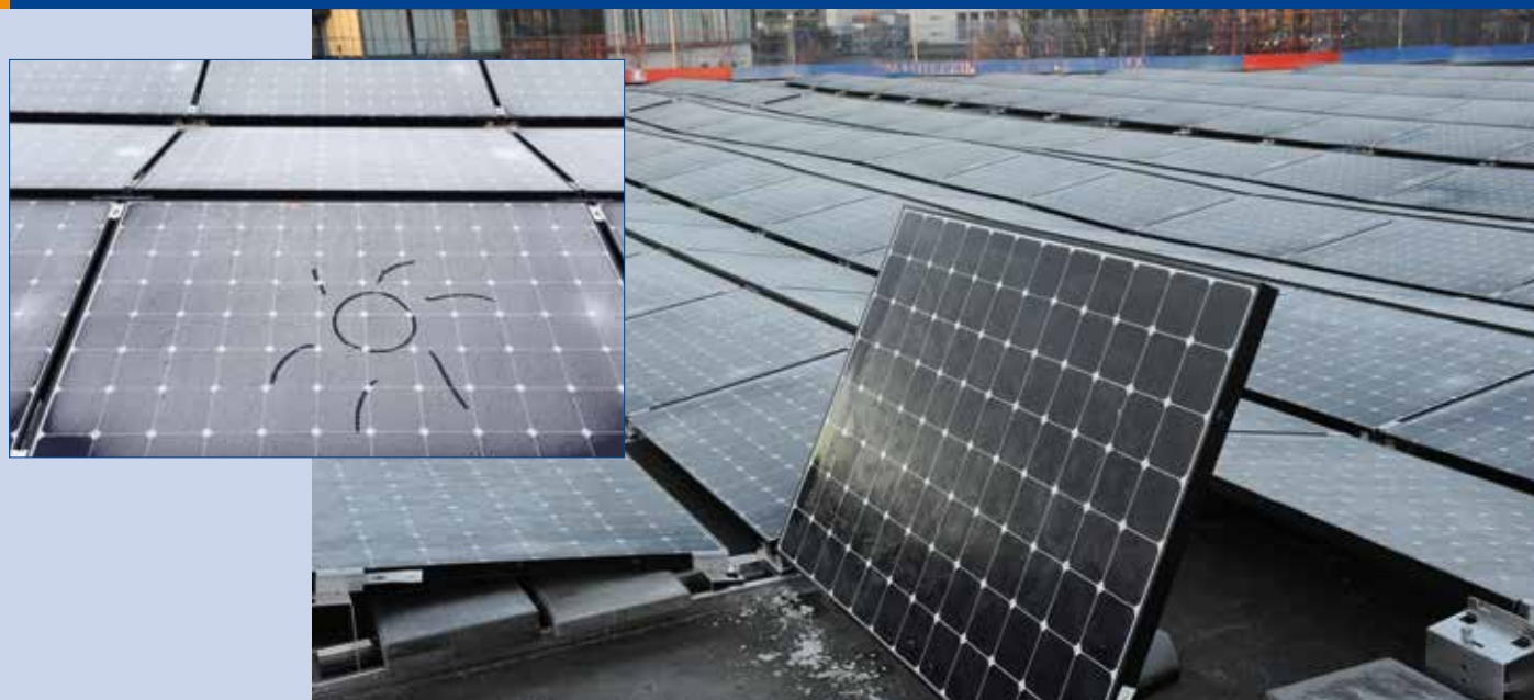
Fig. 4 - PV installation at Powerhouse Kjørbo, delivered by Direct Energy. The system has a capacity of 310 kWp (See also www.powerhouse.no ).
