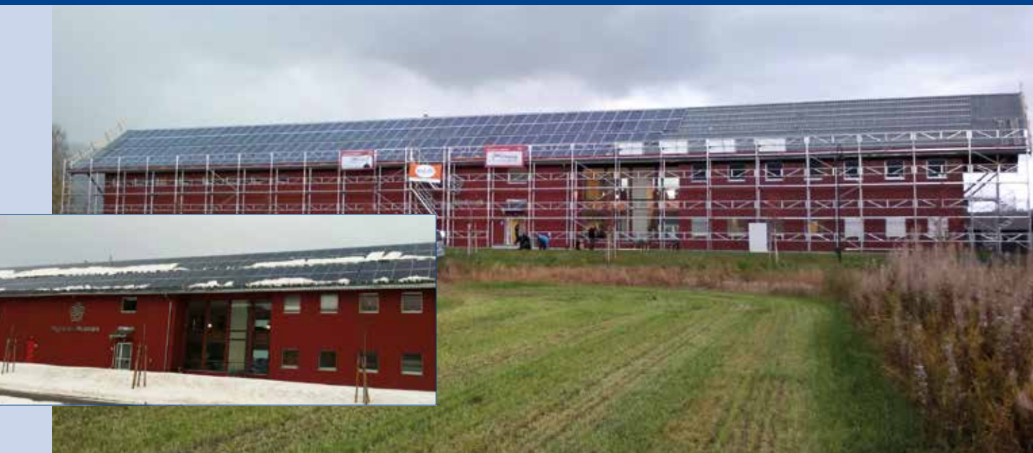
Fig. 1 and 2 - PV installation at Høgskolen i Hedmark, Avdeling Evenstad. 70 kWp system supplied by FusEn AS.
