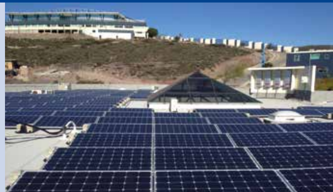
Fig. 2 - 75 kWp Grid Connected PV System at CICESE Ensenada Baja California, Mexico (Photo: Solartec).
