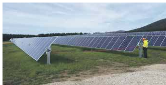
Fig. 2 - Commissioning of the 2,3 MW Mount Majura Solar Farm Oct 2016 developed by Solar Fields and Solar Choice. The Farm uses horizontal single axis trackers with two x 1MVA transformers to connect into the adjoining 11kV distribution lines.
