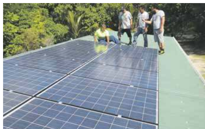
Fig. 9 – Fixing of a PV system in a Pacific Island (Photo: GSES).
