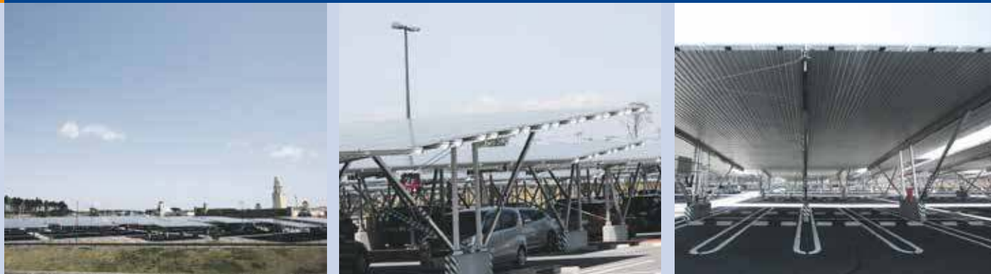
Fig. 3 - PV System for Parking Lot (AMI PREMIUM OUTLETS PV System Self-consuming All the Generated Power) (Ami-Machi, Inashiki Gun, Ibaraki Prefecture) 1,043 kW. Multicrystalline silicon PV module (by Kyocera, 265 W x ca. 4 000 modules).
