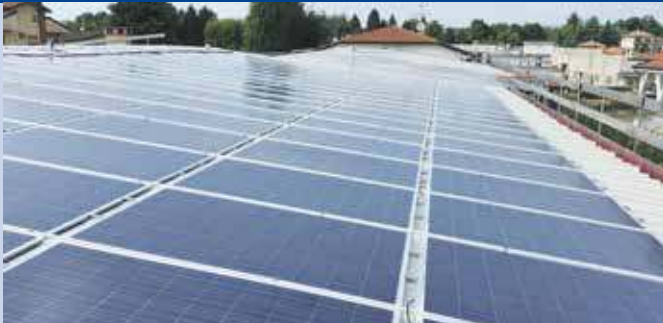
Fig. 1 - Roof integrated 106 kW PV plant at Arsago (VA), Polycrystalline modules (Photo: Solmonte www.solmonte.it ).
