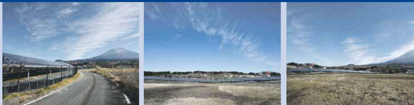
Fig. 1 - Fujigane PV Power Plant at the foot of Mt. Fuji (Fujikawaguchiko Town, Yamanashi Prefecture) 1,512 kW. Single crystalline silicon PV module (by Hansol Technics) (250 W x 6 048 modules).
