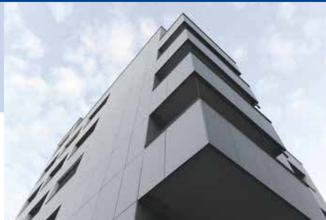
Fig. 2 - Hofwiesen- / Rothstrasse, Zurich, detailed view of the façade. Modules from PVP Photovoltaik GmbH, glass-glass module, based on monocrystalline cells (Photo: ©Viridén + Partner AG, Zürich).
