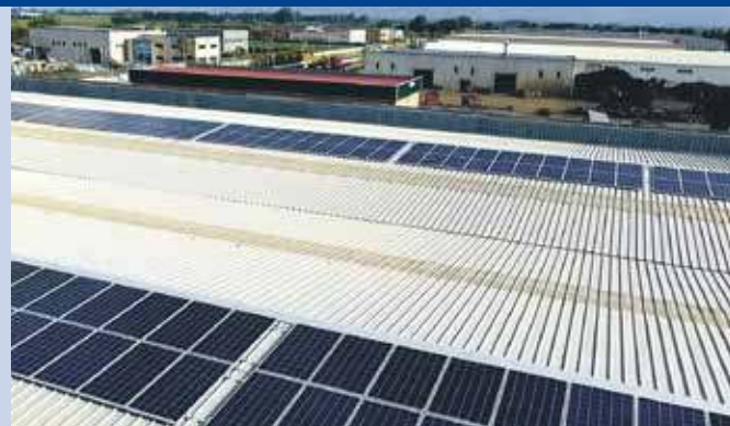
Fig. 4 – Roof integrated 60 kW PV plant at Lamezia Terme (CZ), 250 W Polycrystalline modules (Photo: SunCity Srl).
