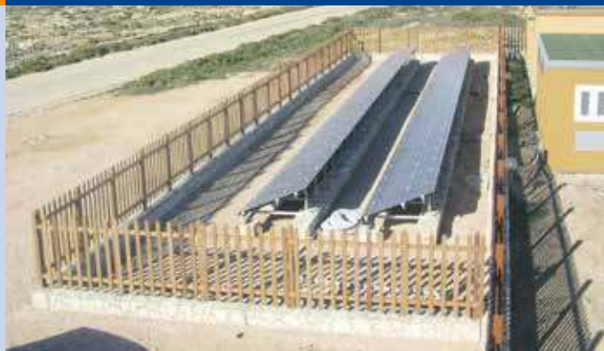
Fig. 3 – 14,4 kWp PV plant with 16 kWh Li-Ion Energy storage system, connected to the grid of Lampedusa island (Photo: ENEA, www.enea.it ).
