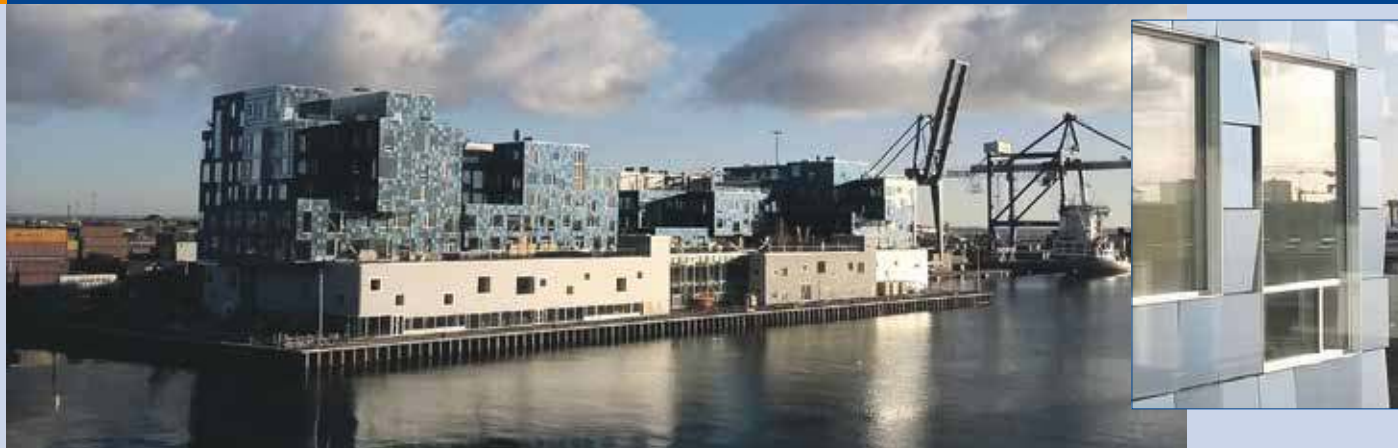
Fig 3 – Copenhagen International School is a new building located in Copenhagen's new district Nordhavn. The school building's facade will be covered in 12 000 solar individually angled panels, which will supply more than half of the school's annual electricity consumption. The PV will cover a total area of 6,048 square meters making it one of the largest building integrated solar PV plants in Denmark (photo: Anne Lilke Krag Hansen). Architect: C. F. Møller. Solar Cells: SolarLab.
