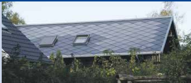
Fig. 1 - Roof integrated system developed and delivered by Gaia Solar and Steni.
