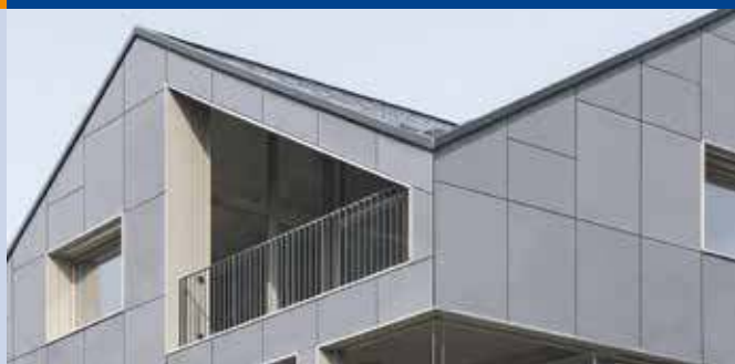
Fig. 3 - First energy self-sufficient apartment building in Switzerland is a project of the Umwelt Arena realised together with exhibition partners. The PV system on a multifamily building consists of an 80 kWp inroof system based on monocrystalline silicon roof system (512m 2 / MegaSlate II) and a 47 kWp micromorph silicon façade system (485 m 2 ). (Photo: ©Umwelt Arena Schweiz, Architekt René Schmid Architekten, Zurich; "Umwelt Arena" is the world's first permanent exhibition dealing with the subject of environmental sustainability.).
