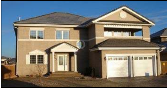
Non-rectangular roof surface - ETI Solar, Canada
