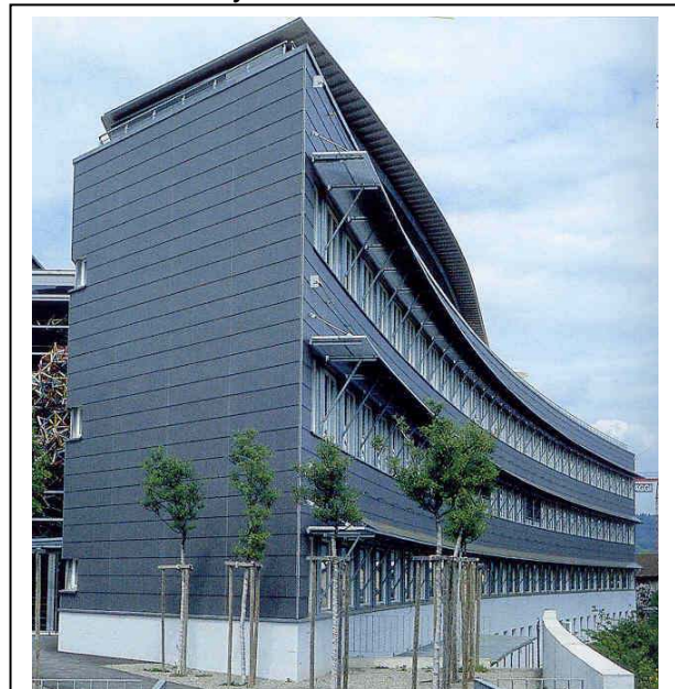
Window shade structure BIPV mounting technique
