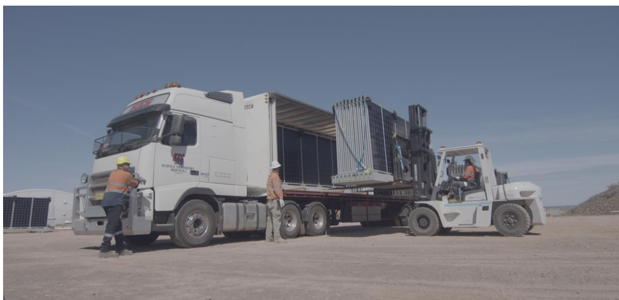
Figure 8. Innovative prefabricated mounting array lowers the cost of deployment in remote regions. Images courtesy of 5B Pty Ltd.
