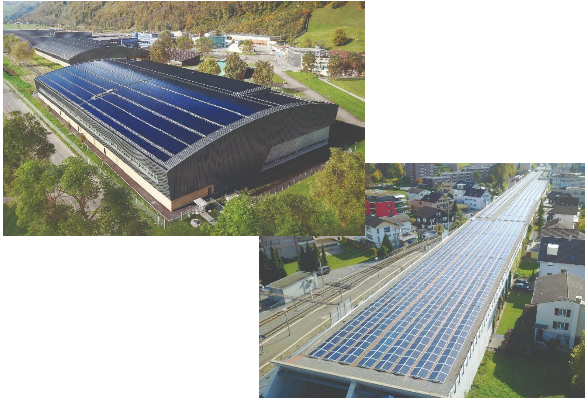
Figure 1: 1.05MW PV installation at Pilatus Aircraft Company, Stans (left) and 840 kW on top of a highway tunnel in Stansstad (right). © Solaragentur
