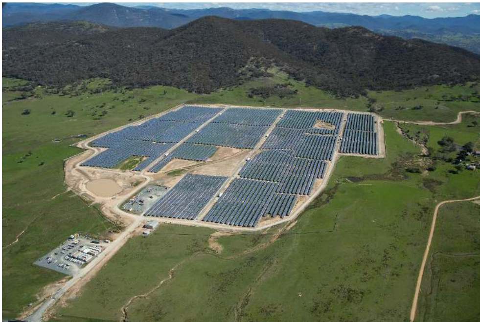
Figure 8: Royalla Solar Farm. (FRV Services Aust Pty Ltd, 2015)
