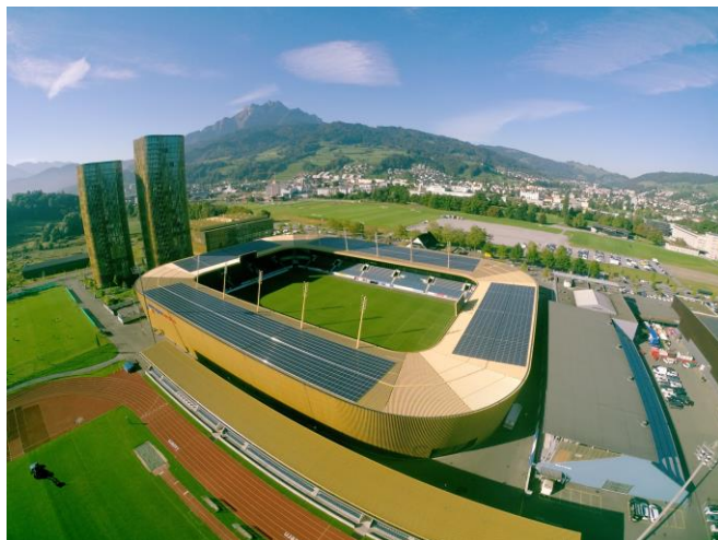
Swissporarena, Lucerne 1,1MWp Engineering, Installation & Photo: BE NETZ AG, Lucerne
