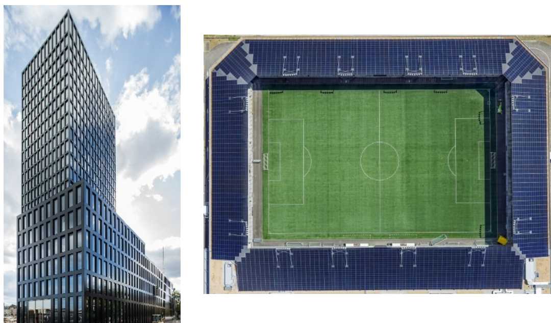
Figure 1: 440 kW PV installation at Grosspeter Tower, Basel (left) and 1.4 MW on a Football Stadium in Schaffhouse (right). © Solaragentur
