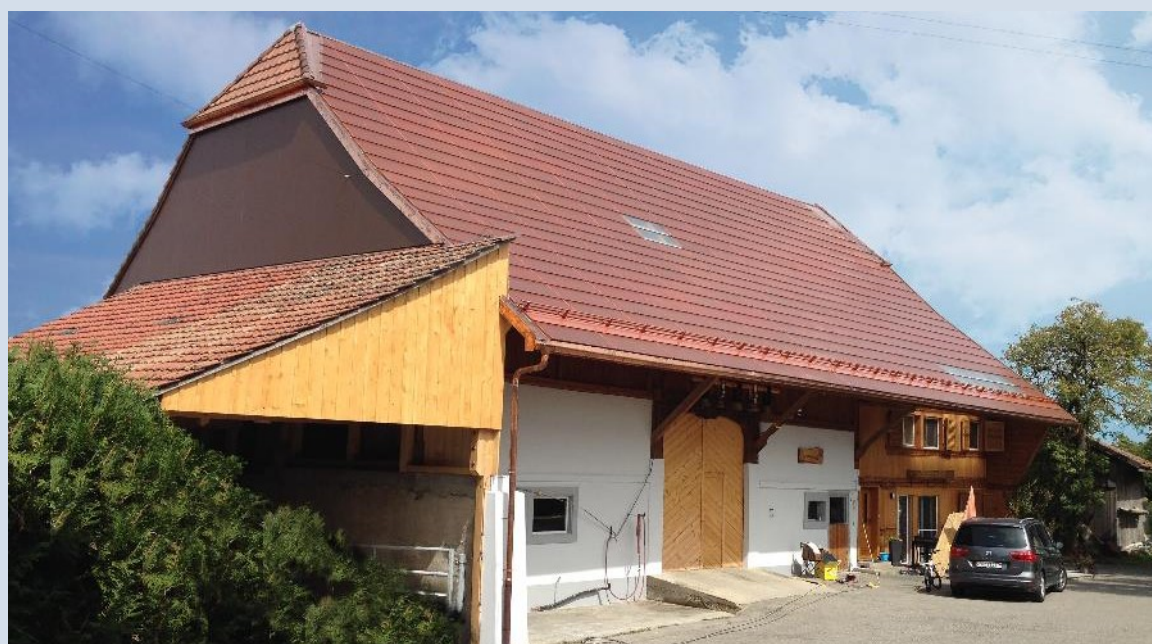
Terracotta-red solar panels installed on the roof of a protected farmhouse in Ecuwillens Foto: © CSEM/Issol, Neuchâtel
