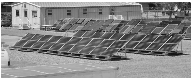
Figure 34: The photovoltaic array used in the present work had a total capacity of 10.8 kW. The array had four strings that each had 10 modules. The strings were combined prior to entering the inverter, where each of the string's current, voltage, and power were monitored
