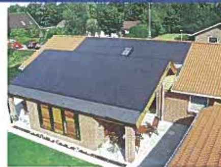
Fig. 1: House from the Sol-300 project with 3 kWp roofintegrated BP-Solarex thinfilm laminates.
