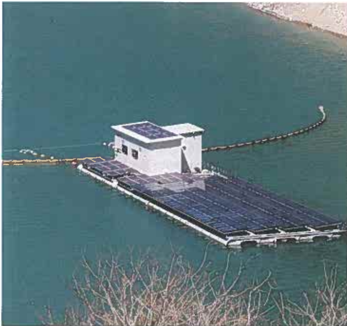
Fig. 3 and 4: 28 kW stand-alone PV system (25 kW mc-Si and 3 kW a-Si) on the moored barge; PV power is mainly used for water purity control equipment, and the surplus PV power is supplied as emergency power source at the parking lot through an underwater cable.
