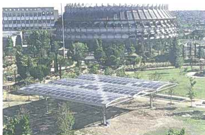
Fig. 1: "40 kW grid-connected PV plant in La Moncloa, Madrid"
