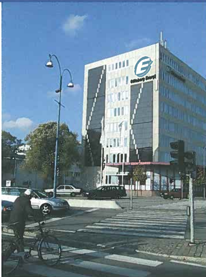
Grid connected 7,3 kWp wall mounted thin film system, Gothenburg Energy Ltd. Office building in Gothenburg, Sweden (Photo: Gothenburg Energy Ltd., 2000)
