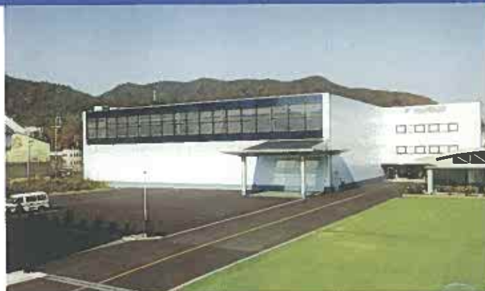
Fig 1: PV system installed on southward semi-transparent wall (19.4 kW, 229 sq. m) and canopy (1.7 kW, 56 sq. m) of plant
