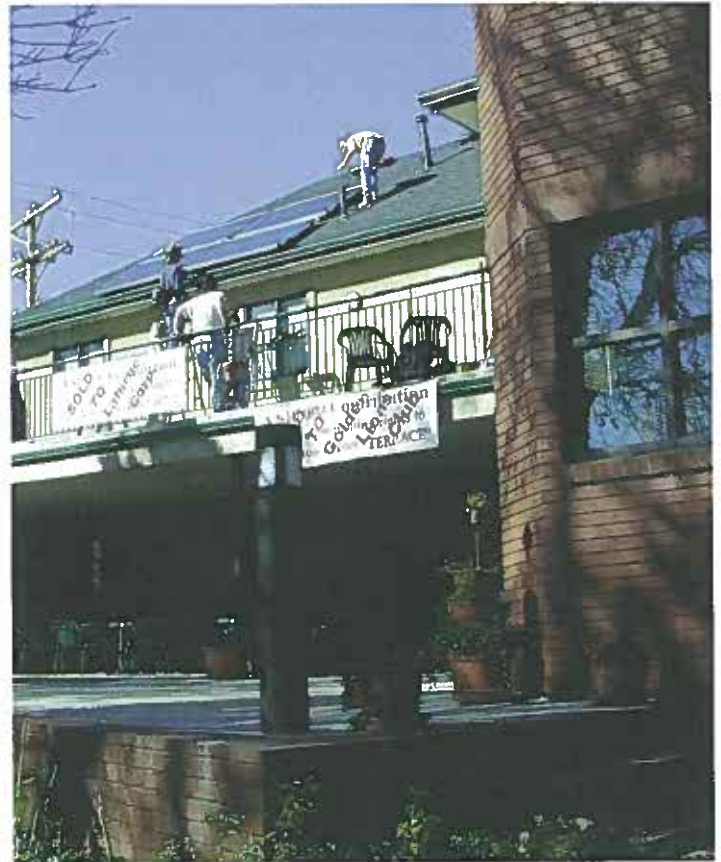
The Visitors Center at Golden, CO hosts four Sunline 300 AC PV Modules. Each AC module uses an Ascension Technology, Inc. micro-inverter attached to an ASE America large area PV module and is rated at 250 Wac. Photo courtesy of Holly Thomas (NREL).
