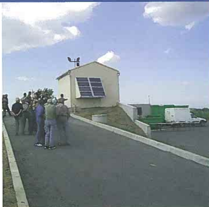
Figure 1 – A Municipal separate collection centre is equipped with a stand alone PV system (Face fund). photo APEX.
