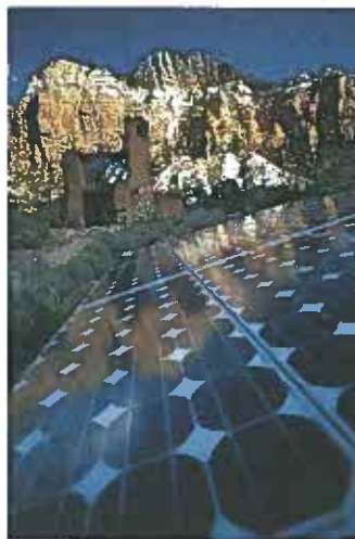
PV Powers This Monastery of Christ in the Desert Where 15 Computers Provide Web Site Designs Worldwide. (Photo Courtesy of Siemens Solar Industries)
