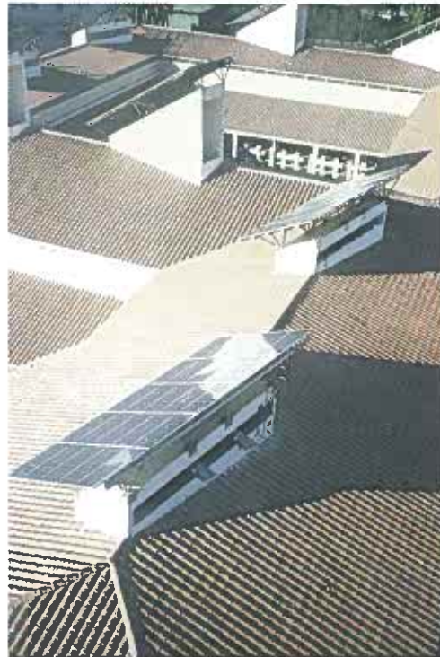
Fig. 2: "11.28 kW grid-connected PV plant in Cádiz
