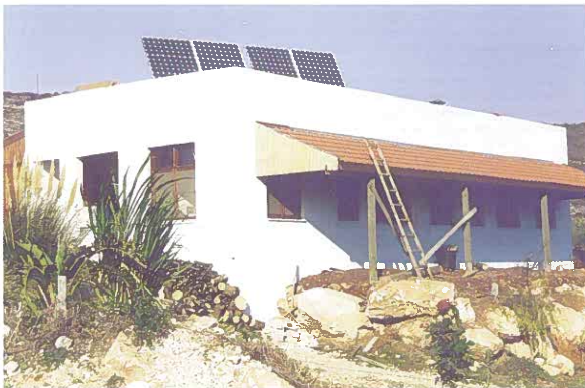
Fig. 3: 1.05 kW array on a remote home in Galilee (Interdan).
