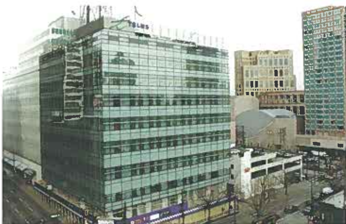
Figure 3. The renovation of this 52-year-old building incorporated a new façade that provides waste heat recovery and the 2.5kW PV panels now power DC fans that ventilate this air space. (Photo: BCIT)
