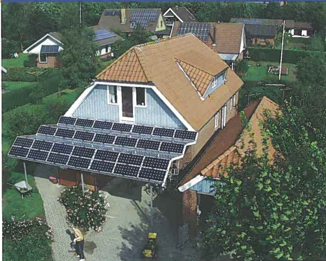
Fig. 2: Houses from the Sol-300 project. In front 2,4 kWp BP-Solarex laminates integrated in a pergola.
