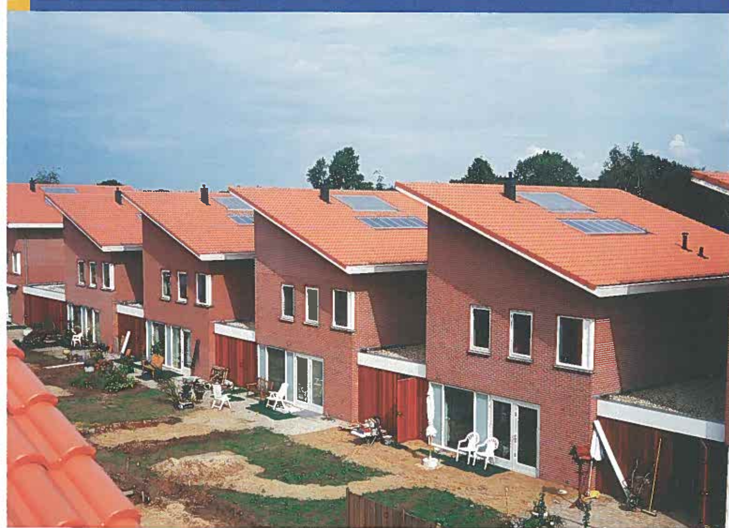
Fig. 3: In the Nijrees project in Almelo three different PV integration systems are applied on private houses, by three developer/architect combinations. Goal of the project is to compare the systems on esthetics, price and building logistics. Systems used are the Shell Solar BOAL, the RBB PV 700 and the Econergy/Unilin integration system (Copyright Novem - Hans Pattist)
