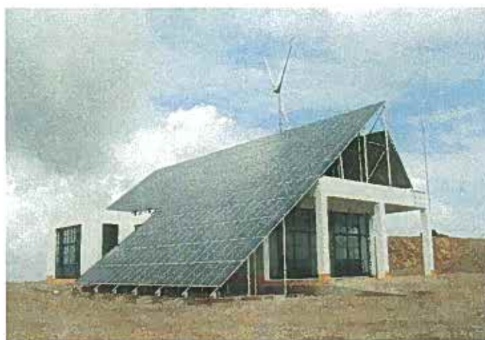
Fig. 4: Stand-alone hybrid PV/wind/diesel system (EDP, Ourique)
