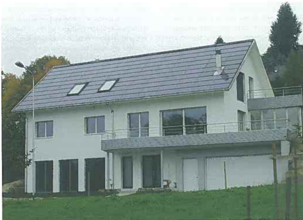
PV roof integration in a low energy house with SOLRIF (Solar Roof Integration Frame), 12 kWp, Enecolo
