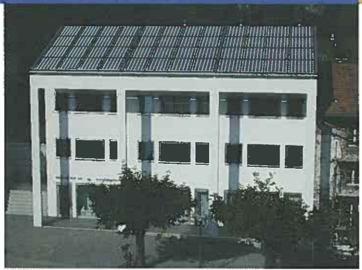
PV roofs in the old town of Interlaken, semi-transparent modules, 6 kWp, Fabrisolar
