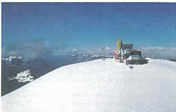
Figure 1. This PV-hybrid telecommunication station owned by NorthwTel is being studied as part of the Canadian PV-hybrid R&D program at CANMET-EDRL.
