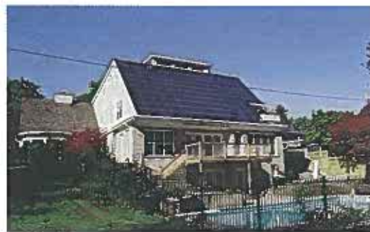
Figure 2. ARISE HOME Research and demonstration covering the surface of this rooftop with both solar thermal and 5kW of PV panels. The objective is to develop a comprehensive solar energy system that will provide much of the electricity and heating needs for new homes. (Photo: ARISE Technologies Corp.)
