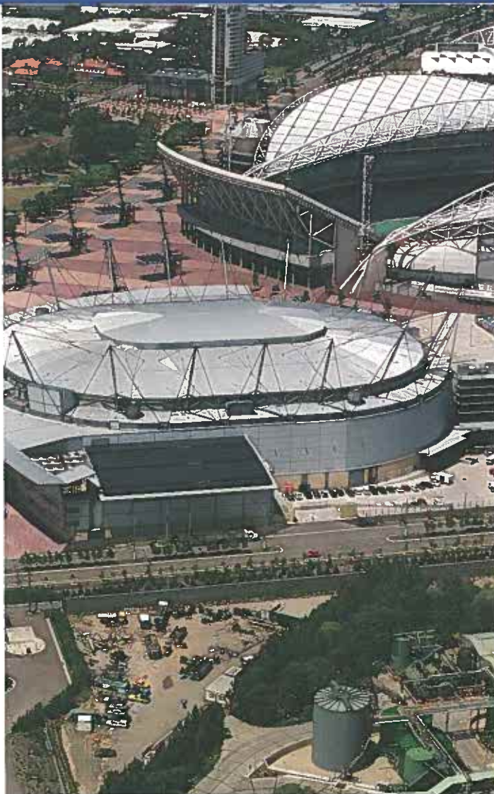
"The 70 kWp PV power system on the roof of the Sydney Superdome provides Green Power for energy retailer EnergyAustralia's 'Pure Energy' scheme (photo courtesy of EnergyAustralia and Canon Australia)"
