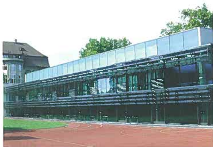
PV façade on a school building in Zurich, insulating glass modules, 11,5 kWp, TNC (façade view)
