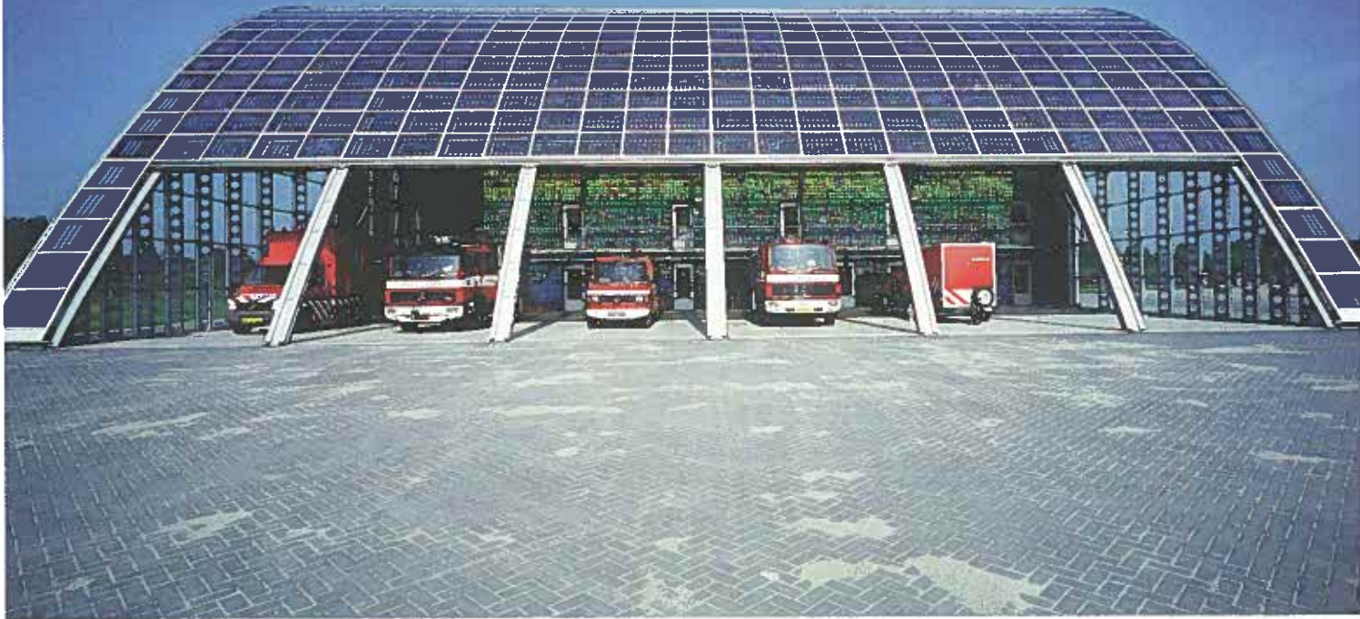
Fig. 2: The fire station of Houten was designed by the Belgian architect Philippe Samyn to combine esthetics and functionality. The semi-transparent panels provide an interesting light pattern in the black and with interior, that is livened up by the bright red fire trucks and colourful childrens' paintings on the interior wall (Copyright Novem - Hans Pattist)
