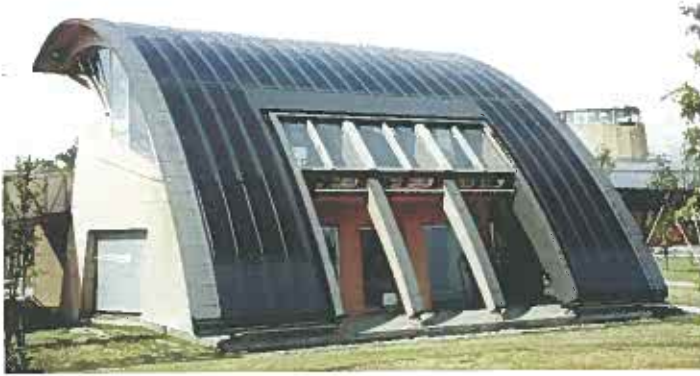
Fig. 2: Arch roofing integrated PV system (7.8 kW) to children's science museum "Fort of Sun and Wind"
