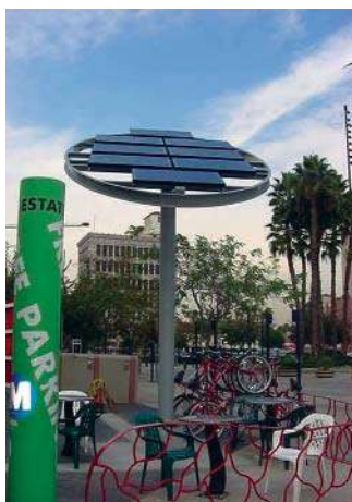
Fig. 2 - Long Beach Bike Station Includes 2 kW PV. Photo by Monica Grau and courtesy of Los Angeles Department of Water and Power.
