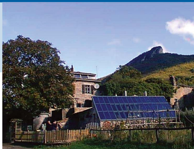
Fig.2 - Rural electrification, Farm in Ombleze (Drôme), 1,8 kW. (photo Transénergie)
