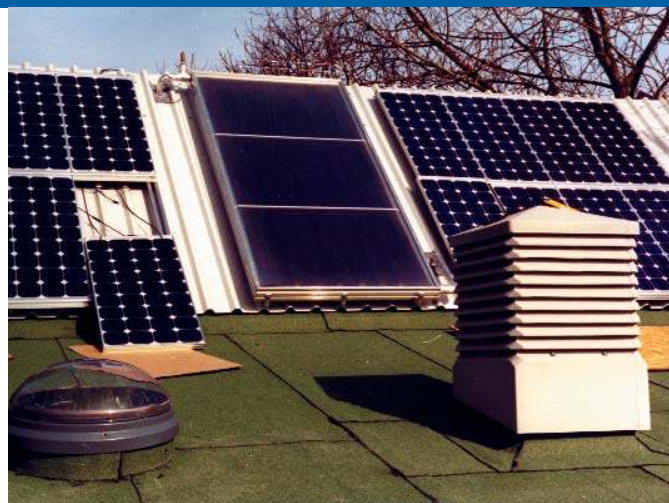
Fig. 1 – Greenfields- A solar collector, natural ventilation flue and light pipe are also saving fossil fuels on this roof.
