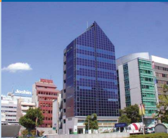
Fig.3 - 60 kW curtain wall type PV system and 16.7 kW skylight PV system.
