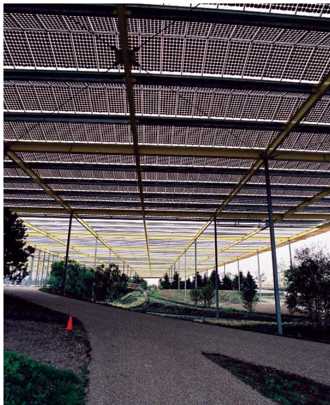
Fig.3 - Floriade At the Floriade 2002 exhibition NUON built the largest roof integrated PV system of the world. 28 000 m 2 of transparent PV panels yield 2,3 MWp of installed PV power. (Copyright NUON)
