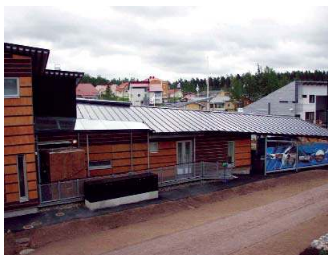
Fig. 1 - Villa 2000, building integrated PV elements (2.4 kWp) by Rautaruukki Oy.
