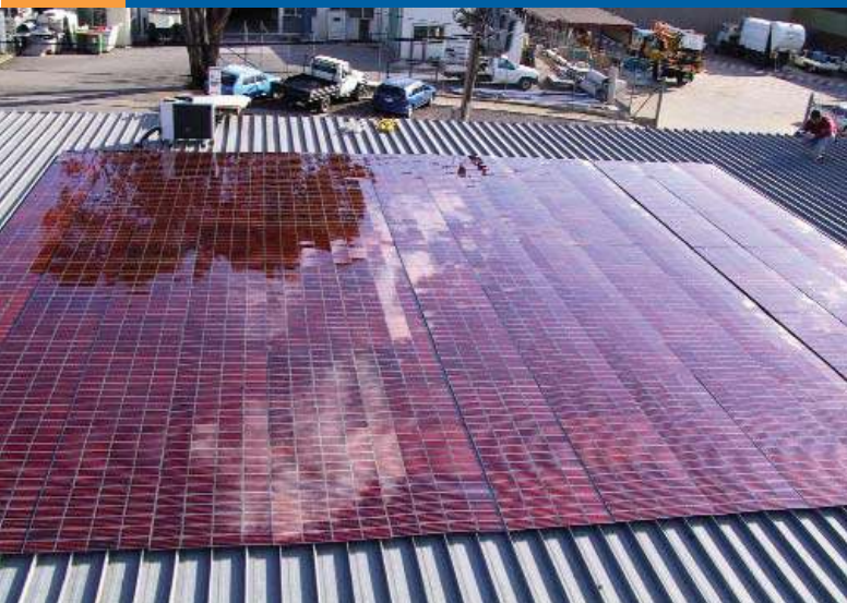
Fig. 2 - The first 100 square metres of solar panels manufactured by Sustainable Technologies International at the world's first Dye Sensitized Solar Cell manufacturing facility. (photo courtesy of Sustainable Technologies International)
