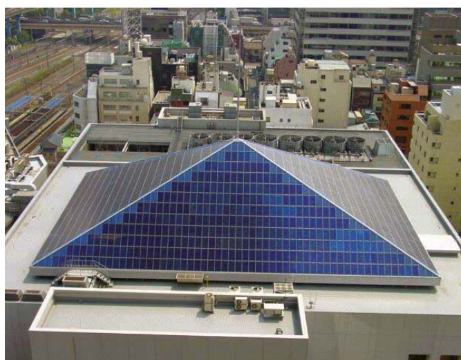
Fig. 2 - 84.7 kW Grid-connected PV system using ribbon type multi-crystalline silicon
