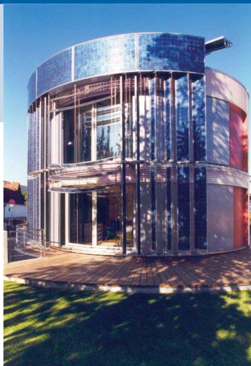
Fig. 2 - Futuristic "Gemini Sun House" at the Styrian state exhibition "Energy" in Weiz, 3 different PV-systems, partly with tracking, 6.7 kWp, AEE.
