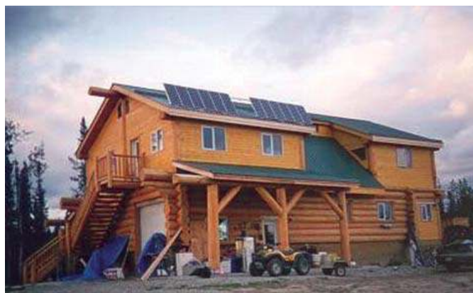
Fig. 2 - This residence is powered by a PV/Genset hybrid system in Whitehorse, Yukon, and is being monitored as part of the Canadian PV-Hybrid R&D Program at CANMET-EDRL.
