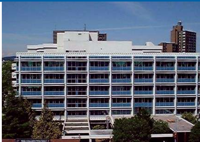
Fig. 1 - The renovation of the Richard Blanchard building for the Ministry of Health in Victoria, British Columbia incorporated Building-Integrated PV elements to replace the opaque spandrel panels on a section of the façade. This 2.6kW demonstration was championed by the BC Green Building Program and the BC Building Corporation. (photo Gordon Howell)
