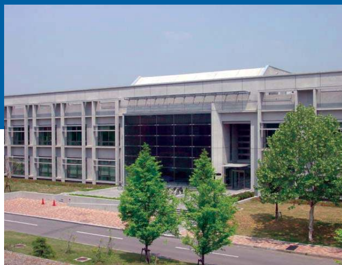
Fig. 1 - Building material integrated PV system (9.5 kW) and light transparent type PV cell (1.9 kW)
