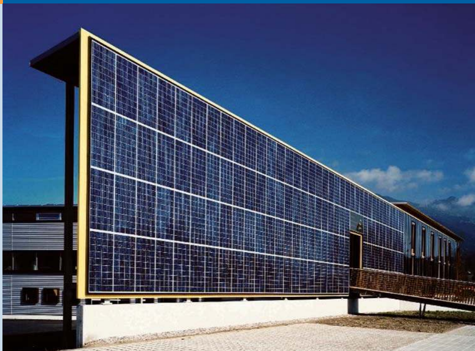
Fig. 3 - Energypark West in Satteins, 220 m 2 energy-facade with PV & thermal modules, 17.16 kWp, stromaufwaerts GmbH.
