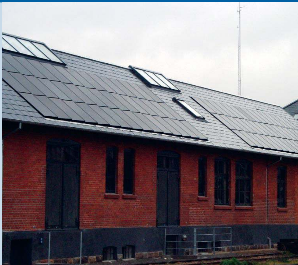
Fig.4 - 3,9 kWp system (thin film) from the Danish BIPV programme. (old warehouse)
