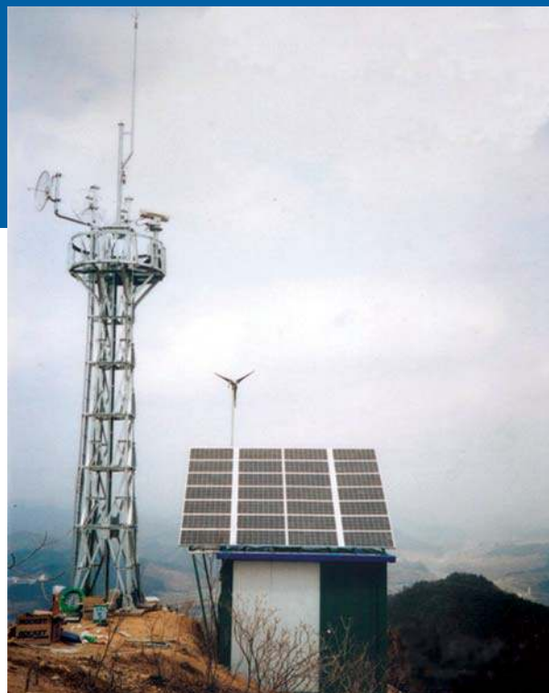
1.5 kWp PV system for forest fire observation towers CCTV.
