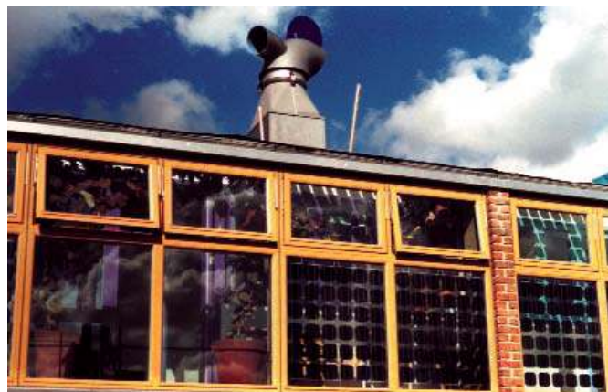
Fig. 3 - PV within double glazing on the zero emissions housing project, BedZed.
