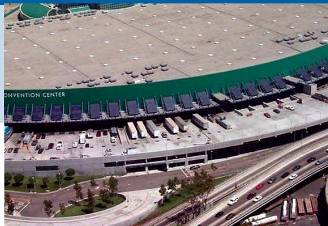
Fig. 3 - Los Angeles Convention Center Canopy completed September 2001 produces 250 kW ac power. Photo by Monica Estrata and courtesy of Los Angeles Department of Water and Power.
