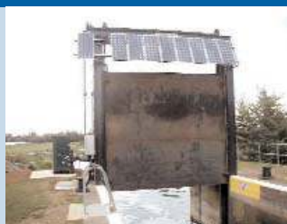
Titchmarsh Lock: PV powered lock gate, UK. (source: IT Power)
