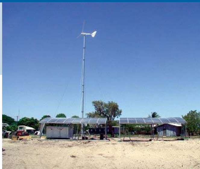
Fig. 4 - An 18 kW off-grid combined PV/wind power system installed at Inkerman Station on Cape York, Queensland. The system includes a 25 kW three phase inverter, a 1 400 Ah 120V DC battery bank and the existing 40 kVA generator has been incorporated into the system. The Inkerman RAPS system is a recipient of a rebate under the joint Australian and Queensland Governments' Working Property Rebate Scheme. (photo courtesy of Ergon Energy)
