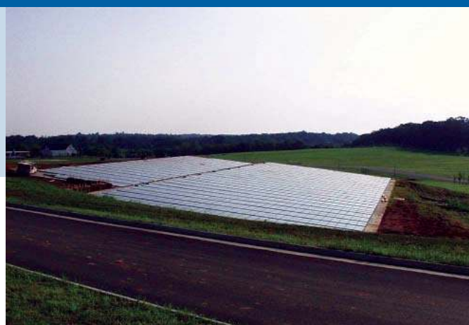
Fig.1 - Barns at Franklin Park 80 kW Millennia PV array and part of an innovative hybrid power system. Photo Courtesy of BP Solar.
