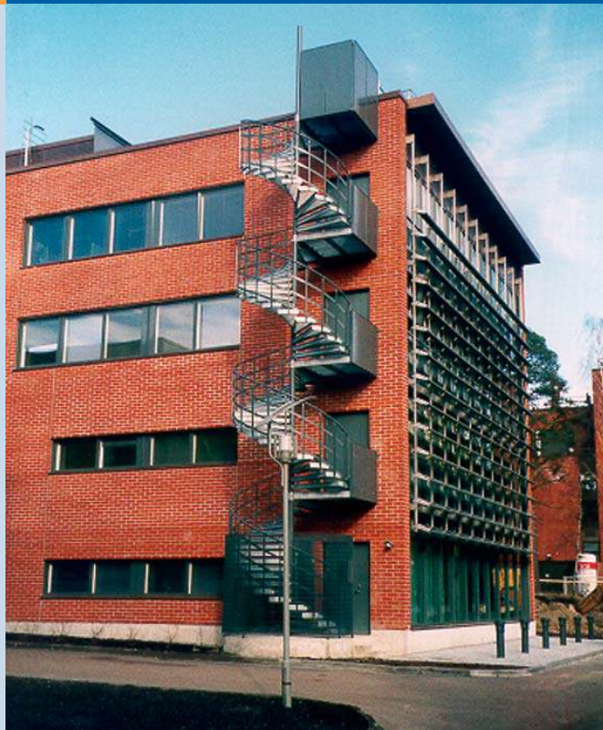
Fig. 2 - Helsinki University of Technology, Department of Electrical Engineering. Solar panels mounted on shading elements forming a total of 60 m 2 panel area and 7 kWp peak power.
