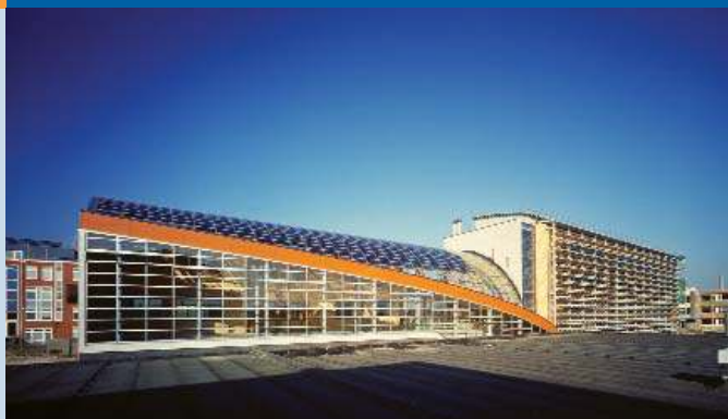
Fig. 2 - ECN facade and glass roof ECN combined different techniques at their offices in Petten, partly new and partly renovation. The facade, staircase and the roof designed by Tjerk Reijenga (BEAR architects) offer space to approximately 70 kWp of PV. (Copyright Novem/Hans Pattist)
