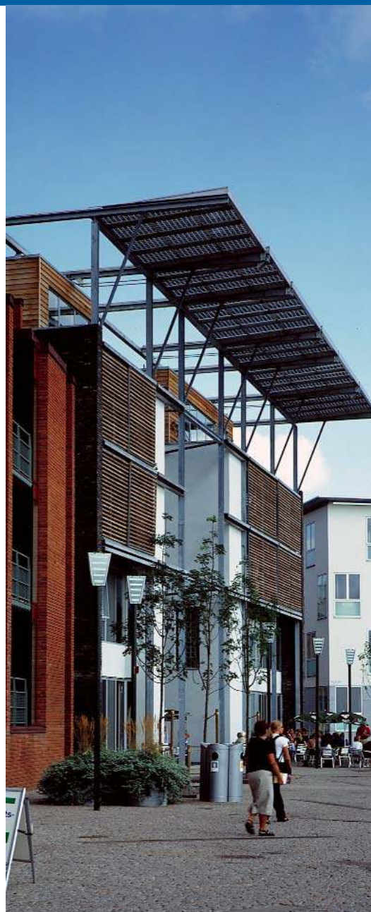
Grid connected 10,9 kWp semi transparent PV-system. Apartment building in "Bo01 City of Tomorrow - a European housing exhibition," Malmö, Sweden. (Photo Carl Michael Johannesson, 2001)
