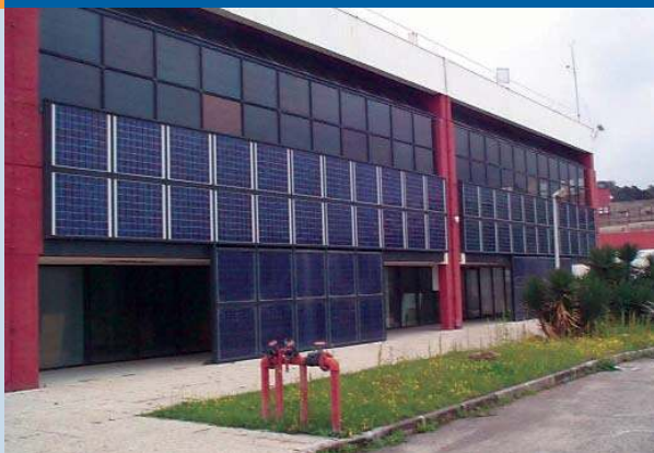
PV facade on ENEA-Portici laboratories
