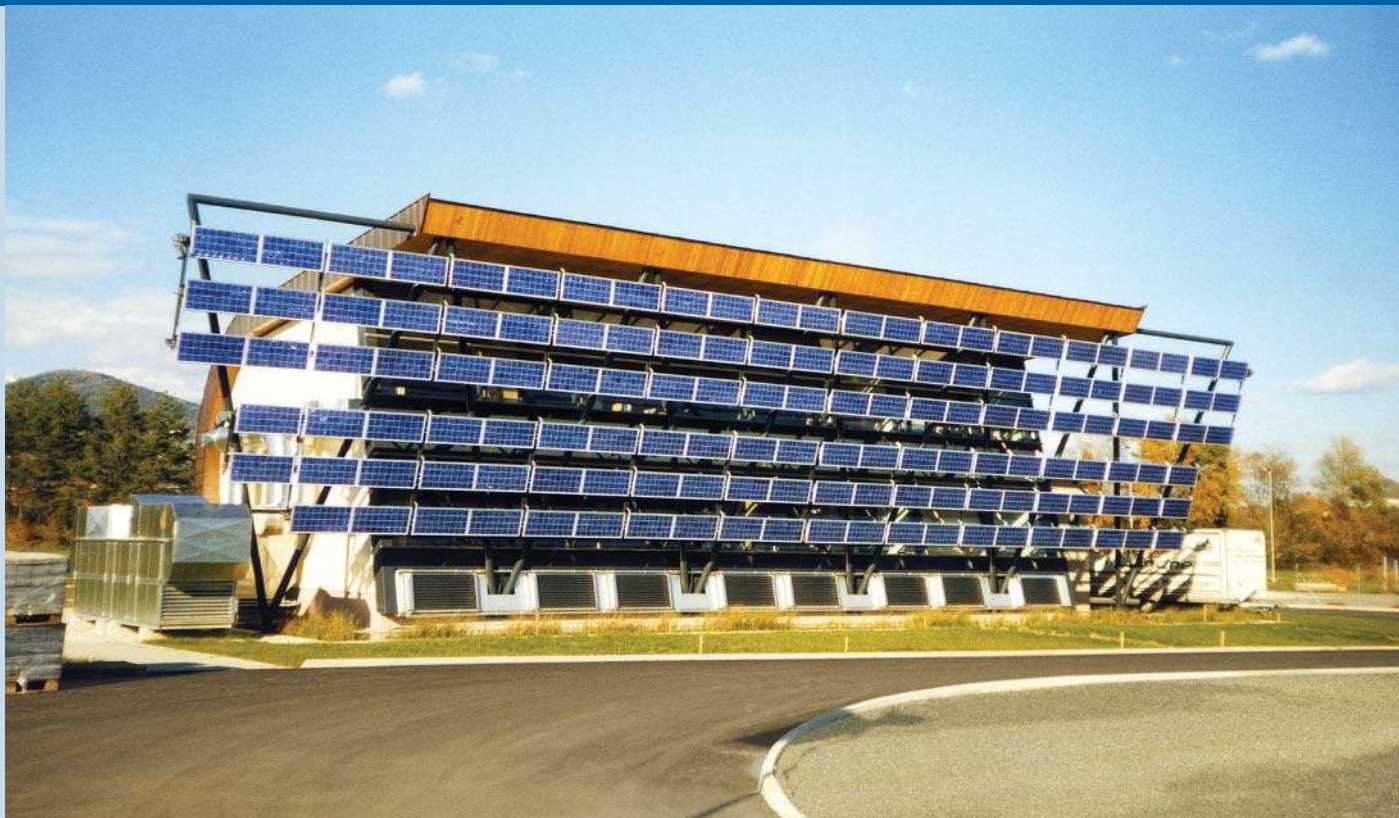
Fig. 1 - Hartberg Ecopark, Research Center, PV-modules as a shading element, Stadtwerke Hartberg. (municipal utility)
