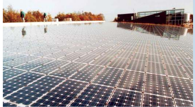
Fig. 1 - Annen zonnecentrale The PV installation of Essent in Annen, 180 kWp is the first utilitieside PV generator in The Netherlands. (Copyright Essent)
