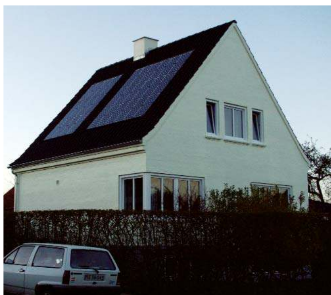
Fig. 2 - 2,55 kWp system from the Danish BIPV programme.
