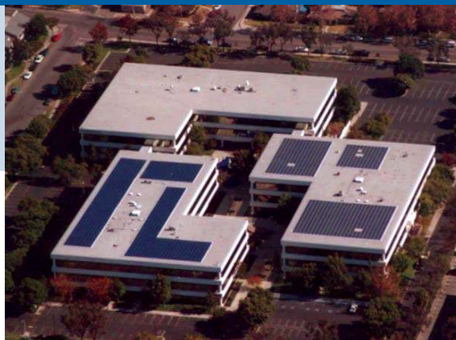
Fig. 4 - Fountain Valley City Center uses two PowerGuard (110kW) PV systems. Photo Courtesy of PowerLight.
