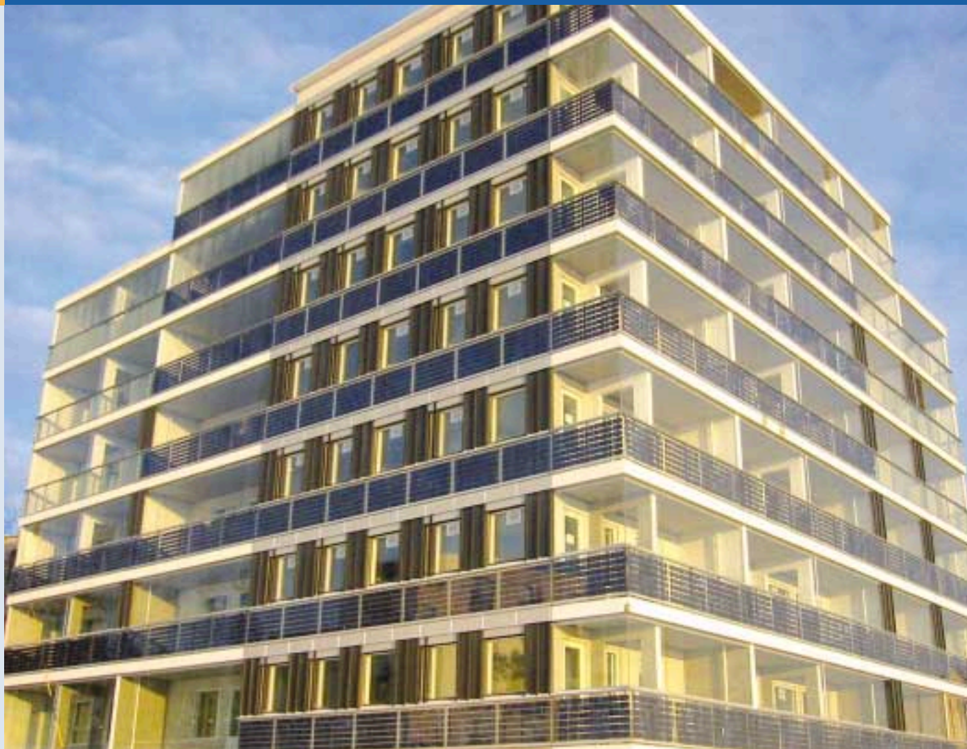
Fig. 1 - Ekoviikki area is a unique ecological housing area in the capital Helsinki. Special emphasis has been put on several ecological issues such as energy. By the end of 2002, the largest building integrated PV system in Finland in a dwelling house (24 kWp) was installed. The modules are partly see-through type and they form part of the balcony glassing on south and west sides of the building. During summer time, the excess electricity is fed into the grid whereas in winter months the local energy company returns it back. Approximately one fourth of the electricity consumption over the year is generated by PV. (Photo Solpros Ay)
