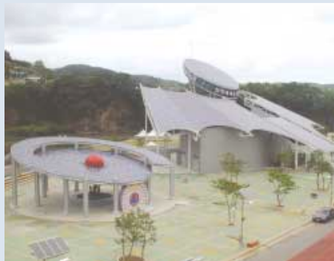
Fig. 3 - 107 kWp BIPV Systems at Cavity Expo Pavilion.
