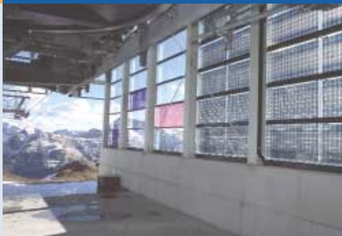
Fig. 2 - Cable-car station at the Kriegerhorn, Lech am Arlberg, 2 100 m above sea level, semitransparent modules 9,5 kWp, ATB.
