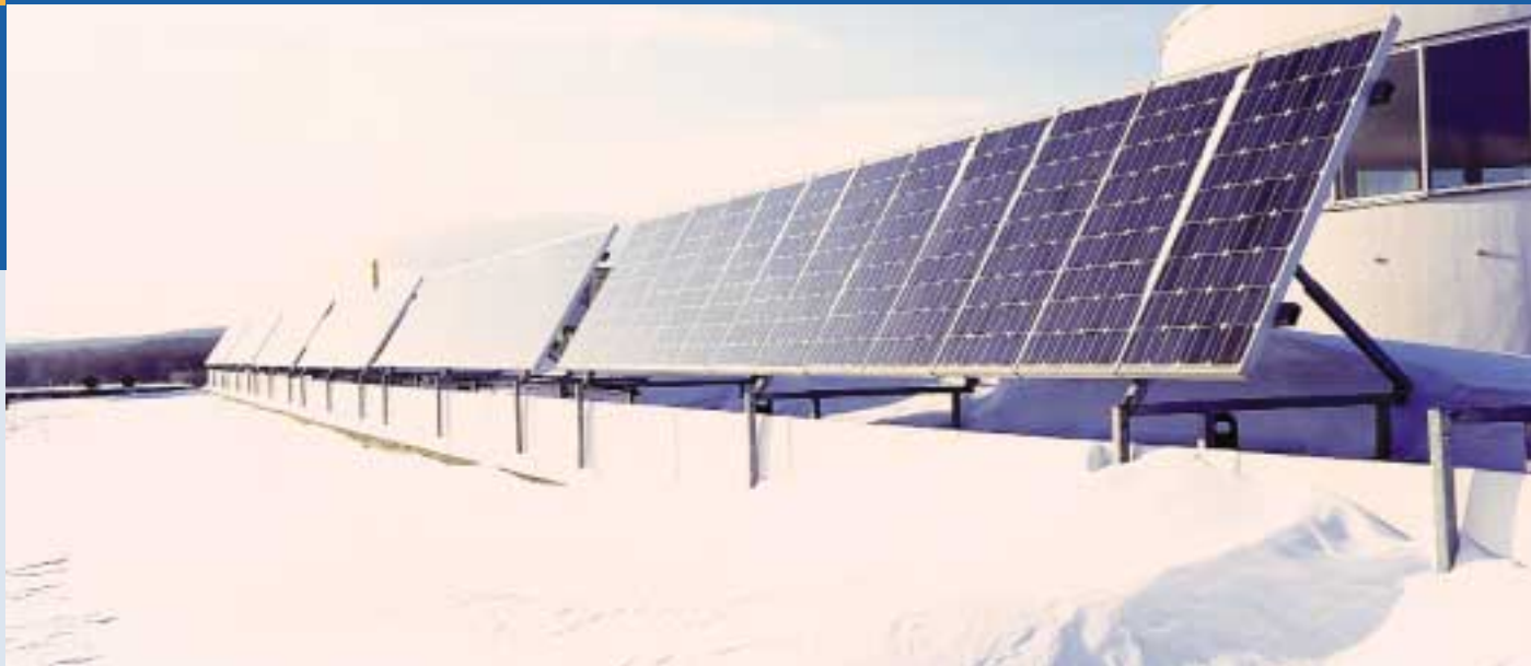
Fig. 2 – Grid-connected 3,24 kW roof-mounted sc-Si system for educational purposes at Borlänge University, Borlänge, Sweden. (Photo Carl Michael Johannesson, 2001)
