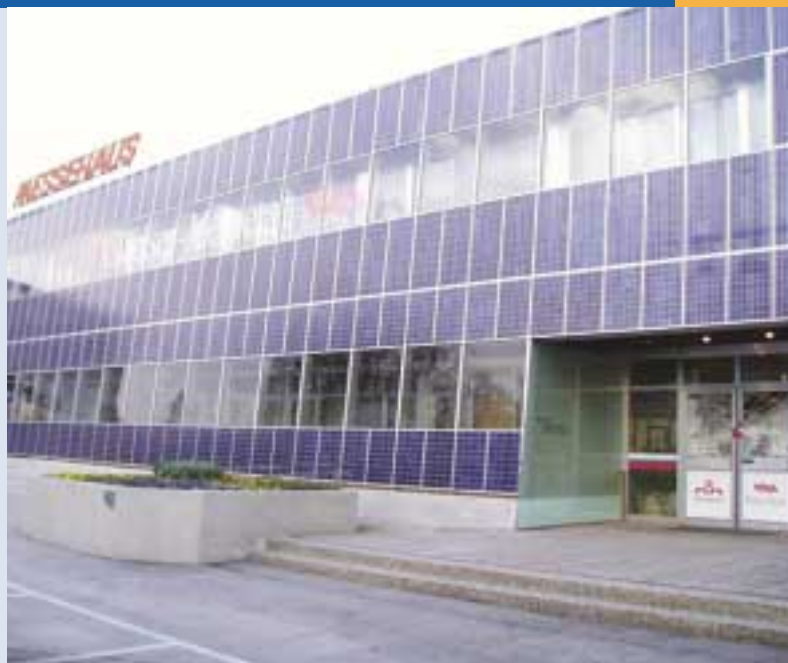
Fig. 4 - Refurbished PV façade at the Wels trade fair center, 17,24 kWp, stromaufwaerts GmbH.
