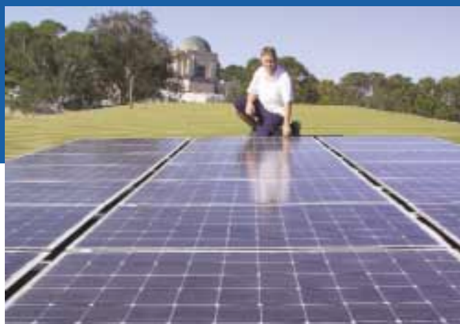
Fig. 1 – Plug & Power TM on Campbell High School in Australia's capital, Canberra, with the Australian War Memorial in the background. This is the first completely modular PV system to be installed on an Australian school and allows progressive expansion module-by-module in the years ahead.
