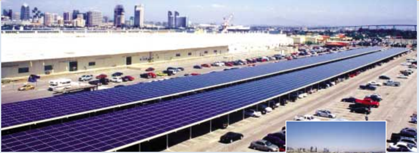
Fig. 4 and 5 - Naval Base in San Diego, California. This 924 kWp PV system provides long-term covered parking for over 400 vehicles while providing enough electricity to power more than 900 homes. (Photo Courtesy of PowerLight Corporation)
