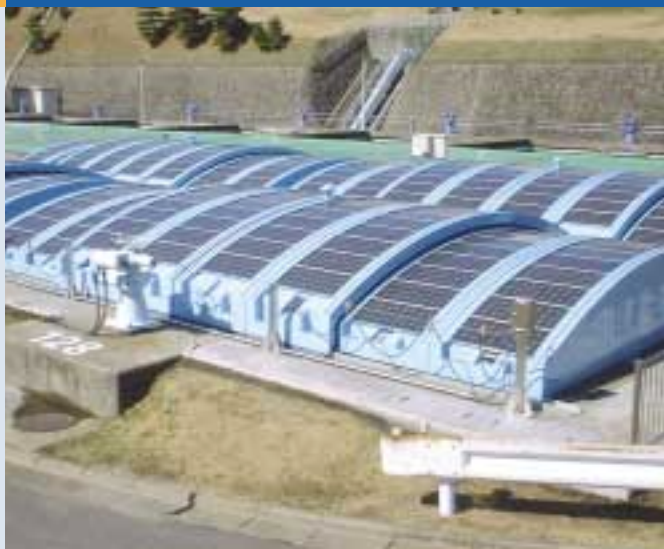
Fig.3 - 20 kW tank cover-integrated PV system for a water treatment plant of Yokohama-City of the Kanagawa Prefecture.
