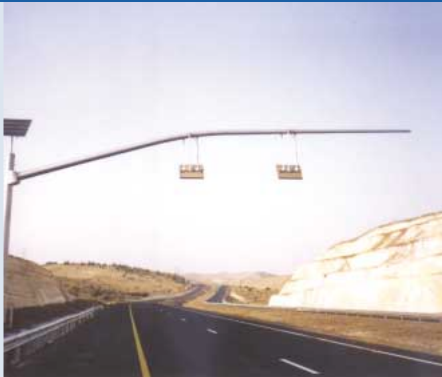
Fig. 1 - Traffic probe readers powered by PV panels on the new Cross-Israel Highway (Millennium Electric).
