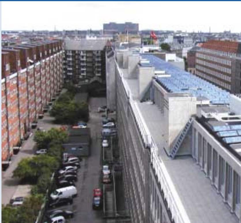
Fig. 2 - As a first part of the Sol 1000 project an office building in Copenhagen has installed a PV-system of 23,1 kWp on the roof and the façade.
