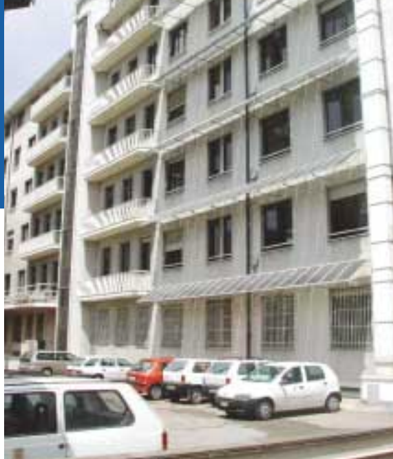
Fig. 1 - Italian Roof-top Program: photovoltaic modules mounted on shading elements at Turin.
