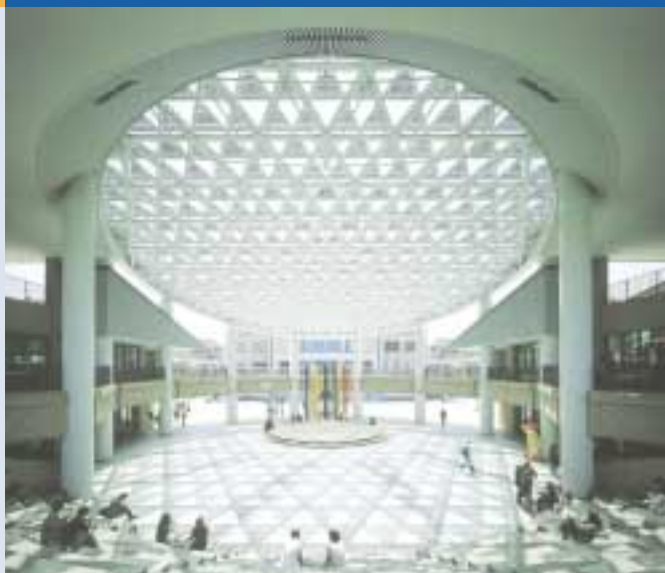
Fig.4 - Skylight PV system (20 kW) installed in Kansai Gaidai University in the Osaka Prefecture.
