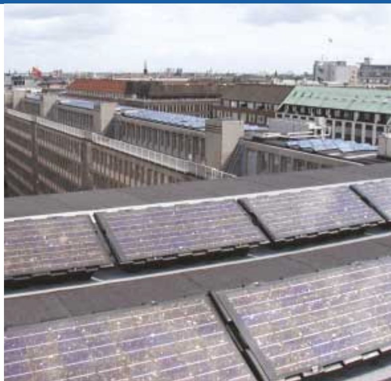
Fig. 1 - As a first part of the Sol 1000 project an office building in Copenhagen has installed a PV-system of 23,1 kWp on the roof and the façade.
