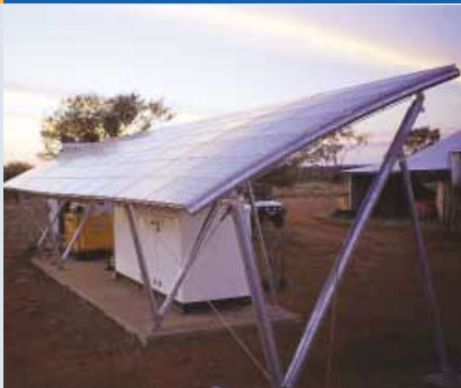
Fig. 4 – Welford power system in Queensland. Design & main structures by Ergon Energy station power: 6,3 kW PV array. Battery 120 V/1400 Ah. Inverter – 2 x 5 kW units operating in parallel to ensure continued operation. Installed May 2002.
