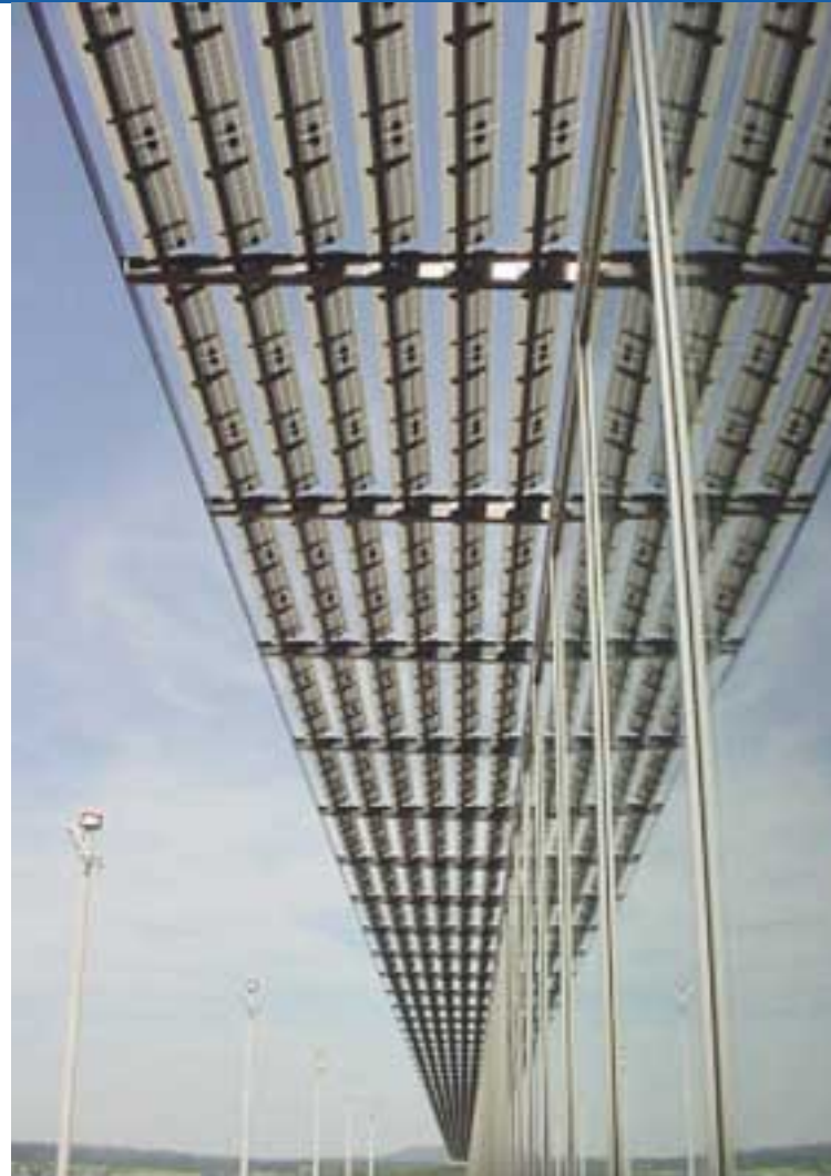
Fig. 1 - Dock Midfield: 283 kWp multifunctional system at the airport of Zurich.
