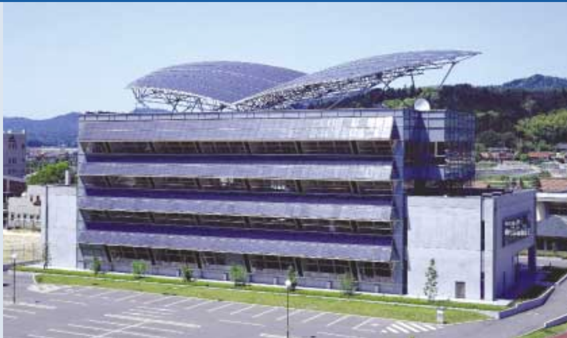
Fig. 2 - 150 kW PV system installed to the roof and façade of the municipal office of Chiyoda-Cho of the Hiroshima Prefecture.
