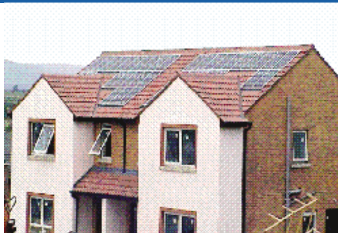
Fig. 1 – Steelstown Energy Programme, Northern Ireland. 51 kWp BP Solar laminates, installed under DTI Domestic Field Trial.
