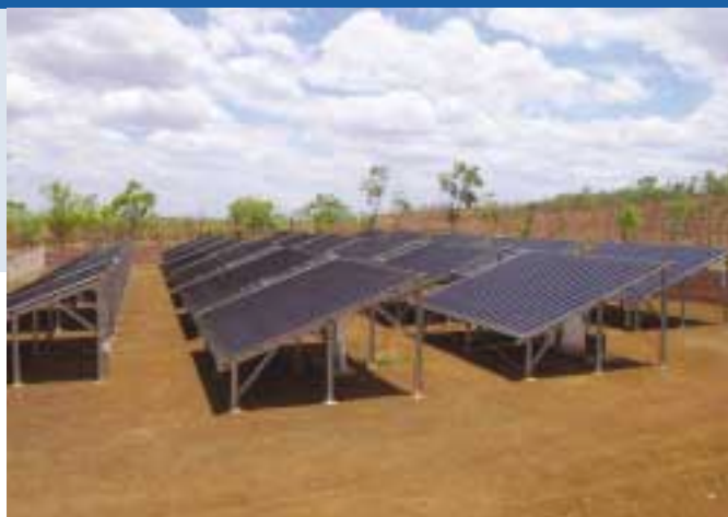
Fig. 3 - Power And Water Corporation's Bulman Solar Power Station. 56 kW of amorphous Silicon PV is displacing diesel fuel at this remote community in Arnhem Land, Northern Territory. The installation was commissioned in November 2002 with the aid of the Northern Territory Centre for Energy Research. (photo courtesy of Wolfgang Meike, NT Centre for Energy Research)
