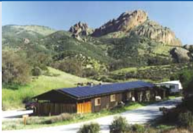
Fig.1 - Pinnacles National Monument: This 10 kW PV Power System provides power for the ranger station, visitor center well pump and other loads. (Photo Courtesy of NREL)
