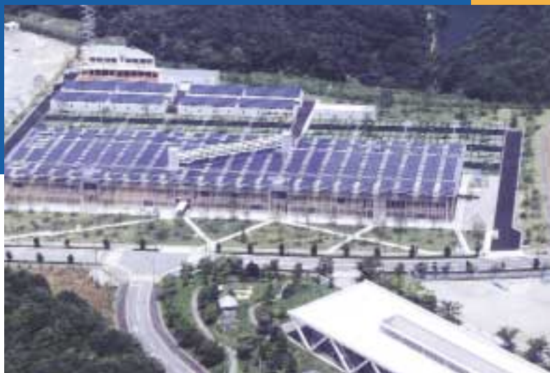
Fig. 1 - 506 kW PV system installed to the roof of Nishi-Harima Governmental Office Building of the Hyogo Prefecture .
