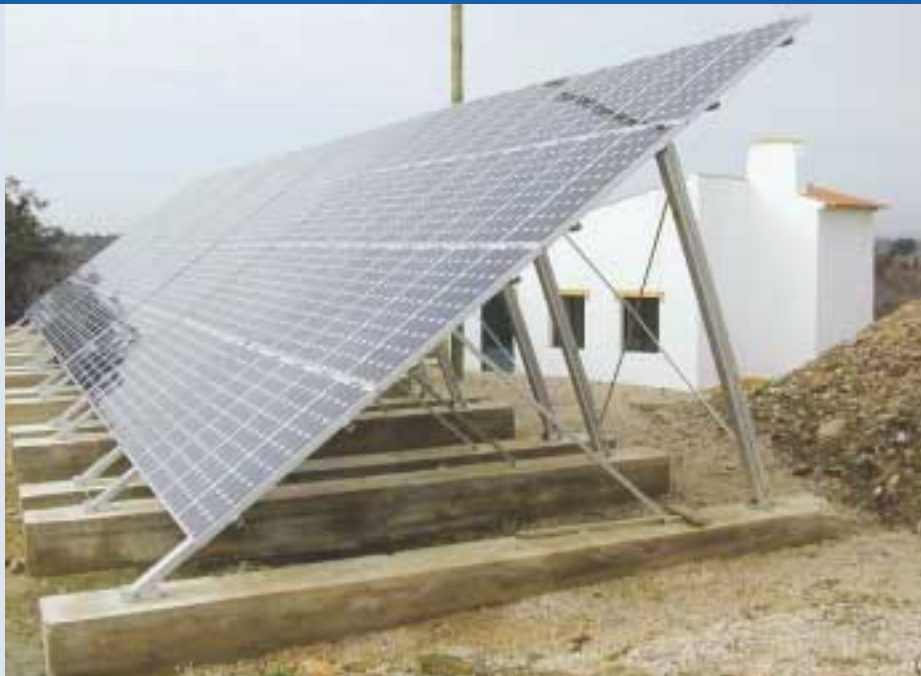
Fig. 2 - Centralised hybrid system (PV+diesel) for village supply. (Ourique)
