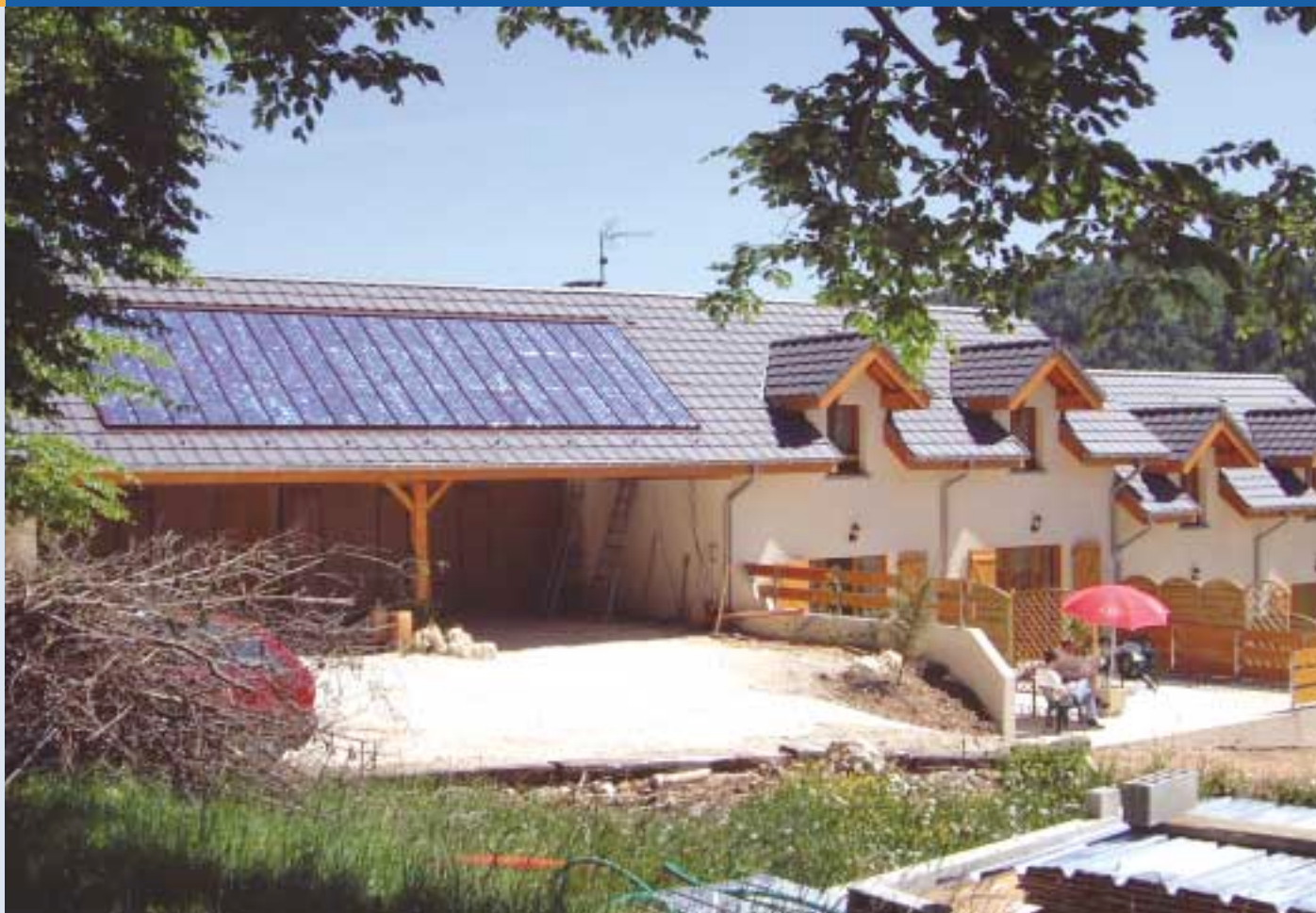
Fig.1 - 3 kW Roof Integrated Photovoltaic System. (Grenoble 38, Courtesy of Total Énergie)
