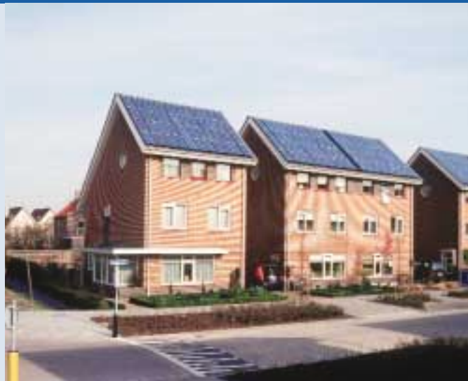
Fig. 3 - PV roofs on in Etter-Leur. Each house is supplied with a 2,7 kWp system.
