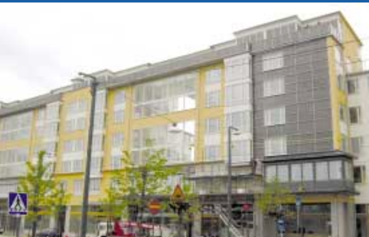
Fig. 1 - Photo of the NCC project Holmen in Hammarby Sjöstad. Semi transparent modules with a total peak power of 17,6 kW distributed on façade, windows, balconies and a small system on a roof window. Naps Sweden AB supplied the system. (photo Energibanken, 2003)
