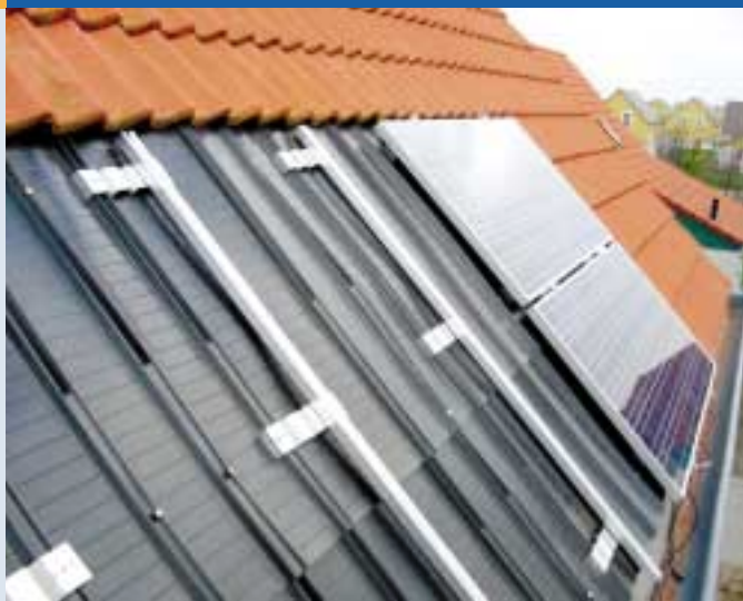
Fig. 2 - Thanks to the improved InterSole, integration of solar panels between the roof tiles is easier than ever.
