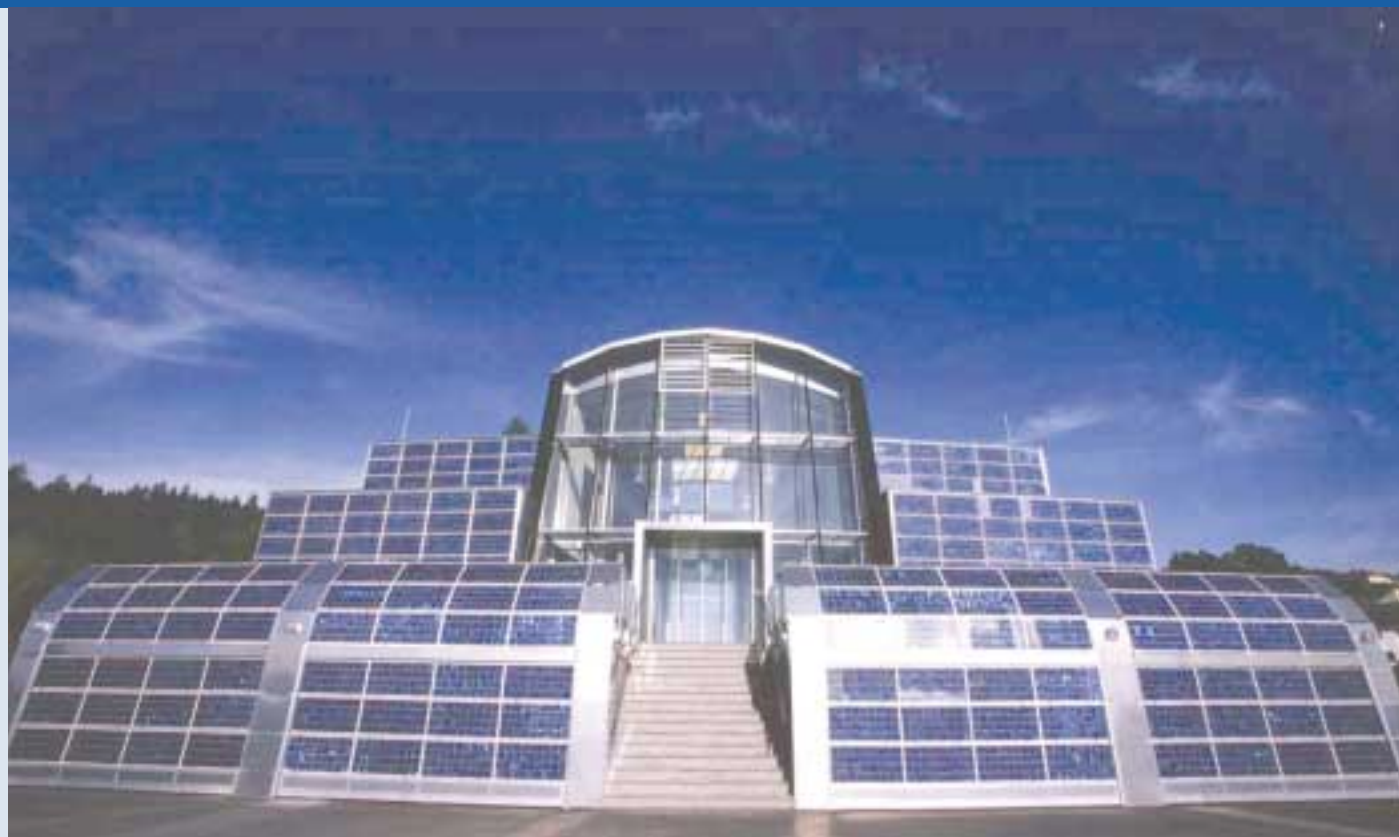
Fig. 1 - 22 kW PV System, Institute for Marketing, Upper Austria, KW-Solartechnik.
