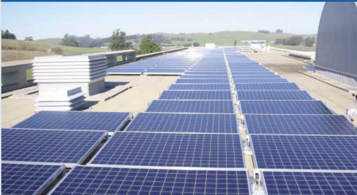
Fig. 4 - 125 kW PV system using RWE Schott Solar's FS mounting and ASE-300 PV modules at the U.S. Coast Guard Training Center in Petaluma, CA. (photo credit RWE Schott Solar, Inc.)
