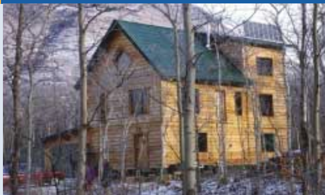
Fig. 4 - Canada's R&D programme is addressing the issues of integrating renewable energy in off-grid residences north of the 60° north parallel. This 600-Watt PV installation in an energy-efficient off-grid residence, Whitehorse, Yukon.
