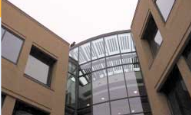
Fig. 5 - Atrium of the Waterloo City Hall building incorporating 1,1 kW of BIPV, Ontario. (photo ARISE Technologies Inc.)
