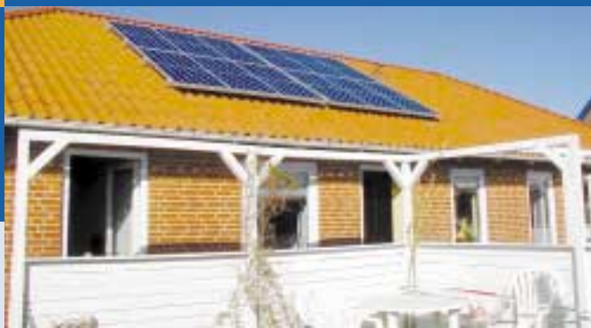
Fig. 2 - 2,04 kWp PV system on a typical residential house located the northern Jutland.
