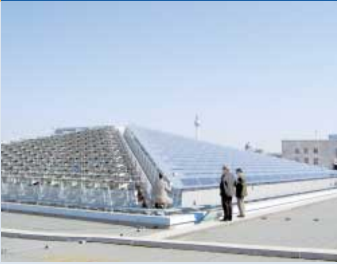
Fig. 4a - German Federal Council in Berlin: 21 kWp PV system as solar shading and light-directing system above the assembly hall. (photo Courtesy of Wolfgang Nasse)
