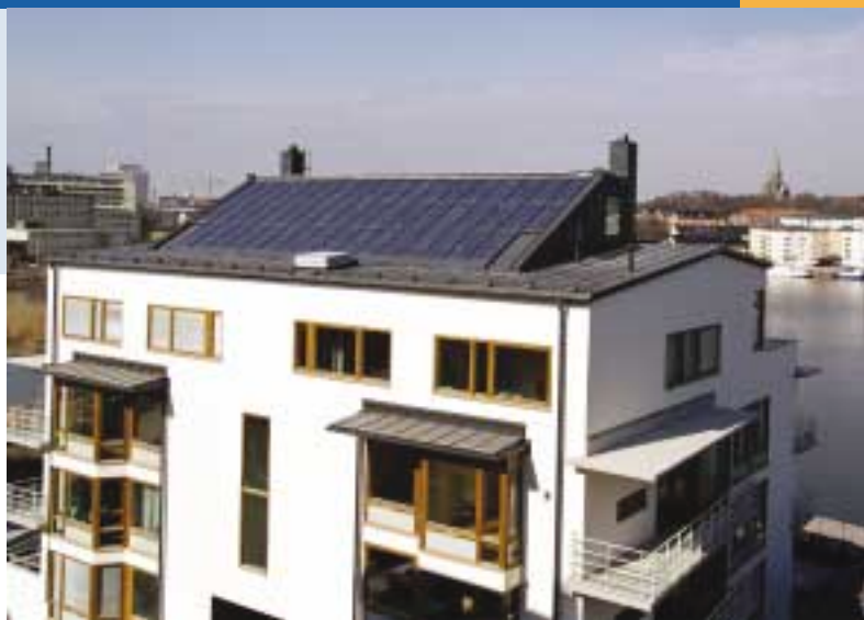
Fig. 3 - Photo of JM ABs and Fortum ABs architecturally building integrated PV-system in Hammarby Sjöstad. This is one of two similar buildings that have been equipped with semi-transparent modules in a glass-roof construction. The peak power of each installation is 5,7 kW. Naps Sweden AB supplied the systems. (photo Lars Hansson 2002)
