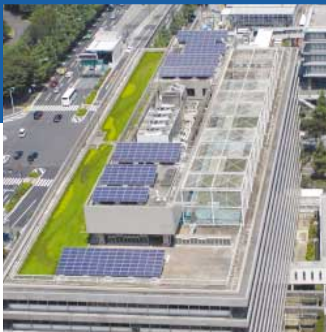
Fig. 1 - 45-kW PV system and the rooftop garden of the Central Government Building No. 4, Tokyo.
