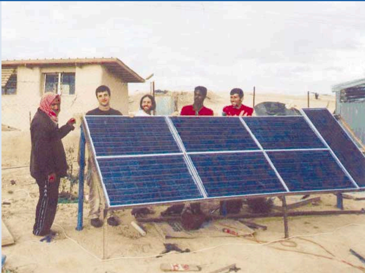
Fig. 2 - 600 W PV system providing electricity for lighting, computing and medicine refrigeration at a bedouin community. (photo SolarPower Ltd.)
