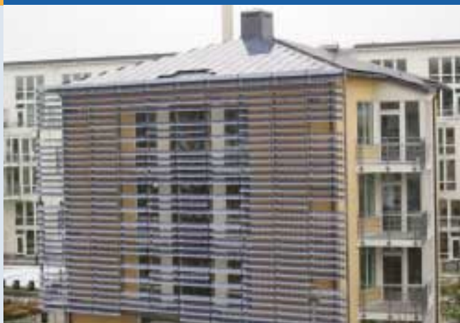
Fig. 2 - Photo of Familjebostäders project Lysande in Hammarby Sjöstad. The total peak power of the system is 22 kW. Semi transparent modules with a total peak power of 9 kW as shading device in front of the façade and 13 kW standard modules on the south, east and west sides of the roof. Gaia Solar in Denmark supplied the system. (photo Energibanken 2003)
