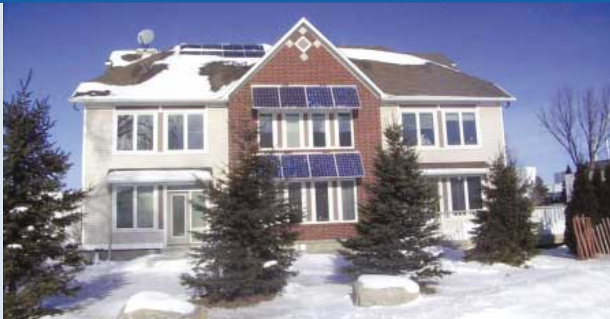
Fig. 1 – Solar PV installation (2,65 kW) at the Canadian Centre for Housing Technology, Ottawa, Ontario. (photo Sol Source Engineering)
