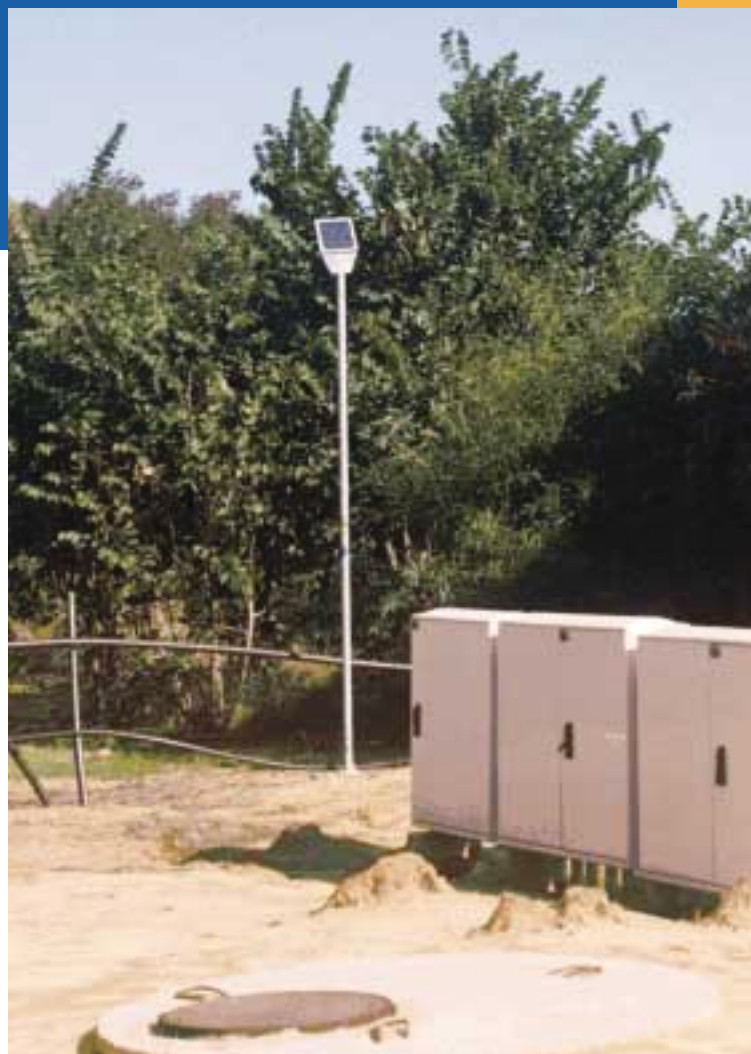
Fig. 1 - One of eight irrigation-control stations operated by a PV system, near Natanya. (photo SolarPower Ltd.)
