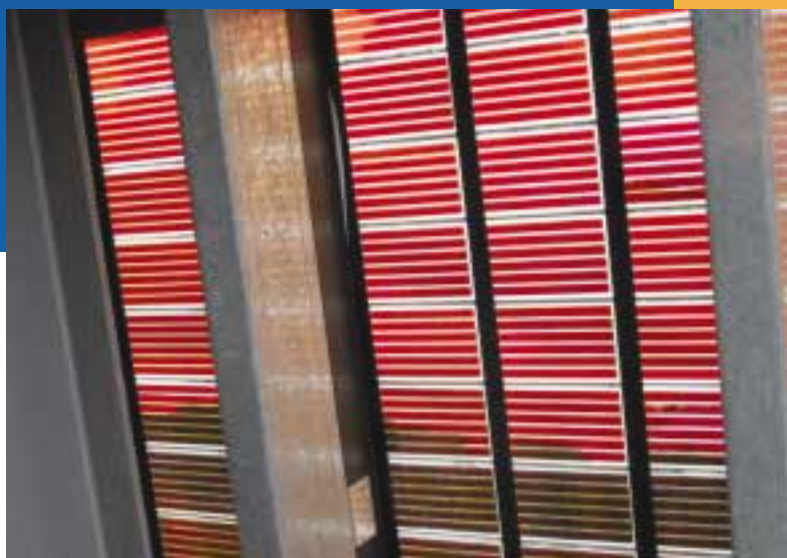
Fig. 1 – DSC façade on CSIRO Building, Newcastle. Photo: STI
