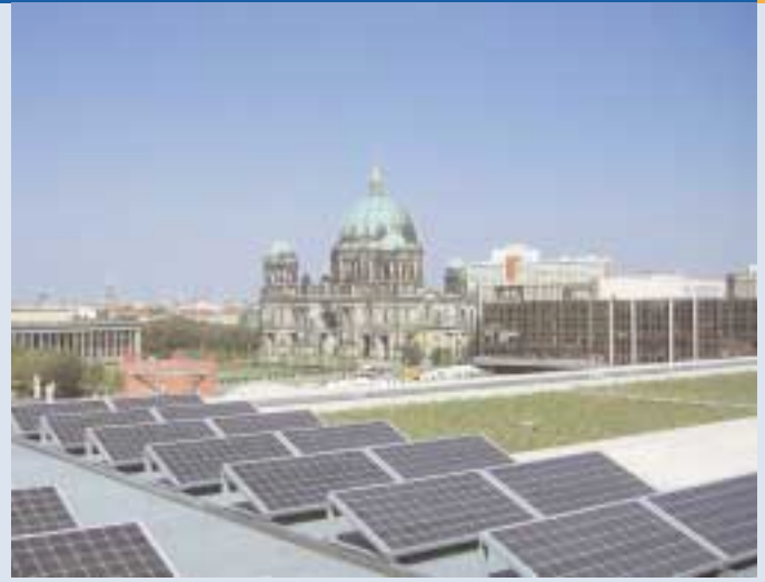
Fig. 4b - German Foreign Office in Berlin: 23 kWp PV system as add-on construction. (photo Courtesy of Thomas Nordmann)
