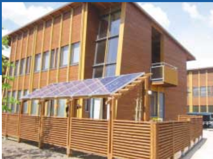
Fig. 1 - In 2003 a new office of Solpros, a consultant company working in the field of solar energy and environment, was opened. The building is a low energy house utilising photovoltaic power and passive solar energy. The estimated need for purchased energy is 50 kWh/m 2 annually. (photo Solpros, 2003)
