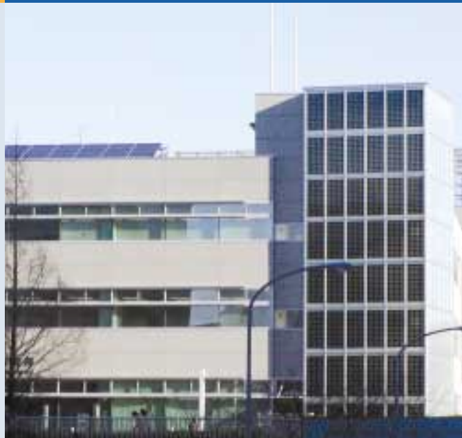
Fig. 2 - PV systems installed in the curtain wall (8,5 kW) and the rooftop (31,5 kW) of the Tsuzuki Post Office, Yokohama City, Kanagawa Prefecture.
