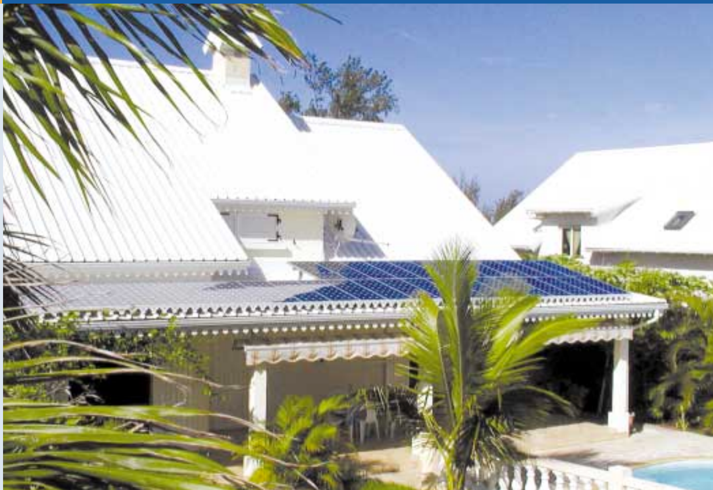
Fig. 2 – Réunion Island (French overseas department). Private house. 4 kW grid-connected PV. (photo Courtesy of Apex-Bp-Solar)
