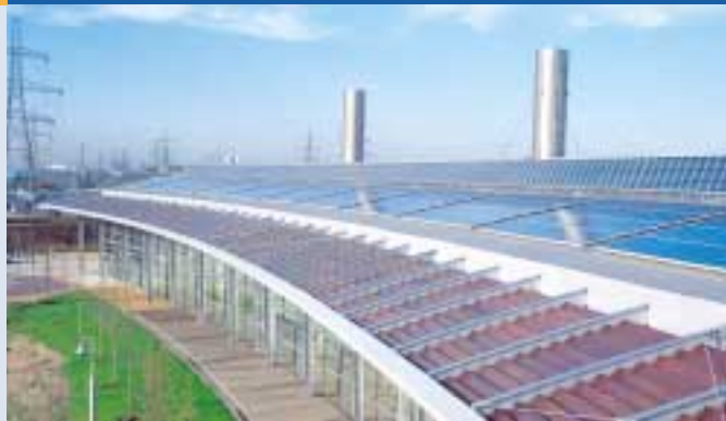
Fig. 2 - 115 kWp roof-mounted and glass-glass canopy at Ford's Centre for Engineering and Manufacturing Excellence in East London - largest installation in UK at time of commissioning.
