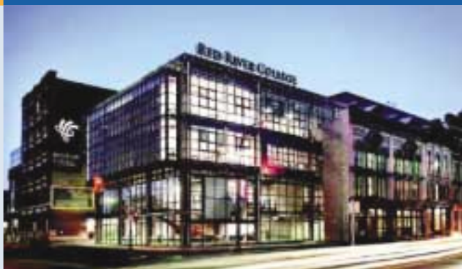
Fig. 2 – A BIPV façade (12,4 kW) at the Red River College Princess Street Campus, Winnipeg, Manitoba. (photo Corbett Cibinel Architects)
