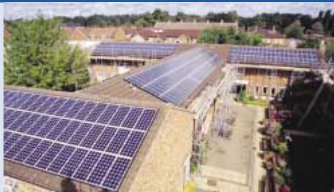
Fig. 3 - 99 kWp roof-mounted system on housing estate in Woking, Surrey.
