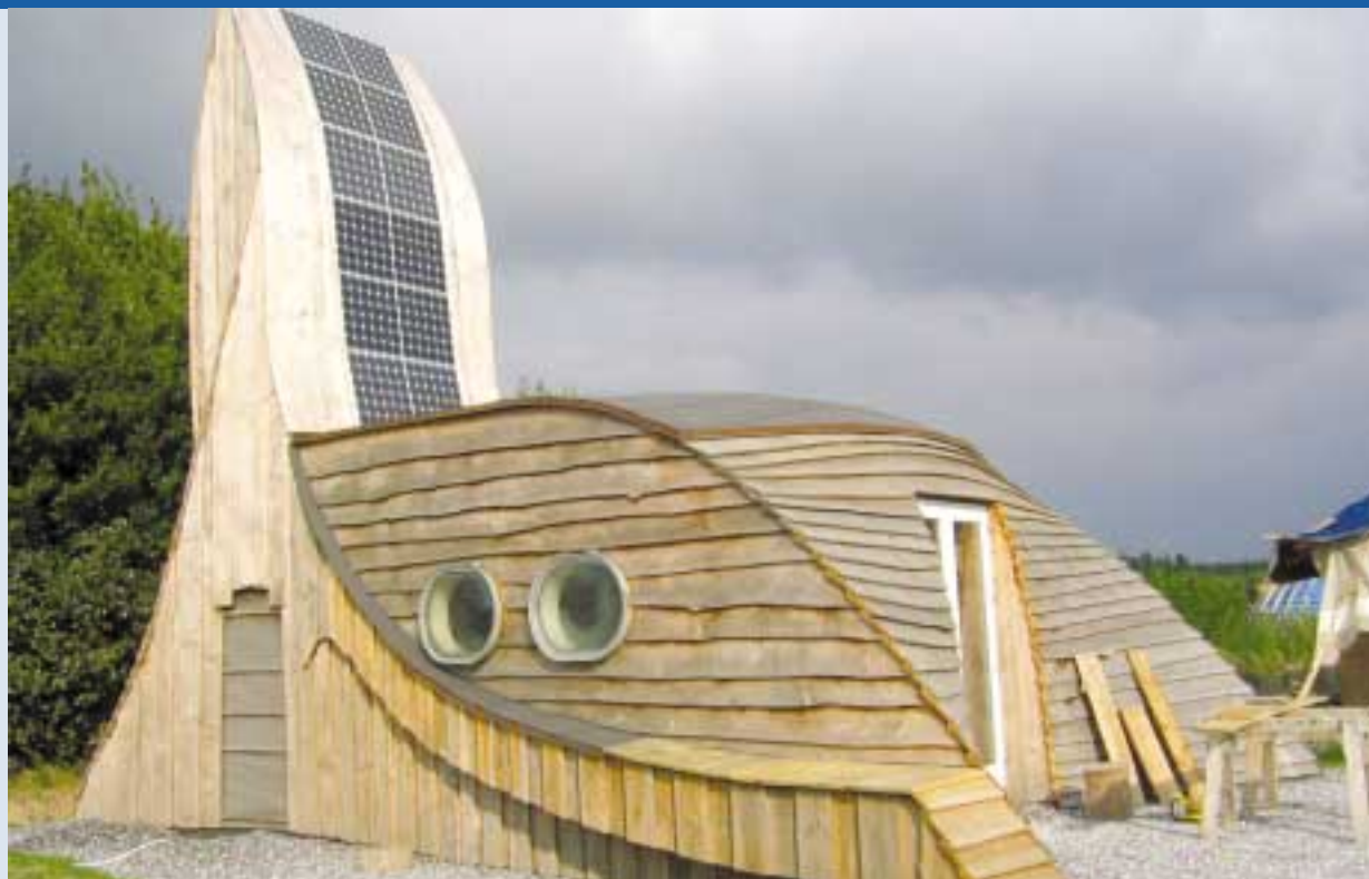
Fig. 1 – 1,02 kWp PV system on a house from Friland, an experimental area in Denmark for alternative buildings.
