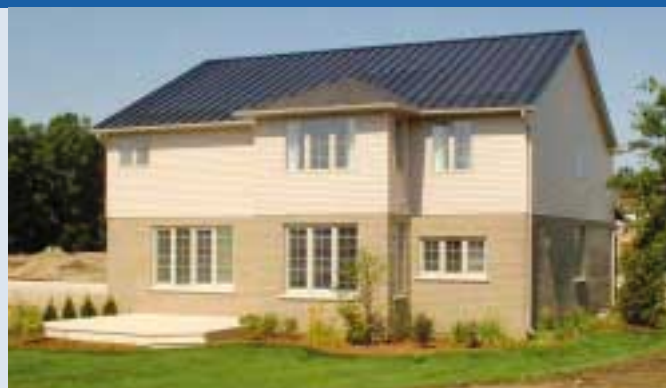
Fig. 3 – The Solar-Powered Rotary Dream Home, City of Waterloo, Ontario incorporated a 3 kW UniSolar metal roof as part of the first demonstration of community-scale PV rooftop systems in a neighbourhood in Canada. (photo ARISE Technologies Inc.)
