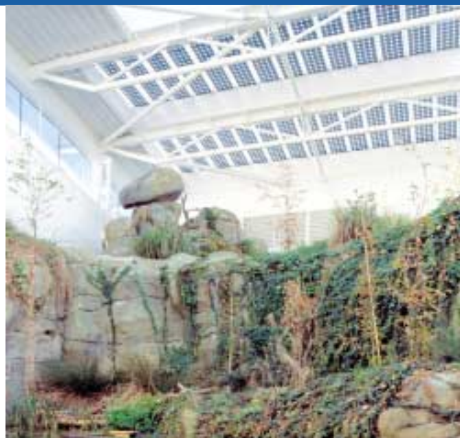
Fig. 1 - 30 kWp glass/glass laminates at the National Marine Aquarium, Plymouth.
