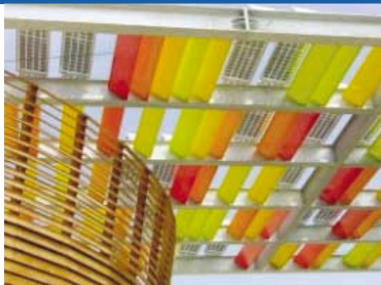
Fig.1 - Pic Saint Loup School (Hérault dpt). European Universol project. 5 kW grid-connected PV canopy. (photo courtesy of Hespul and Apex)
