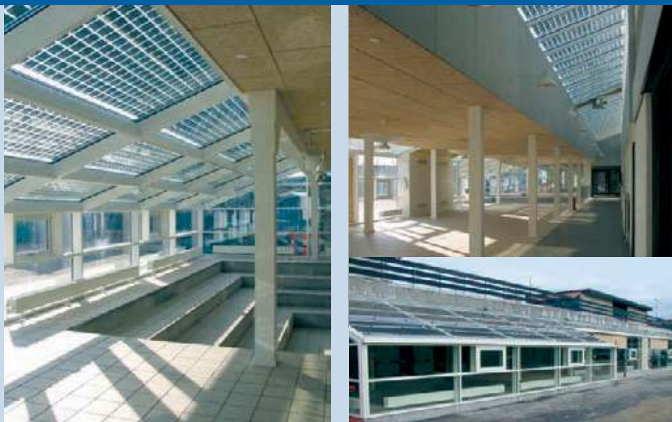
Fig. 1 - The Tjornehojskolen School, Copenhagen. A fully integrated PV system of 17,4 kWp.
