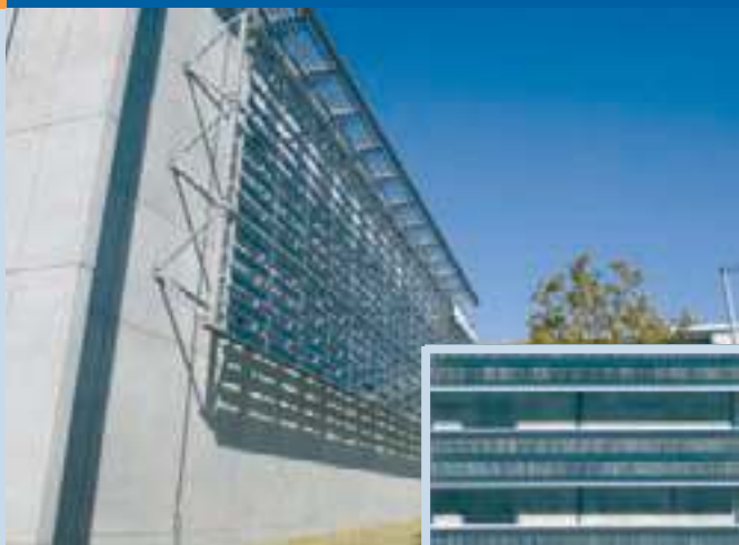
Fig. 5 - Louver integrated PV system installed in the showroom of Panasonic Center, 12,12 kW, Koto-ku, Tokyo.
