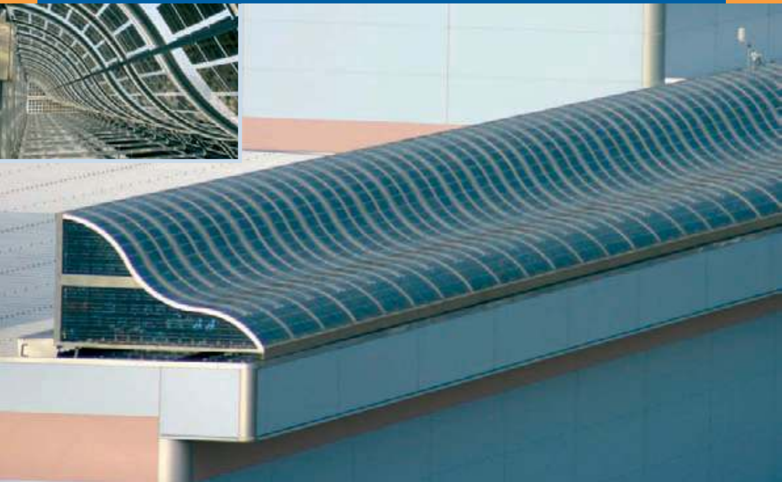
Fig. 6 - PV system using curved crystalline silicon modules installed in Fujipream Kohto Factory, 21,66 kW, Ibo Gun, Hyogo Prefecture.
