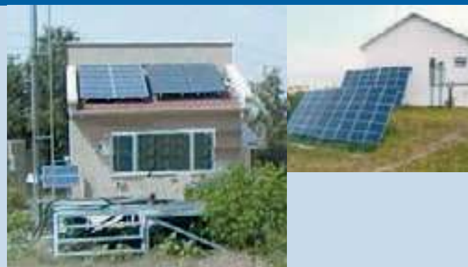
Fig. 5 - 4,8 and 1,2 kWp Grid-Connected Photovoltaic systems of EIE.
