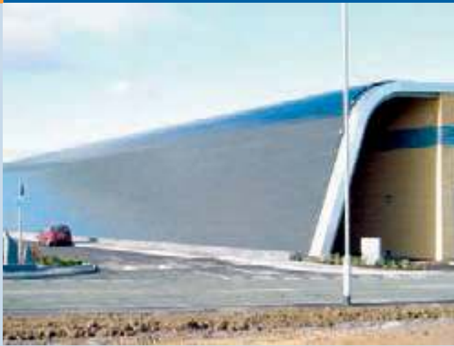
Fig. 4 - 85 kW CIS 'solar wall' in Denbighshire, North Wales –the world's largest single CIS PV installation (photo EETS).
