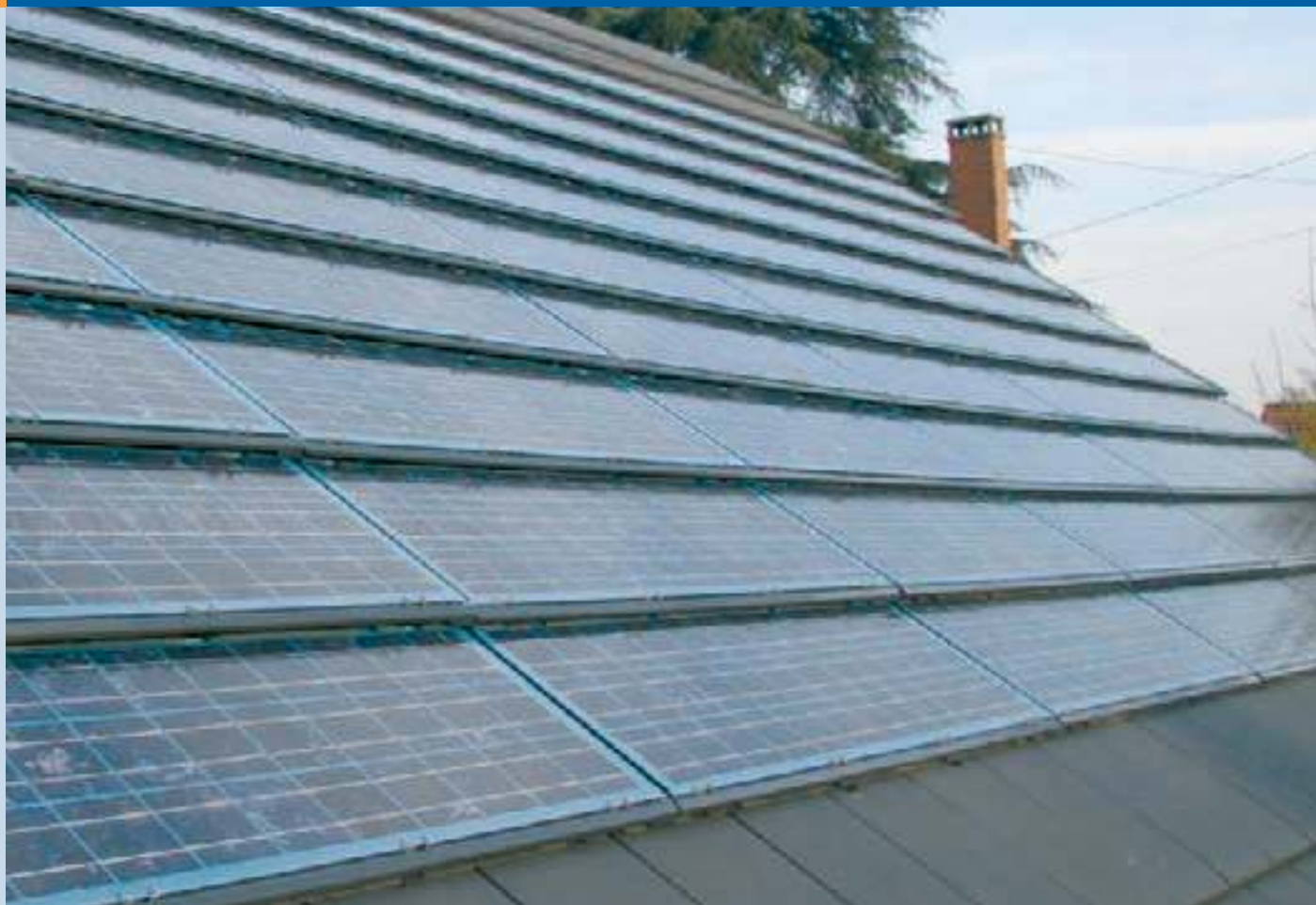
Fig. 2 - PV STARLET project, "SUNSAT" PV tile (photo courtesy of Imerys Toiture/Hespul).
