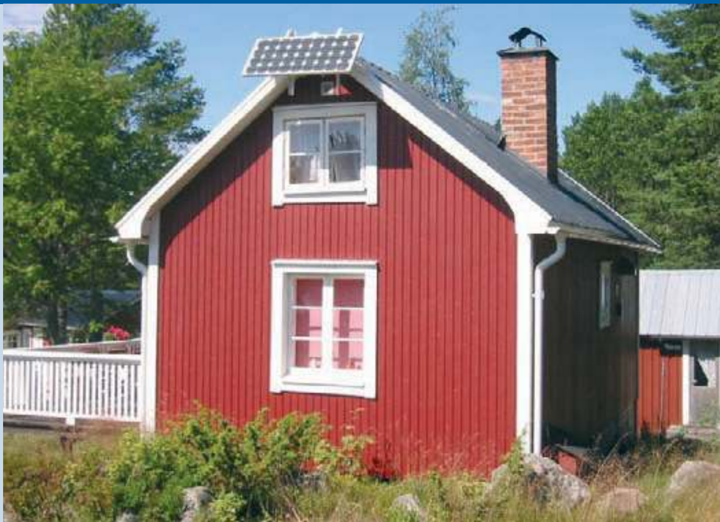
Fig. 1 - The majority of the Swedish PV installations are small domestic off-grid systems such as this module on a summer cottage in the Stockholm archipelago (photo Energibanken AB).
