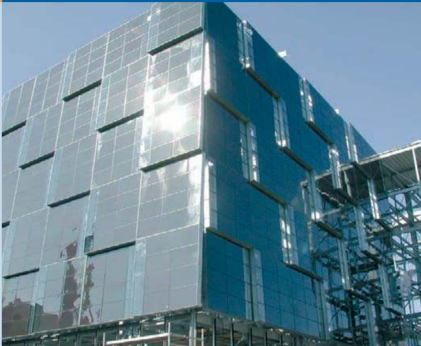
Fig. 3 - Amorphous silicon façade on a parking garage in Zwolle (photo Oskomera).
