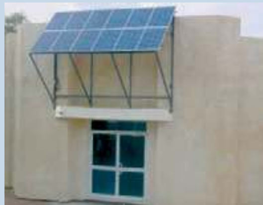
Fig. 3 - 1 kWp grid-connected system in the Arava (photo SolarPower).
