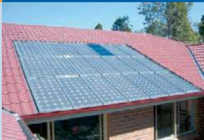
Fig. 3 – Pennant Hills 1,5 kWp PV tiles with skylight (photo PV Solar Tiles).
