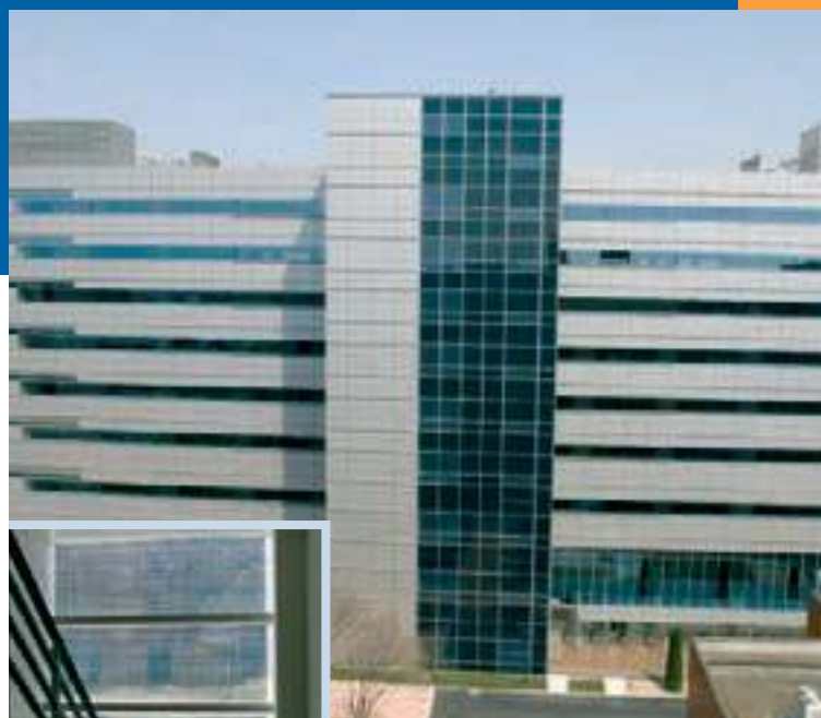
Fig. 1 - PV system using transparent sc-Si cells, installed in National Institute of Advanced Industrial Science and Technology (AIST), 41 kW, Tsukuba City, Ibaraki Prefecture.
