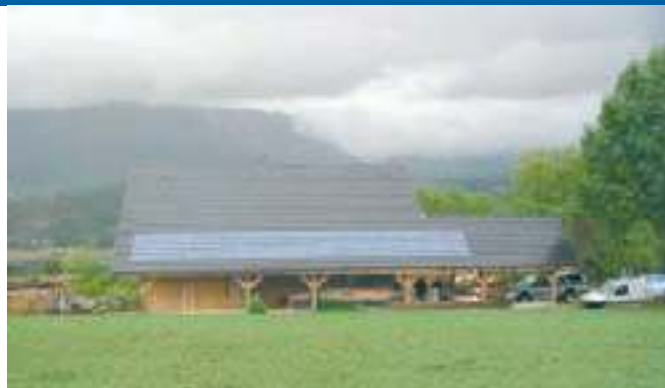
Fig.1 - PV-STARLET project, Nattages Charmont (Ain): 4 kW BIPV (photo courtesy of Imerys Toiture/Hespul).
