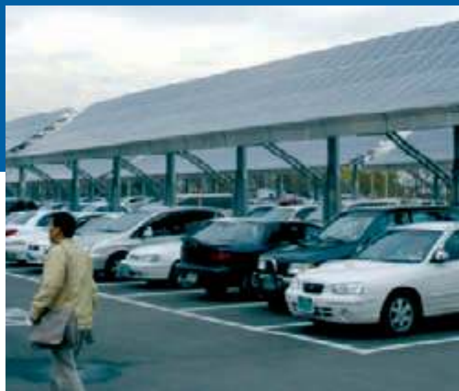
Fig. 1 - 100kWp grid-connected PV systems installed at a parking place inside Gwangju metropolitan city hall, under the Local Energy Development Programme, in 2004.
