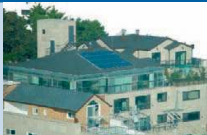
Fig. 5 - 3kW grid-connected PV systems installed at private residential houses under the Program of Local Energy Development Program in 2003.
