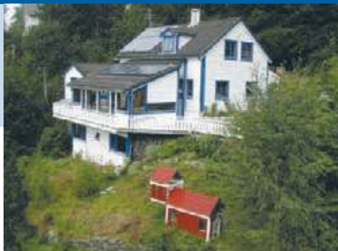
Fig. 2 - Private house with 1,2 kWp solar cells in Bergen (photo Nakling).
