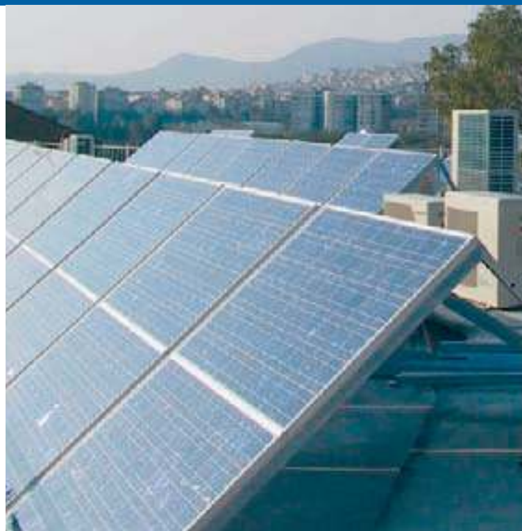
Fig. 1 - 11 kWp Grid-Connected Photovoltaic systems of Solar Energy Institute in Izmir.
