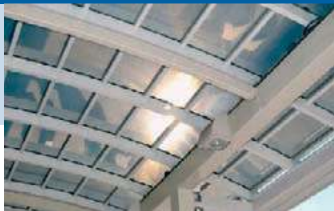
Fig. 4 - Transparent PV on BP Gas Station Canopy in Denver, Colorado. The PowerView Semi-transparent PV modules are a novel system that serves as partial skylight and power generation. It is envisioned these panels will become a functional replacement for glass in walls, skylights, atriums in modern architecture (photo courtesy of Warren Gretz).
