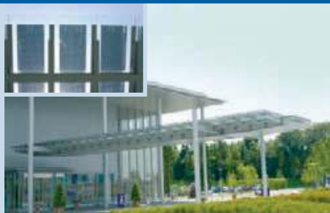
Fig. 3 - PV system installed in the canopy at Suntory Kyushu Kumamoto Plant, 2,16 kW, Kami-Mashiki Gun, Kumamoto Prefecture.
