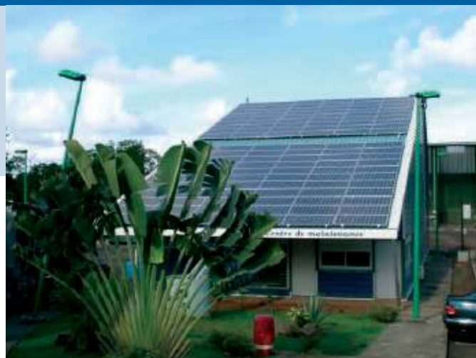
Fig.2 - Grid-connected PV system, 22 kW roof of waste treatment centre - Martinique Island (photo - courtesy Apex BP Solar).
