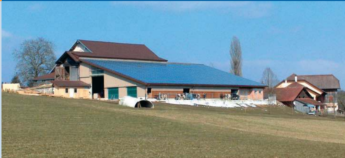
Fig. 2 - 110 kWp roof integration on a farmhouse with Solrif® frames (PV design: Solstis, photo NET).
