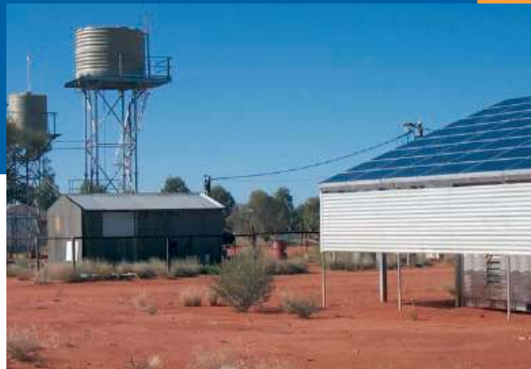
Fig. 1 - PV system for a remote railway bore pump (photo BCSE).
