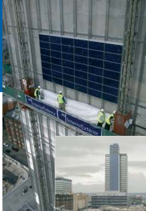
Fig. 1 – The 391 kW PV system on Manchester's CIS building will be Europe's largest vertical solar façade.
