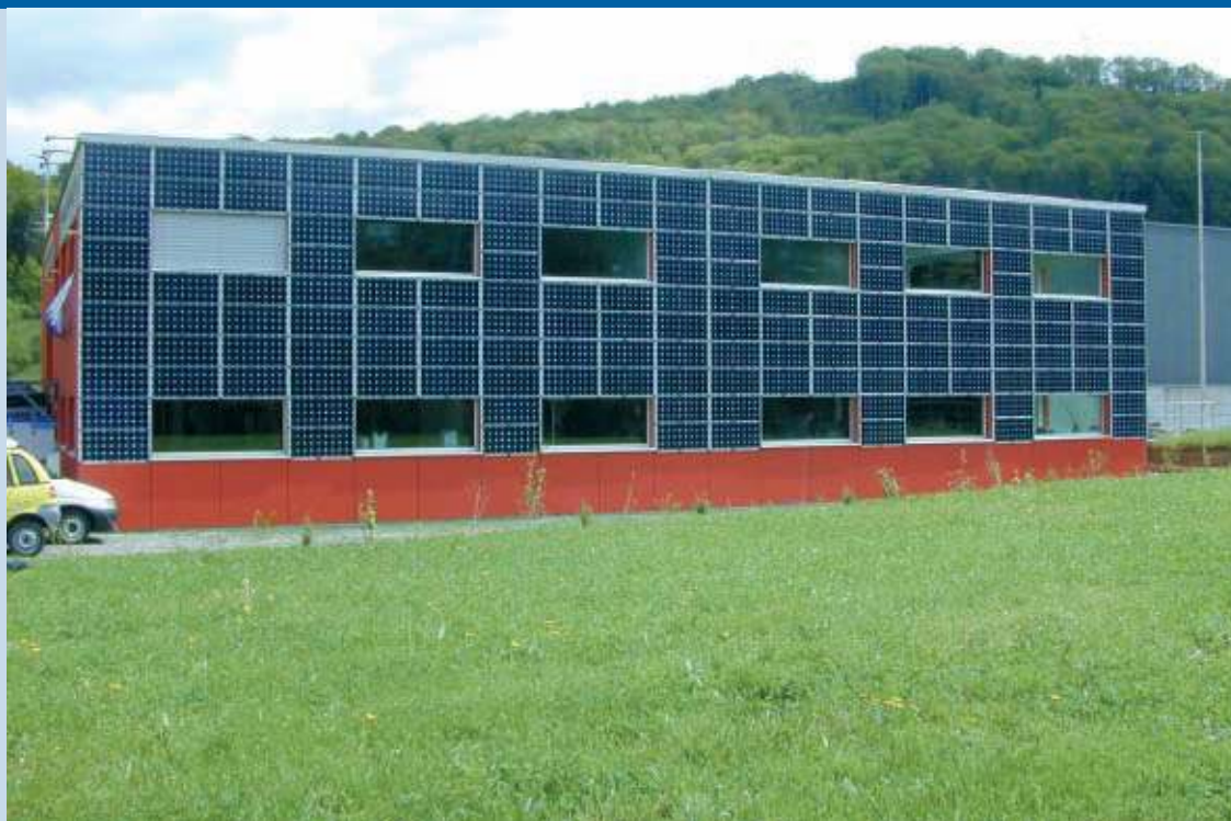
Fig. 3 - 12 kWp facade system on the highly energy efficient commercial building Wattwerk (PV design: Holinger Solar, photo NET).
