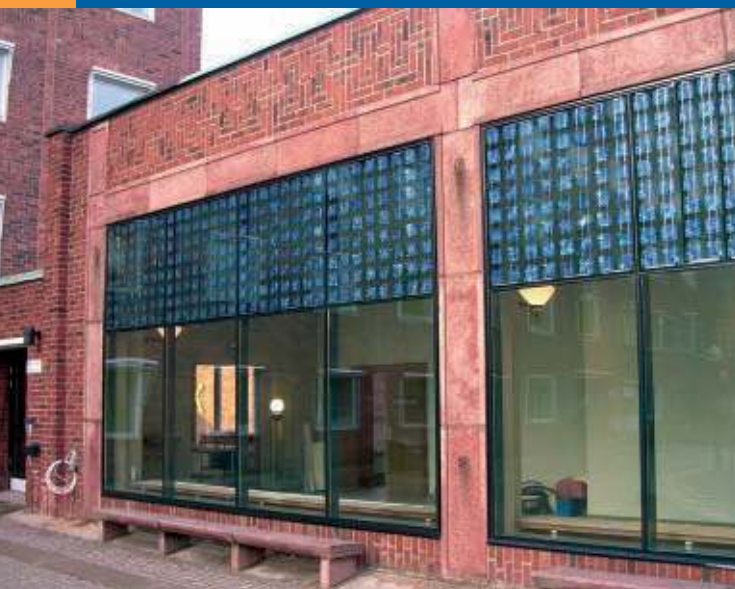
Fig. 1 - A 3 kWp semitransparent PV installation at the Royal Institute of Technology, Stockholm. The system has been in operation since January 2006 (photo Energibanken AB).
