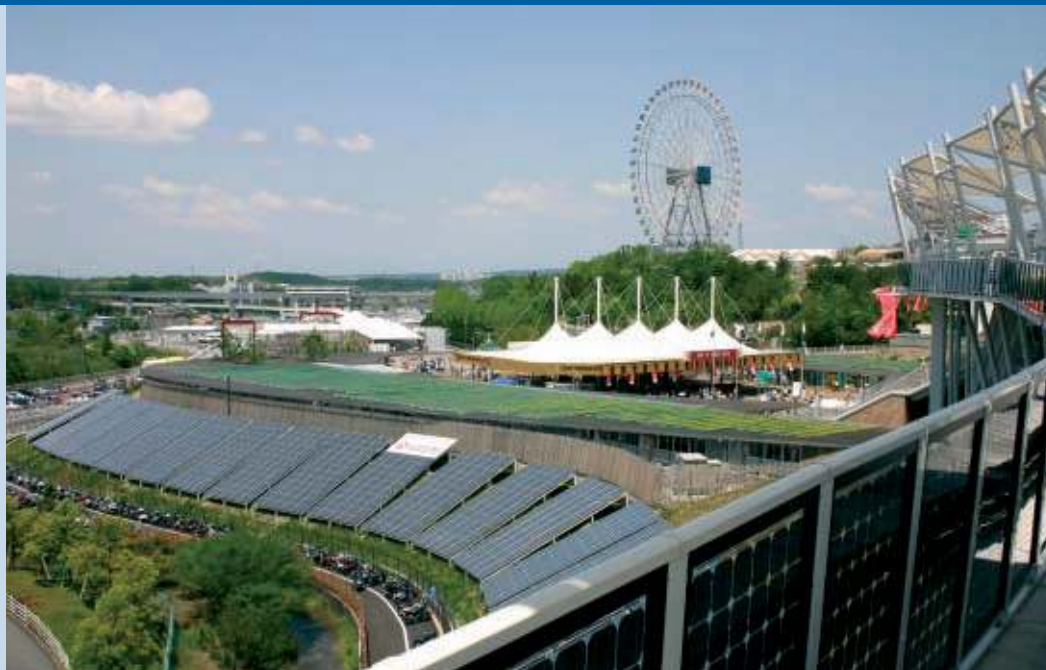
Fig. 1 - 30-kW Bifacial type PV system (front), 200-kW PV System installed on the slope (back), Aichi EXPO.
