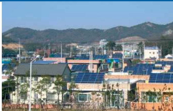
Fig. 1 - PV powered Green Village in Kwangju Metropolitan City under the 100 000 Rooftop Programme. Total 96,9 kW grid-connected PV systems are installed on the roof of 46 residential homes.
