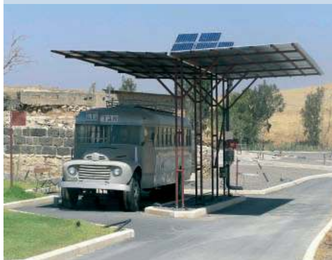
Fig. 3 - 400 W grid-connected system, at a transportation museum in the Jordan Valley (photo SolarPower).
