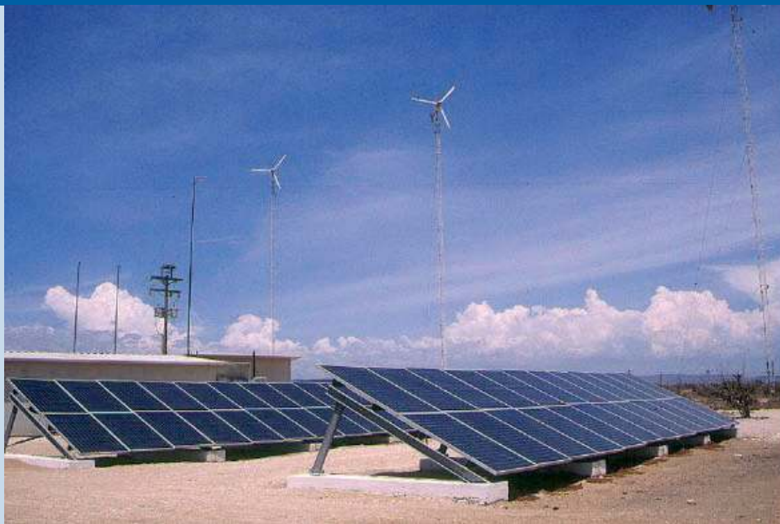
Fig. 1 - San Juanico PV-Wind Diesel Hybrid and mini-grid system in operation since 1999.
