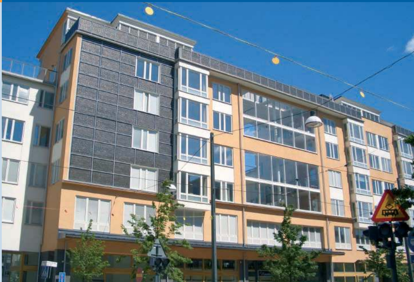
Fig. 2 - The Grynnan Building in Hammarby Sjöstad, Stockholm, is the second in a pair with PV integrated into the facade, balcony railings and semi-transparent windows. The 17 kW PV installation was planned at an early stage of the building process and in close co-operation between architects, builders and PV installers (photo Ulf Malm).
