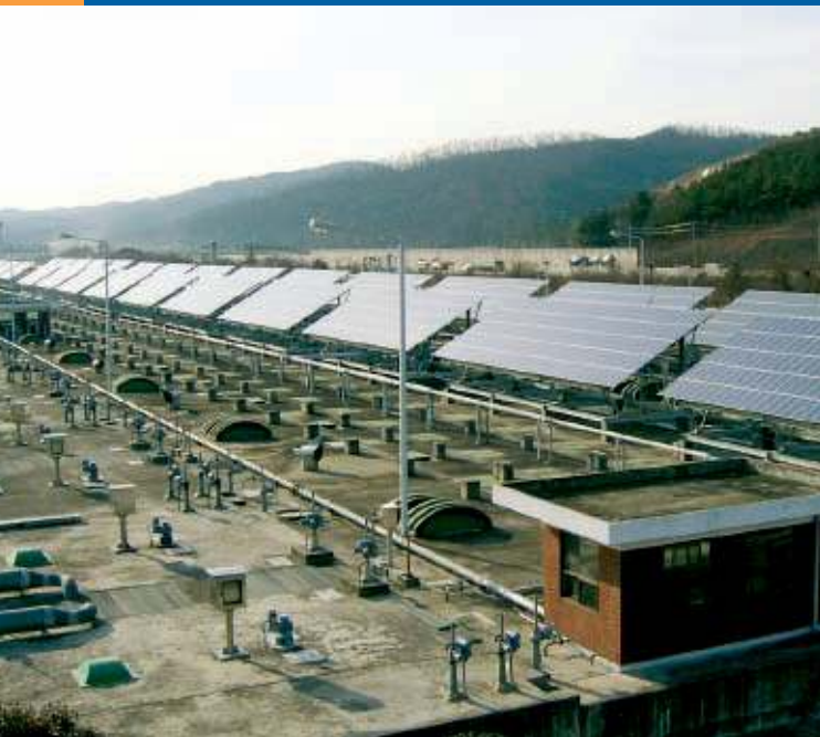
Fig. 2 - The 479 kW grid-connected PV systems for a sewage treatment plant in Daegu Metropolitan City under the Local Energy Development Program in 2004: The PV provides about 1,1 % of the plant's total electricity consumption.
