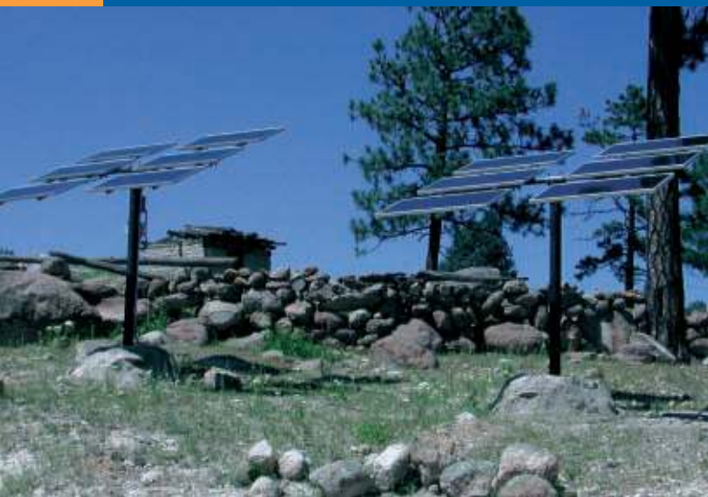
Fig. 2 - PV pumping system provides drinkable water to rural communities.
