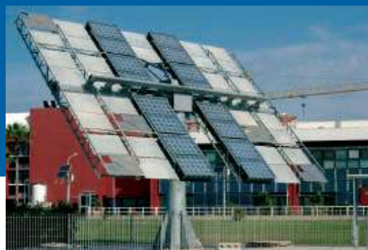
Fig. 1 - PhoCUS Project: the first 5 kW prototype (photo ENEA Research Centre).
