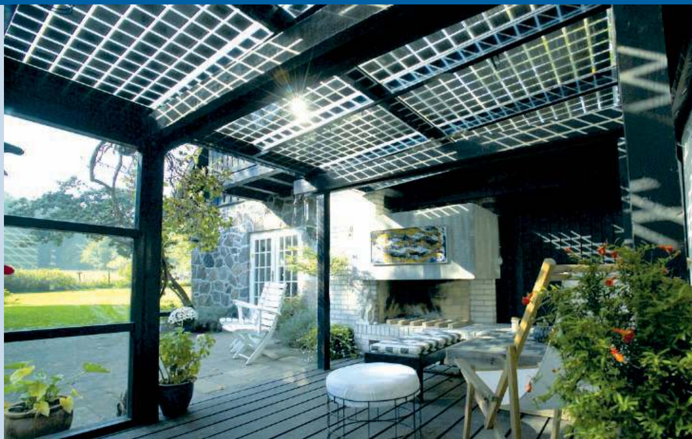
Fig. 1 - Transparent solar modules as roof on patio.
