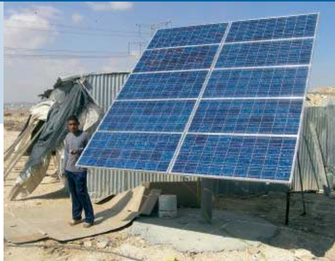
Fig. 2 - 1 200 W off-grid system, providing electricity to a Bedouin family (photo SolarPower).
