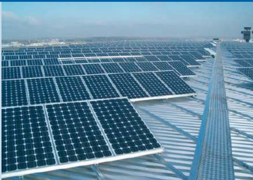
Fig. 1 - 280 kWp flat roof system at Geneva airport with AluStand® mounting system (PV design: Enecolo, photo Urs Bühler).
