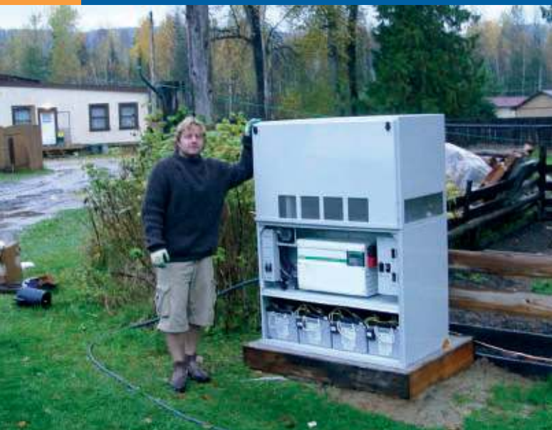
Fig. 2 - Hybrid Remote Area Power Systems at Seymour Arm, British Columbia - a complete turn-key solution for off-grid power supply by Xantrex Technology Inc. (photo by Xantrex).
