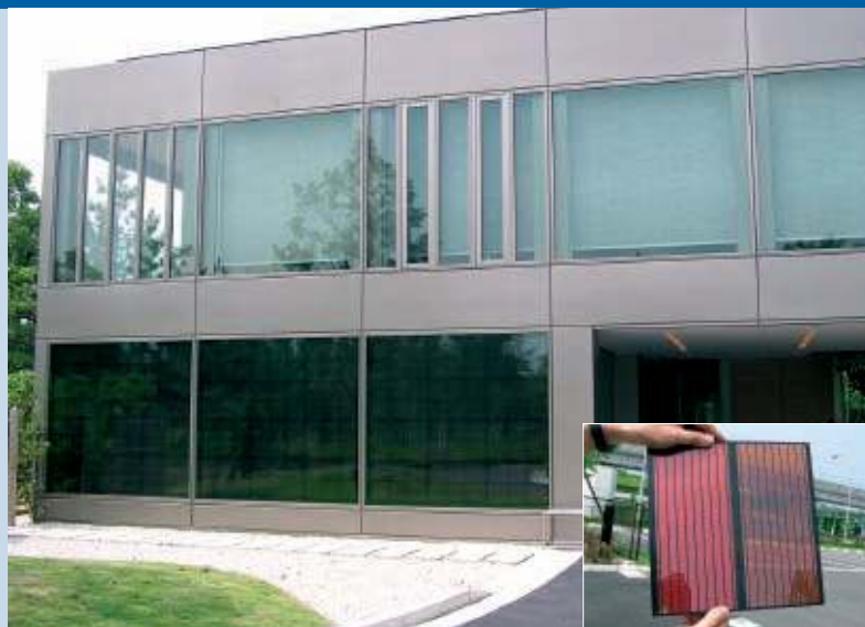
Fig. 7 - PV system using Dye-sensitized Solar Cell (DSC) at Toyota Dream House "PAPI", Nagakute Town, Aichi Prefecture.
