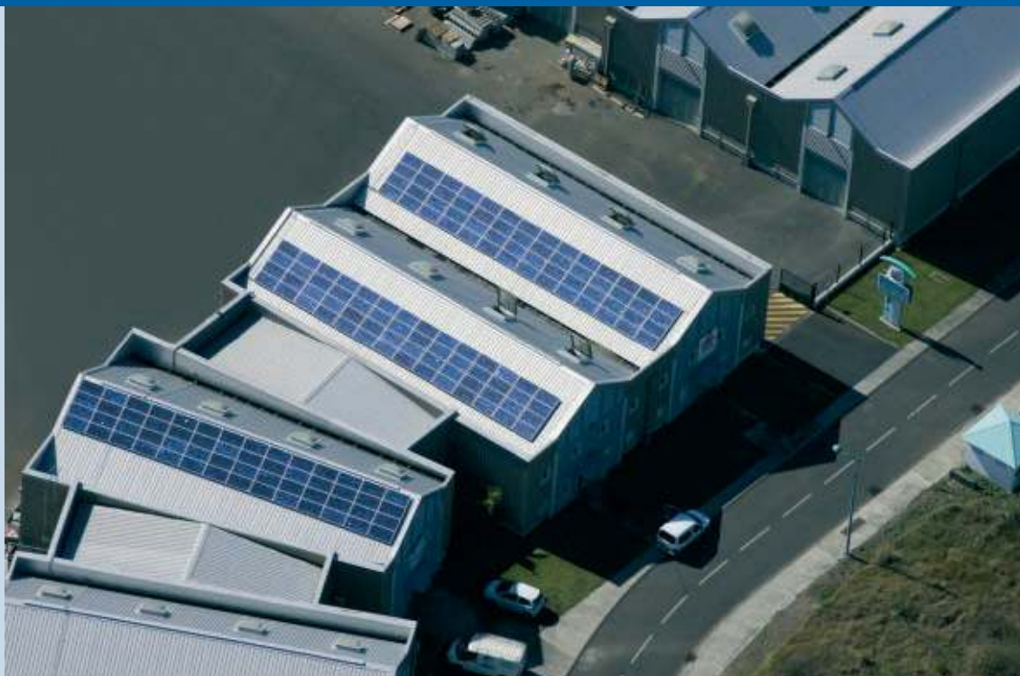
Fig.1 – Grid-connected PV system, 32 kW – Réunion Island (photo –courtesy Apex BP Solar).
