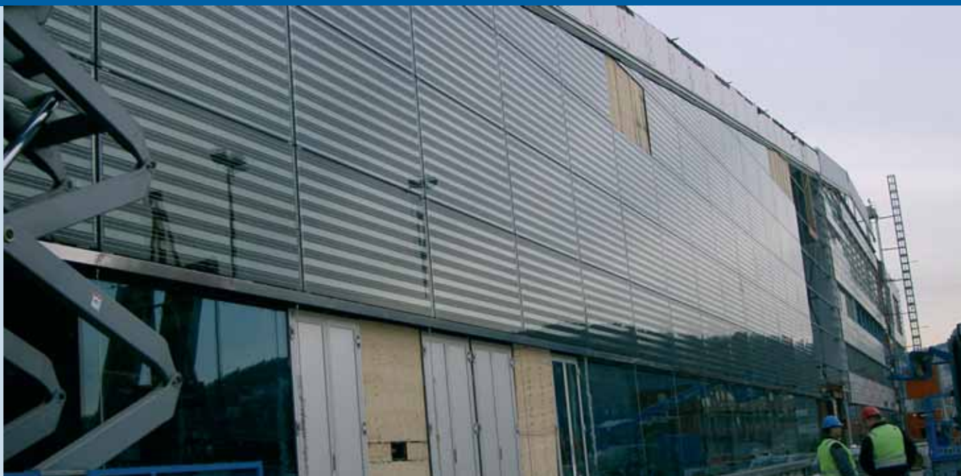
Fig. 1 - Semitransparent solar cells under installation at the new opera house in Oslo (photo Ida Bryhn, Erichsen & Horgen AS).
