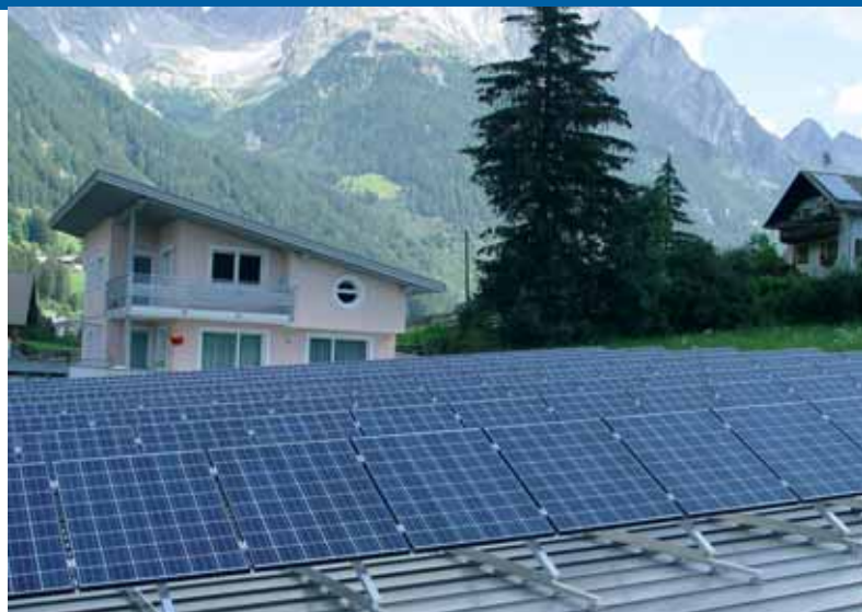
Fig. 1 – Grid-connected 26,7 kW PV system on flat roof in Anterselva, Bolzano, Italy.
