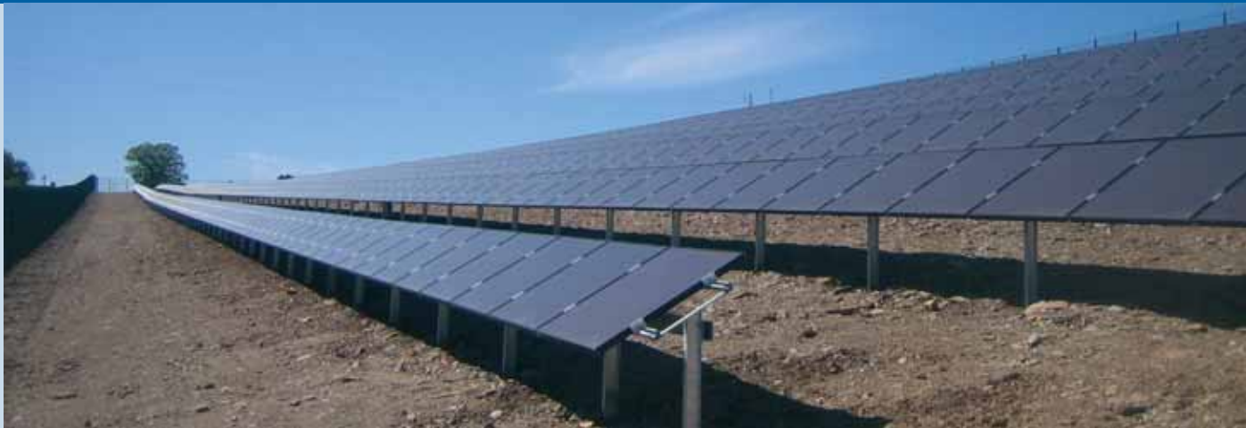
Fig. 1 - 124 kWp amorphous silicon plant (Lamelas) (photo courtesy of Jayme da Costa, S.A.).
