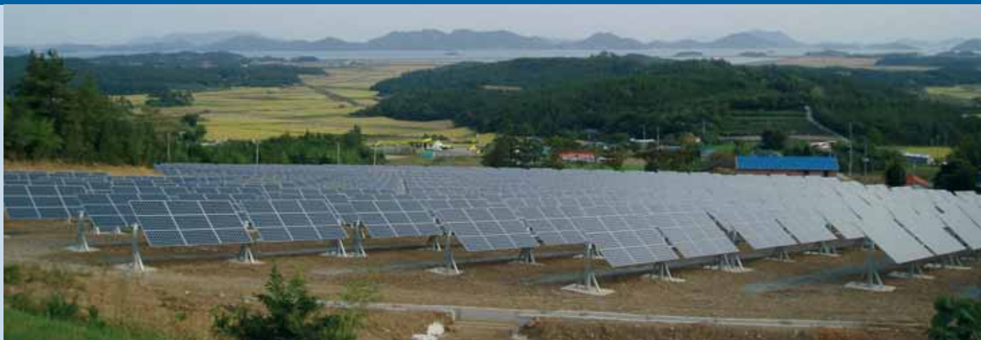
Fig. 1 - 1 MWp PV plant in Kang-Jin located in south west of Korean Peninsula. This plant has a single-axis tracking system with domestic PV modules and four 250 kWp inverters.
