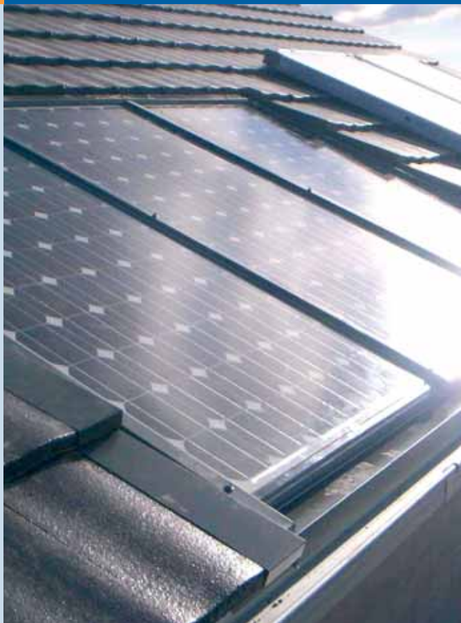
Fig. 3 - Roof integrated PV Solar Tiles at Newington Solar Village. The PV Tiles can be installed with a PV Airflow system which facilitates module cooling and offers space heating in winter (photo PV Solar Energy).
