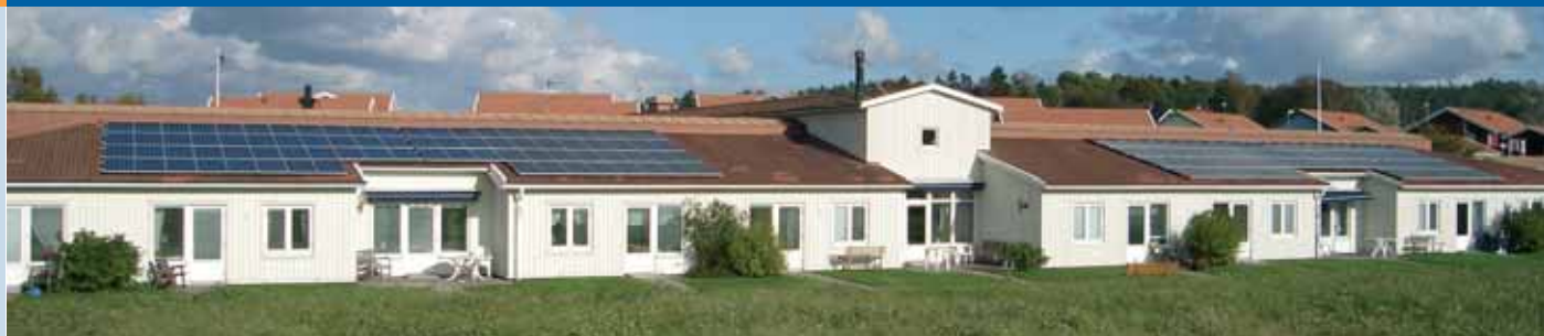
Fig. 3 - A total of 31 kW p split into two identical systems at Solängen retirement home in Gothenburg, Sweden; Project Developer & Source: Switchpower; System Operator: MedicHus/City of Gothenburg (photo Switchpower).
