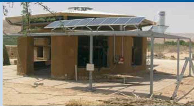
Fig. 3 - 640 W grid-connected system, at Kibbutz Lotan (SolarPower).
