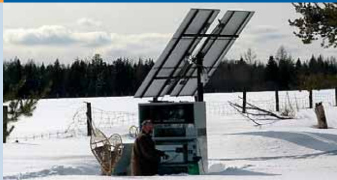
Fig. 3 - Residential 1 kWp PV/6 kVA genset hybrid in New Liskard, ON, Canada (photo courtesy of Xantrex Technology).
