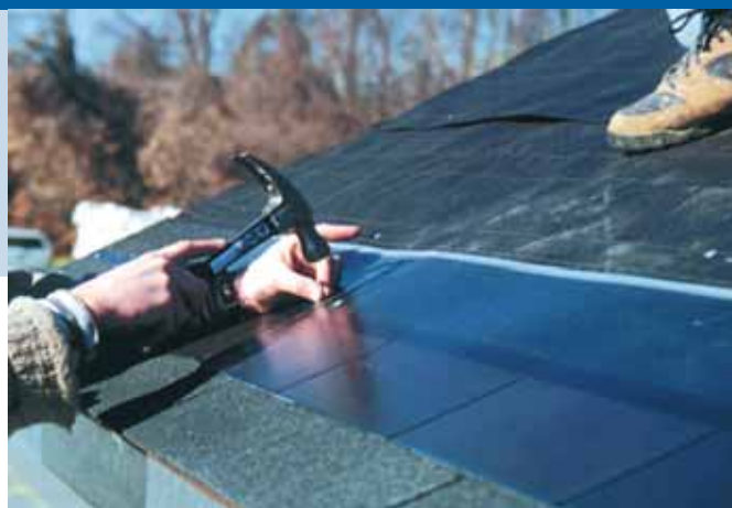
Fig. 3 - PV can be used in many ways to reduce electrical loads created by buildings. These PV shingles, developed with support from the U.S. DOE, can take the place of regular asphalt shingles (photo NREL).
