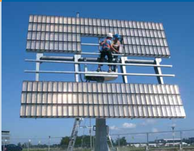
Fig. 2 - Erection of a 5 kW FLATCON®-System (Source: Concentrix Solar GmbH).
