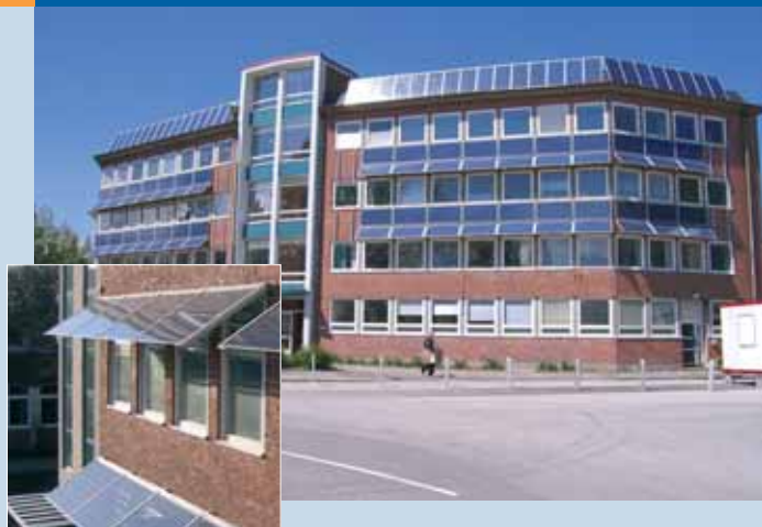
Fig. 2 - PV modules with dual function: electricity generation and solar shading, at the Student Union and the school Mellanhedsskolan (lower left) in Malmö, Sweden. The modules are semi-transparent glass-glass modules of 2x1,5 m (photo Martin Nilsson).
