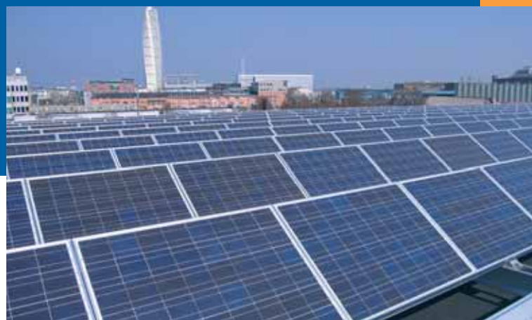
Fig. 1 - The museum of technology in Malmö, Sweden, has a roof top system of 393 m 2 (50,1 kW p ) poly crystalline modules and a facade system of 124 m 2 (17,5 kW p ) mono crystalline modules (photo Martin Nilsson).
