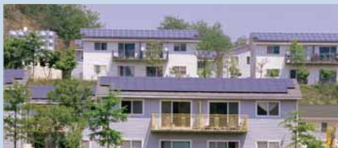
Fig. 4 - Asan green village with a total of 208 kWp grid-connected PV systems for 104 homes.
