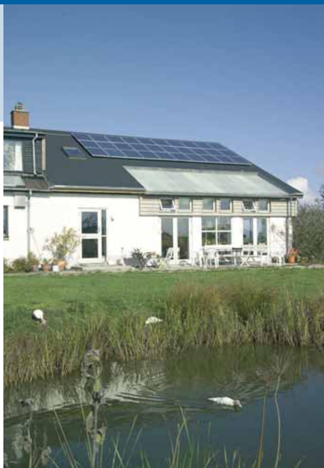
Fig. 2 – PV system from the Danish Sol 1000 with a capacity of 3,15 kWp.
