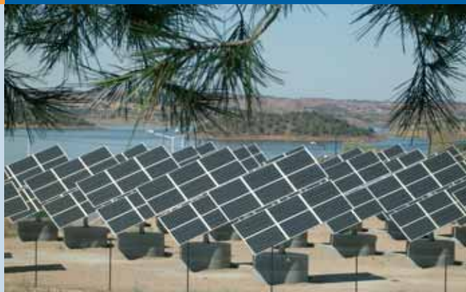
Fig. 2 - 64 kWp one-axis tracking system (Alqueva) (photo courtesy of EDIA, S.A.).
