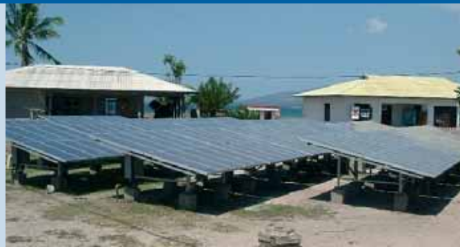
Fig. 4 - Ponelo hybrid system in Indonesia 24 kWp 950 Ah, 240V DC, 125 kVA (photo courtesy of BPPT (Indonesia) / Transénergie (France)).
