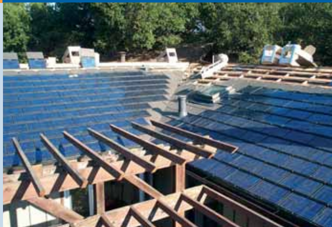
Fig. 4 - These building-integrated PV roof tiles were installed as part of a demonstration project with the City of Palo Alto, California (photo NREL).
