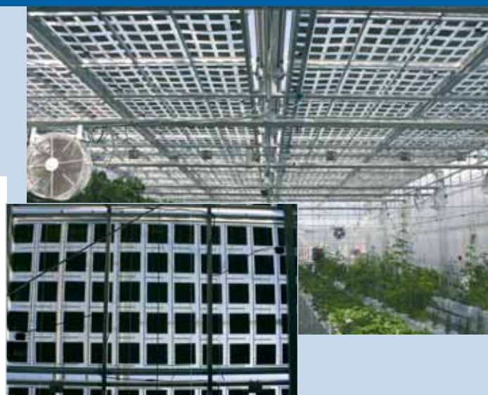
Fig. 2 - PV system at Fujipream agricultural house, 10 kW, Himeji City, Hyogo Prefecture.
