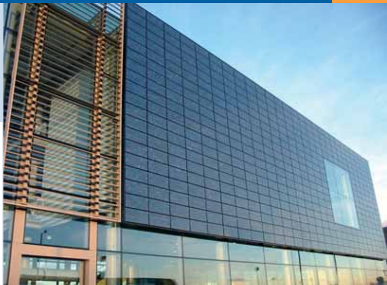
Fig. 2 - PV cladding is part of the new Manchester College of Arts and Technology (MANCAT) building, incorporating pioneering design and building innovation (photo courtesy of solarcentury.com ).
