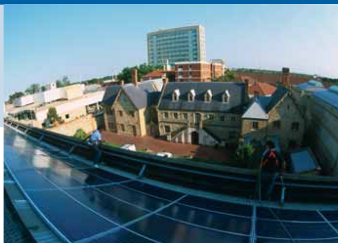
Fig. 2 - Rooftop PV array on South Australian Museum. This is a 19.8 kW PV system, installed by Origin Energy. The panels were manufactured by BP Solar. It is the first installation of the North Terrace Solar Precinct. Solar panels have also been installed on the roofs of Adelaide's Art Gallery, Parliament House and State Library (photo Capital City Committee, a partnership between the South Australian Government and Adelaide City Council).
