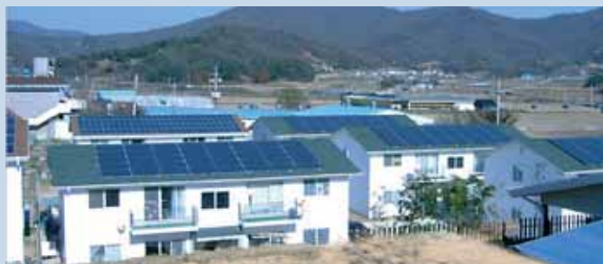
Fig. 3 - A green village in Cheonan City located about 100 km south of Seoul which has 32 2 kWp PV roof-top systems.
