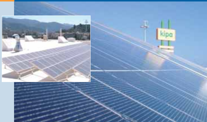
Fig. 6 – 30 kWp grid-connected PV system in Marmaris by Enisolar Ltd.
