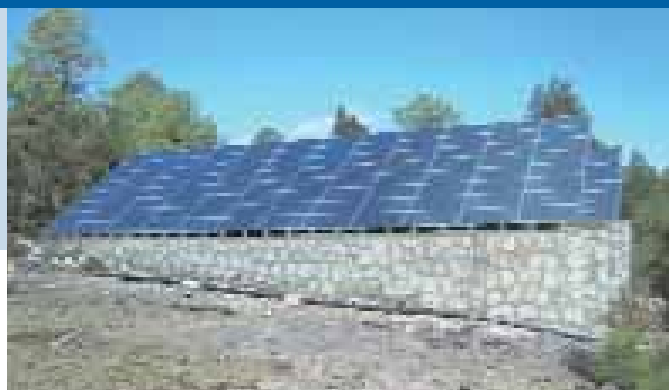
Fig. 2 - 15,2 kW PV array of a water pumping system used for water supply in a rural community in Northern Chihuahua State (photo Conergy Mexico).
