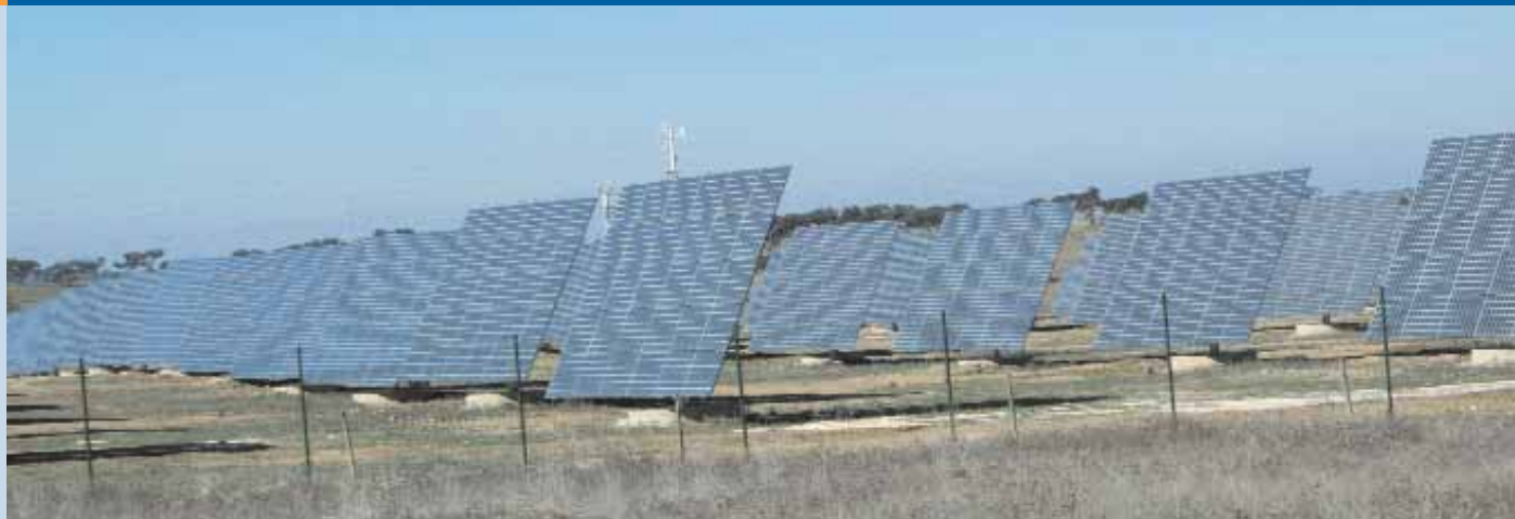
Fig. 2 - PSIA power plant (Almodovar) – 2,15 MWp 2-axis tracking system.
