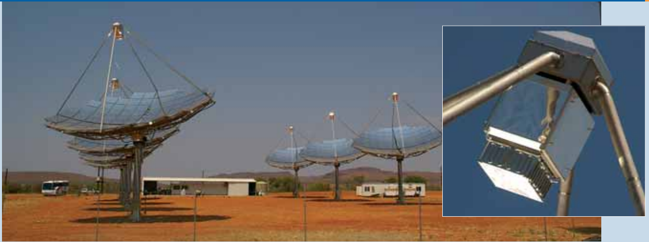
Fig. 2 - Hermannsburg Solar Power Station, part of a diesel mini grid in Central Australia. 8 x 24 kW (192 kW) solar concentrating dishes by Solar Systems Pty Ltd (photo Novolta/W Meike).
