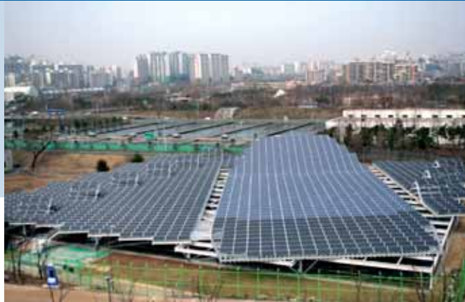
Fig.3 - The 310kW PV power plant installed at water purification sites from Seoul Metropolis in 2007.
