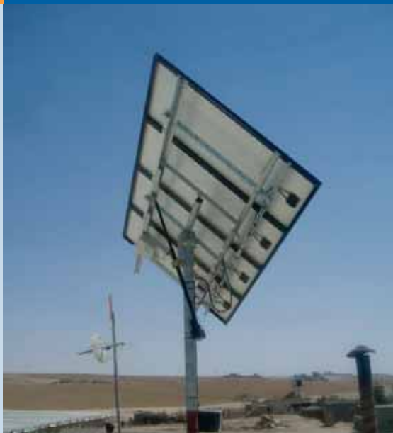
Fig. 4 - 520 W tracking system (photo SolarPower).
