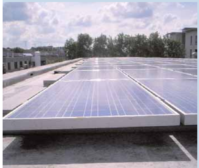
Fig. 3 - 42 kWp flat roof – top PV installation in Groningen, The Netherlands Oskomera.
