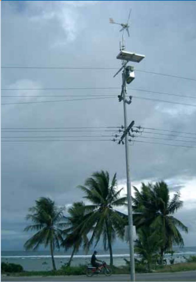
Fig. 9 - Solar-wind powered WIFI repeater grid in Nauru.
