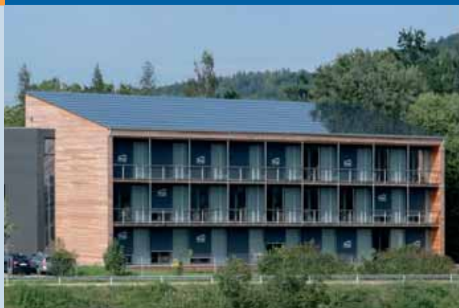
Fig. 2 - Minergie-P-eco office building Marché International in Kemptthal with 45 kWp solar power system (architect: Beat Kämpfen , PV design and engineering: Suntechnics , photo: Suntechnics ).
