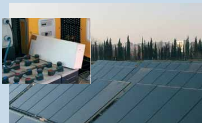
Fig. 8 - HYDEPARK Project in TUBITAK-MRC in Gebze. (12 kWp PV modules, 5 kWp wind turbine, 2,4 kWp PEM type fuel cell, 48 V 1500 Ah battery capacity, inverters, a meteorology station, etc.).
