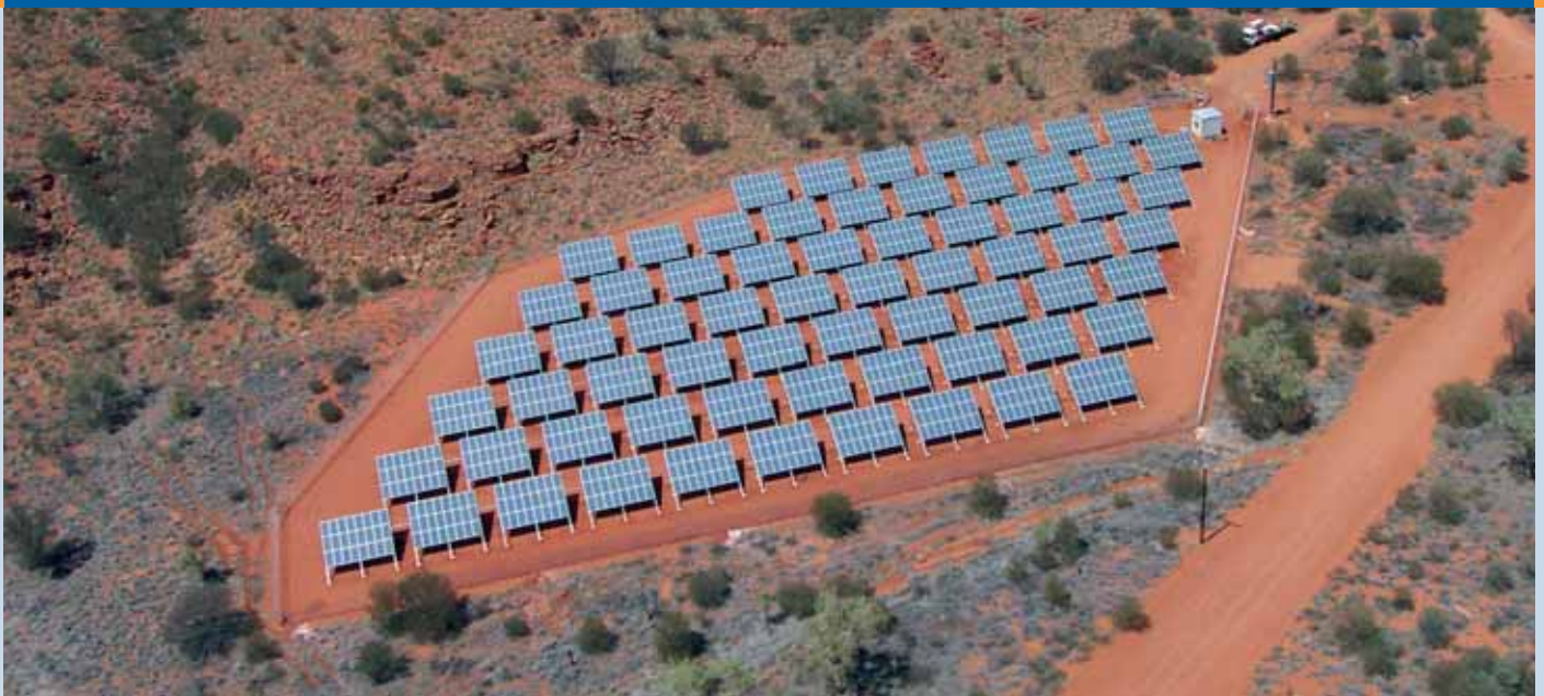
Fig. 4 - 225 kW Kings Canyon Solar Power Station, part of a diesel mini grid in Central Australia. Owned by Power And Water Corporation, the local electric utility. Concept and Design by Wolfgang Meike (photo Novolta/W Meike).
