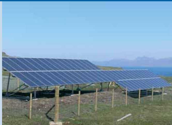
Fig. 3 - This 9,9kW array was installed during 2007 as part of the Isle of Elgg Electrification project (photo Wind and Sun).
