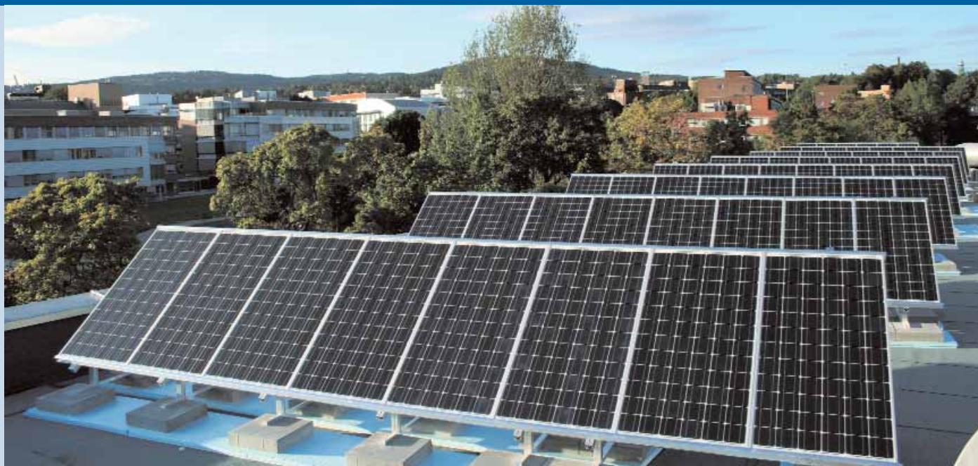
Fig. 1 - The 17,6 kWp installation on the roof of Oslo Innovation Centre in Oslo (photo Norsk Solkraft as).
