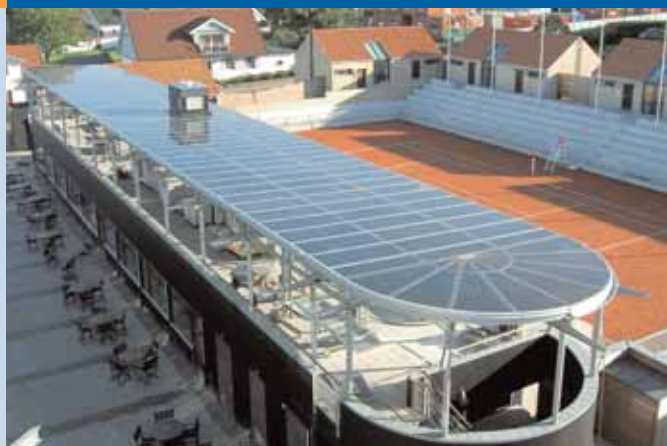
Fig. 3 - In time for the Swedish Open tennis tournament in July 2007; approximately 80 kWp split into two systems, were installed at the Båstad Tennis arena (photo Glacell /Sharp).
