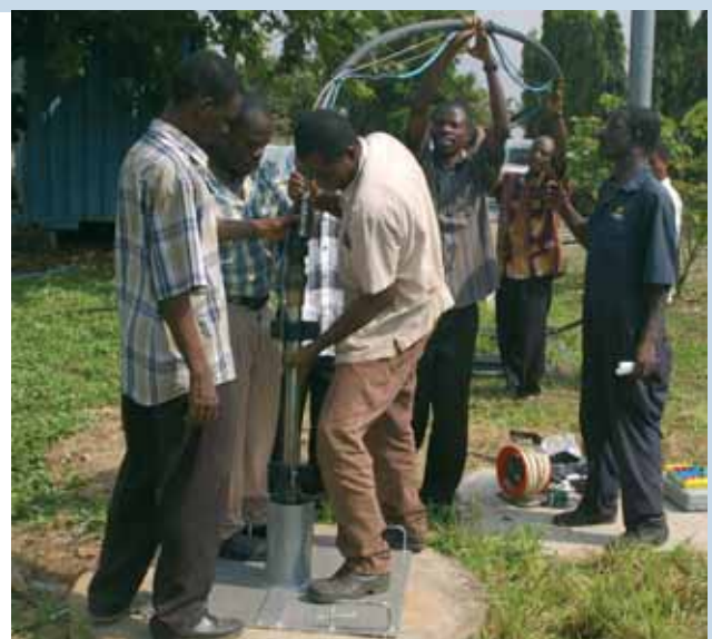
Fig. 6 - Installing a borehole pump as part of a training course by DENG in Ghana.
