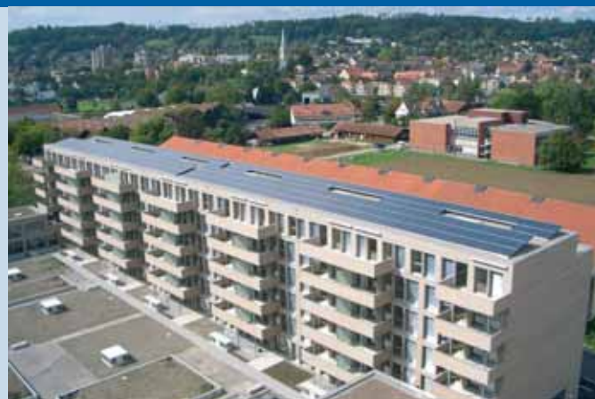
Fig. 3 - Zero energy multifamily buildings Eulachhof in Winterthur with 176 kWp solar power system (PV design and engineering: Amstein & Walther , TRITEC , photo: TRITEC ).
