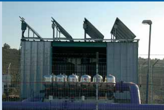
Fig. 3 - 1,5 kW PV system at a large water control station (photo Interdan).
