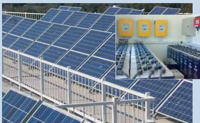
Fig 4 - PV power system in Izmir by Ege University Solar Energy Institute (14 kWp stand-alone and 10 kWp grid-connected PV system).
