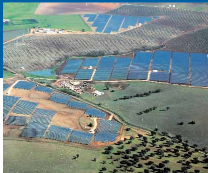
Fig. 1 - Hercules power plant (Serpa) – 11 MWp single-axis tracking system.
