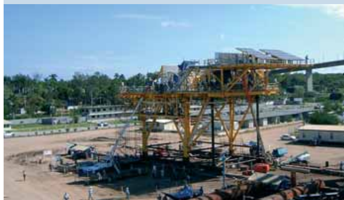
Fig. 3 - 7,5 kW PV to power a SCADA and telecommunication system for a non- manned offshore oil platform (photo: Conergy Mexico).
