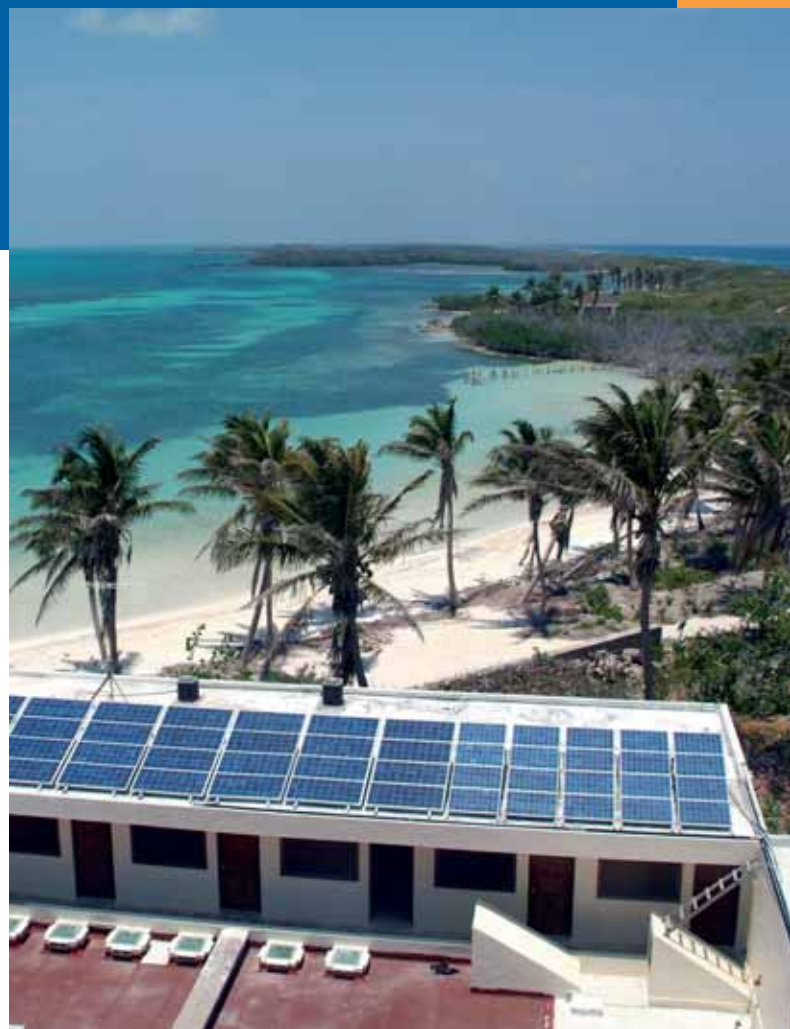
Fig. 1 - 5,6 kW PV array of a PV-Wind-Diesel hybrid system installed at the Biodiversity Reserve on Contoy Island, near Cancun (photo Conergy Mexico).
