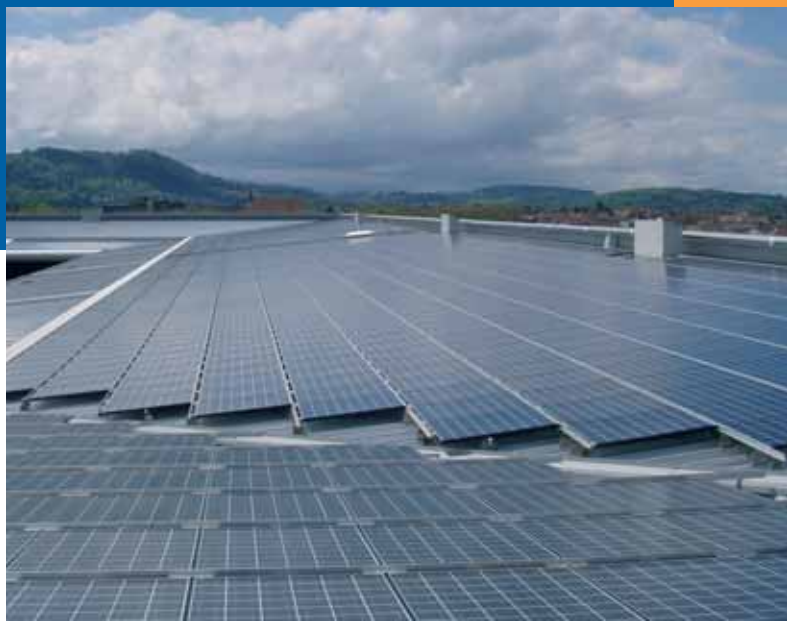
Fig. 1 - Extension of the solar power system on the football stadium Wankdorf in Bern to 1,35 MWp (PV design, engineering and installation: energiebüro®, Ingenieurbüro Hostettler, Minder Energy Consulting, TRITEC; photo: TRITEC).
