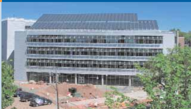
Fig. 2 - Newly installed 108 grid-tie solar power system on the Jean Canfield Government of Canada Building, Charlottetown, PEI (photo Carmanah Technologies Corp.).
