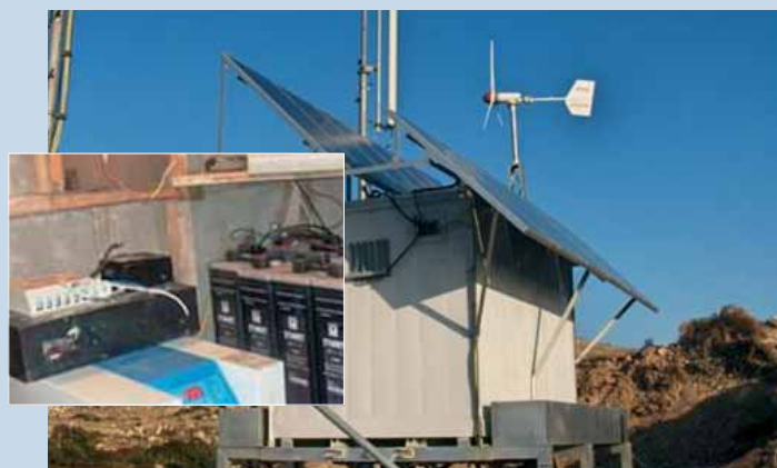
Fig. 9 - A hybrid PV-wind application for telecommunication systems by OZMAK Ltd. in Cesme-Izmir.
