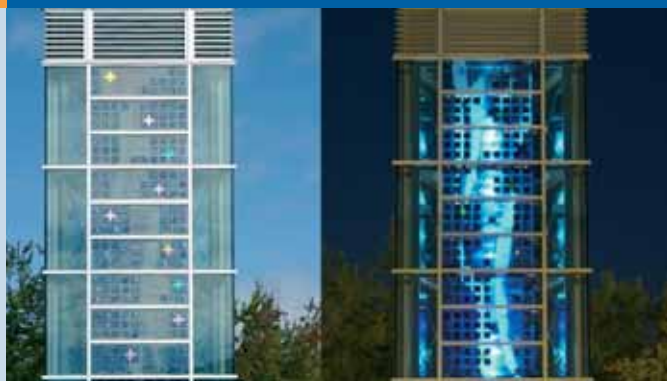
Fig. 3 - Sarah Hall's Lux Nova exhibit of stained glass embedded with solar cells and LED lighting grace the wind tower of Regent College, British Columbia (photos Sarah Hall).
