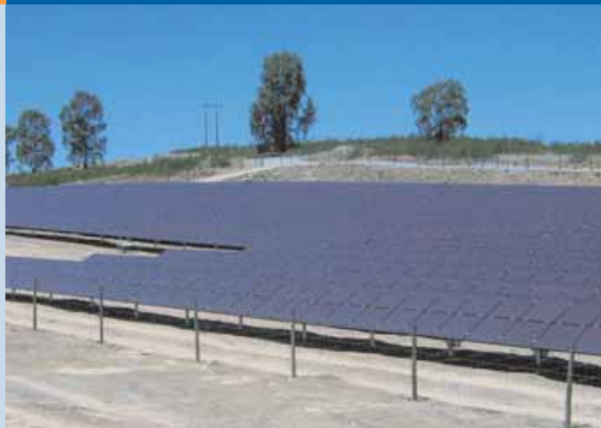
Fig. 3 - Pao e Agua power plant (Mertola) – 756 kWp a-Si system.
