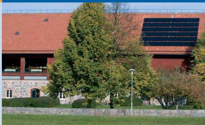
Fig. 3 - The system is the first in Sweden with CIGS modules from Solibro, a company that was founded as a spin-off from thin film research at Uppsala University. The system is installed at the Swedish University of Agricultural Sciences in Uppsala (photo Julio Gonzalez, SLU).
