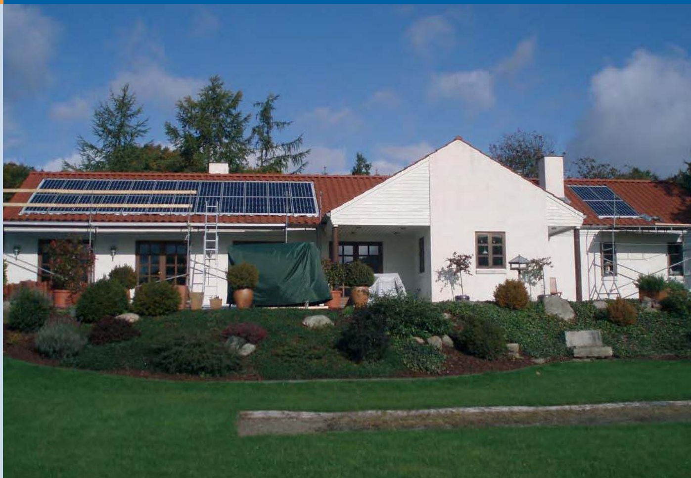
Fig. 2 - The 6 kWp installation supplies free heat through a heat pump and in addition contributes to the other electricity consumption of the building. The mix of a PV system and a heat pump is becoming a popular mix in Denmark despite the lack of governmental support.
