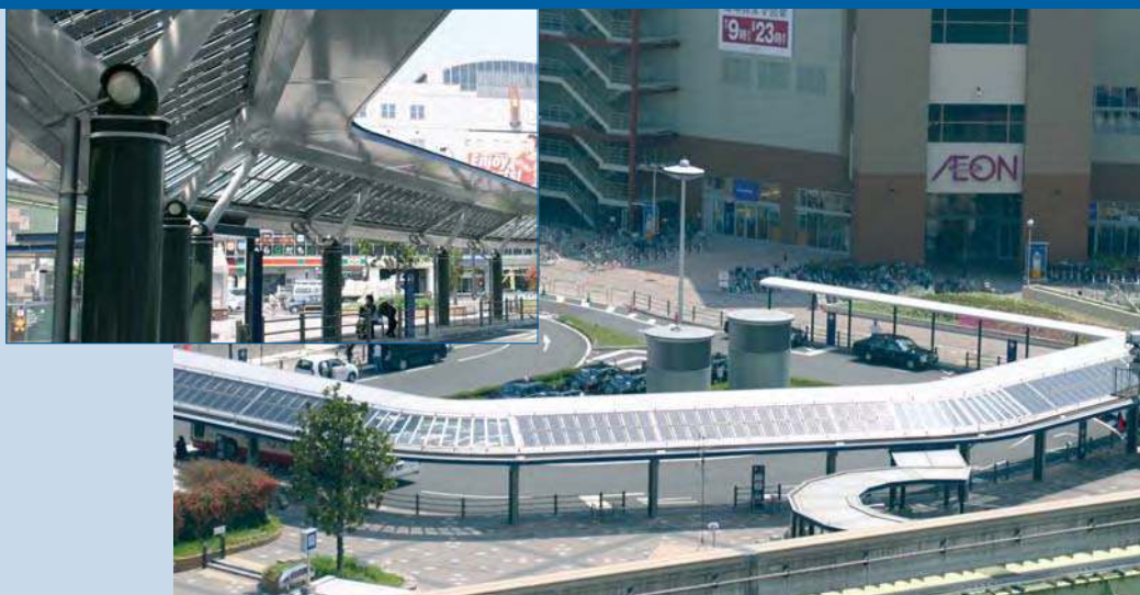
Fig.2 – PV System in front of Osaka Dainichi Station, 11kW (Dainichi Higashi-machi, Moriguchi City, Osaka) (photo RTS Corporation).
