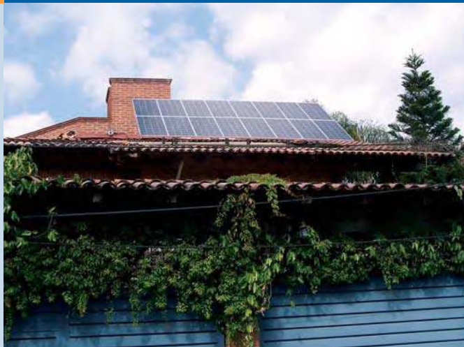
Fig. 2 - 10 kWp Grid Connected System in a house (photo Cryplant).
