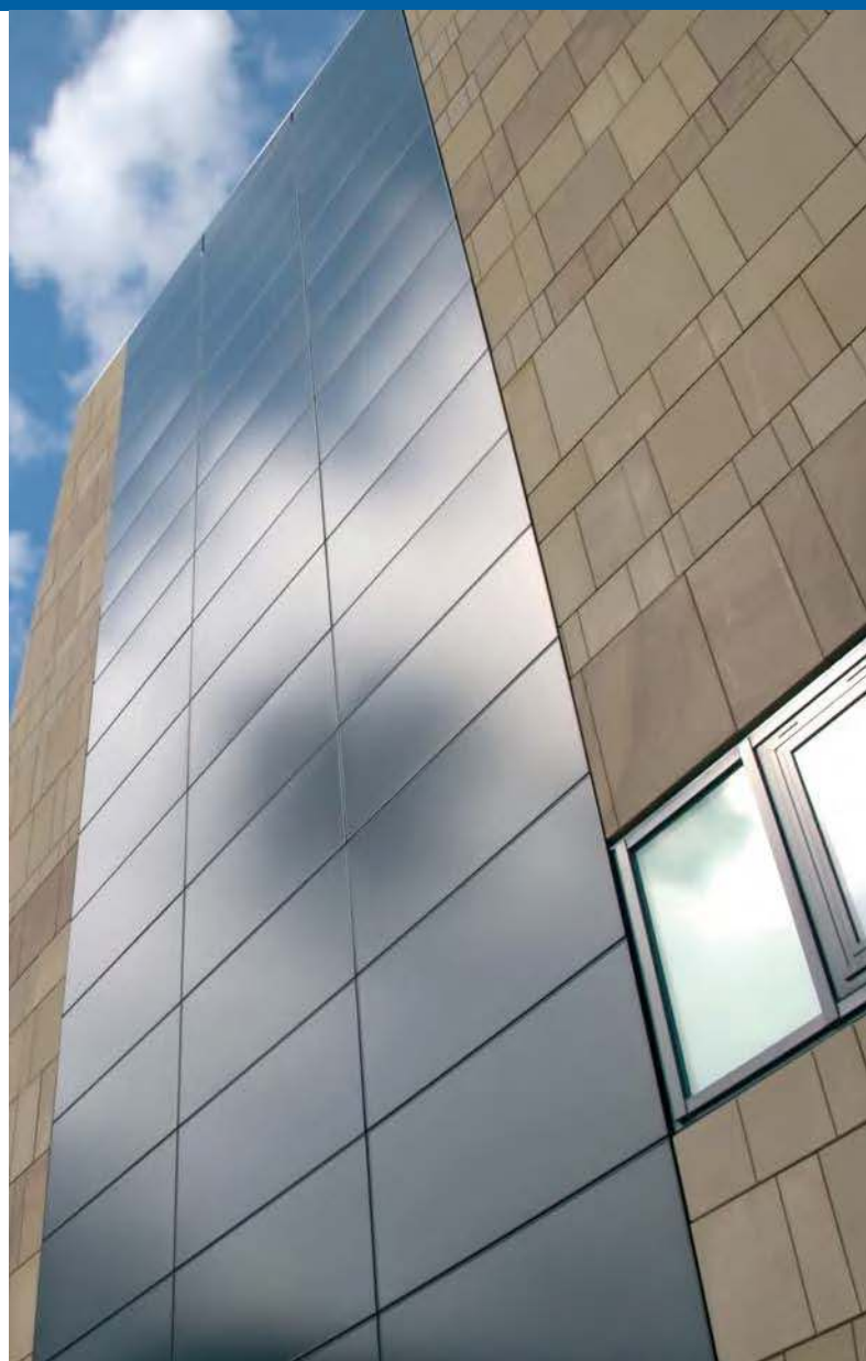
Fig. 1 – 8,4 kWp PV façade at Derby Quad Arts Centre (photo Solarcentury).
