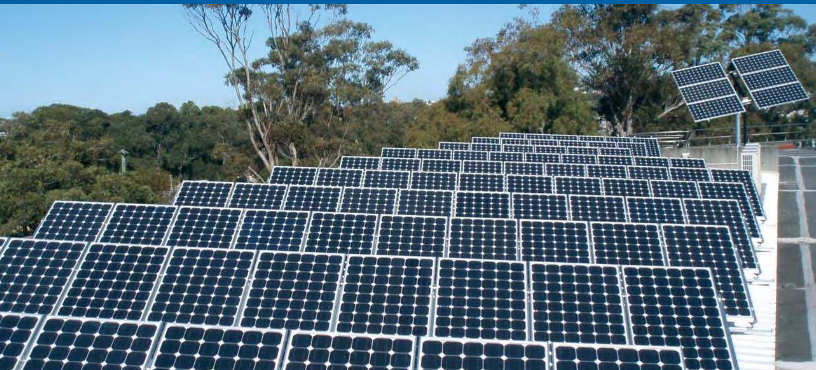
Fig. 1 – Conergy photovoltaic system installed by Solar Newcastle. 17 kW PV system at the Tighes Hill Campus of Newcastle TAFE. Modules: Conergy S175 M. 16 kW is mounted on the Conergy SolarFamulus mounting system, with the remaining 1 kW mounted on the single axis tracker.
