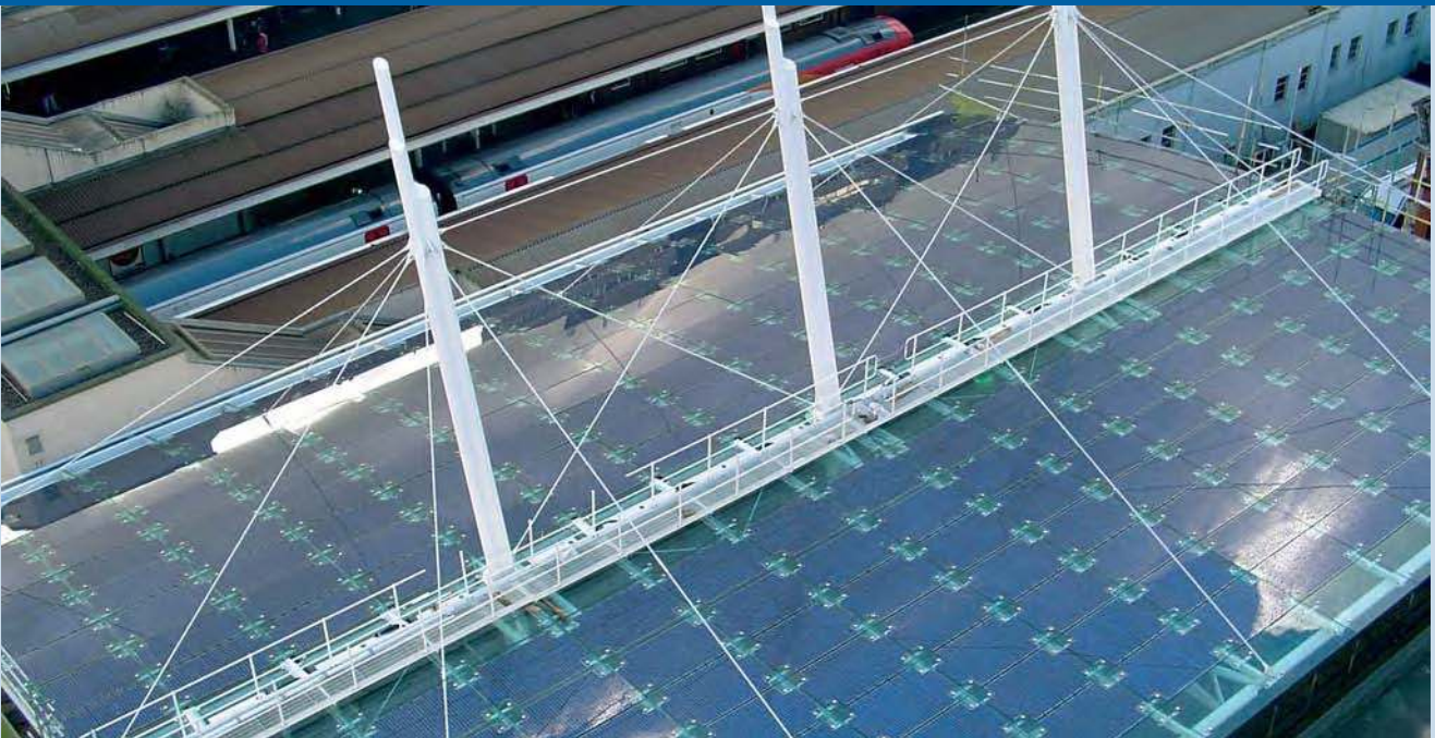
Fig. 2 – 73 kWp PV Canopy at Woking Station (photo PV Systems).
