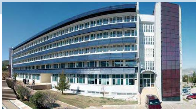
Fig. 3 - 40 kWp BIPV PV power system in Mugla by Mugla University.
