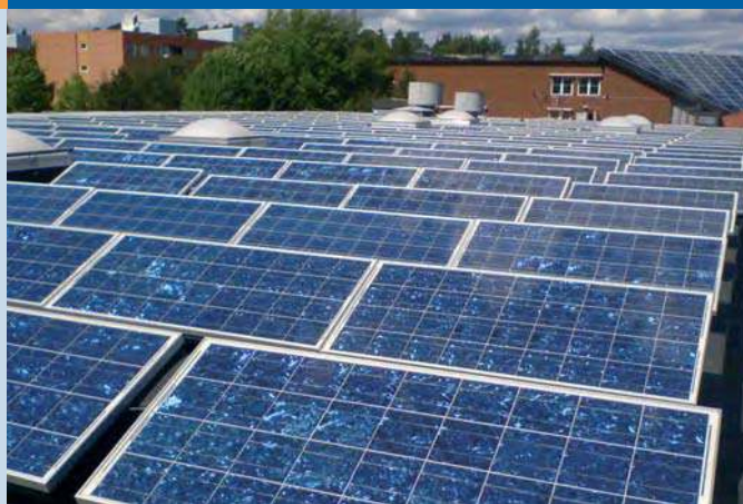
Fig. 2 - 64 kWp PV system on the roof of Andersberg Centrum and on the triangular roof of the nearby Andreas' Church in Gävle (photo Anders Holmsten, Gavlegårdarna).
