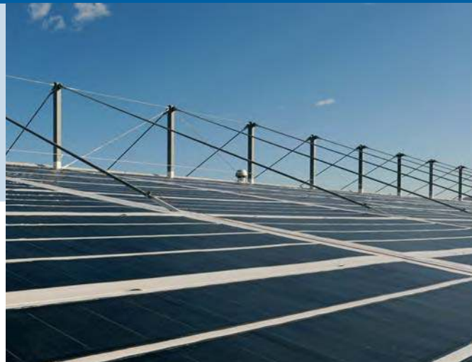
Fig. 2 - Grünendmoos Stadium. Switzerland's largest solar power plant with an installed capacity of 56 kWp made of roofing membrane with integrated thin-film photovoltaic cells. The Grünendmoos Stadium in St.Gallen is the venue of the international CSIO horse riding competition in Switzerland. Surface: 1 200 m². Owner: Sankt Galler Stadtwerke (photo energiebüro, Switzerland).
