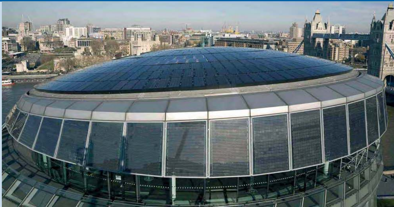
Fig.3 – Intricate design at London City Hall, 67 kWp PV system, Solar Technologies (photo GLA).
