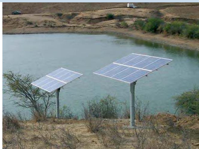
Fig. 4 - Two 0.64 kWp Water pumping systems (photo Cryplant).
