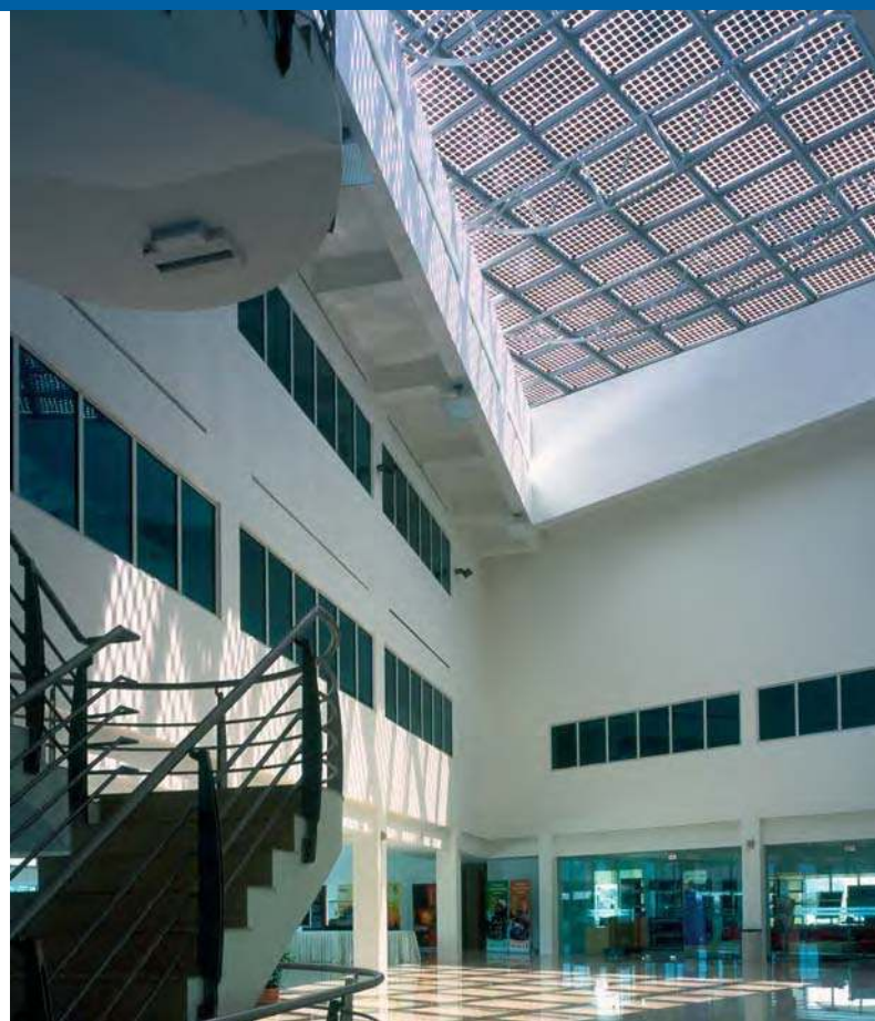
Fig. 1- Semi-transparent BIPV system at atrium of PTM-ZEO building.
