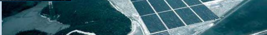
Fig. 3 - Asia's largest PV power plant with capacity of 23,95 MW in Shinan, the southern part of Korea. The systems are operated by horizontal axis tracking mode. It has started commercial operation from November, 2008.
