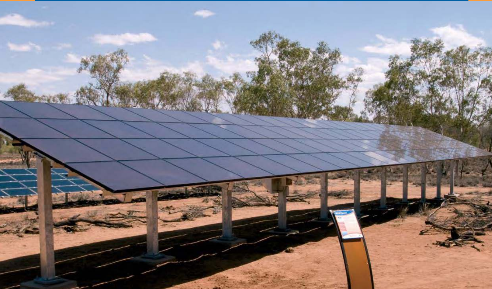
Fig. 2 – Solar arrays at the Desert Springs Solar Test Centre, Alice Springs Kyocera amorphous modules, 1,08 kW each unit, 135 watt panels, 13,5 % efficiency, Wattsun tracker. Five trackers connected to grid through a 5 kW inverter. Behind amorphous array are the CdTe panels (photo Simon Troman).
