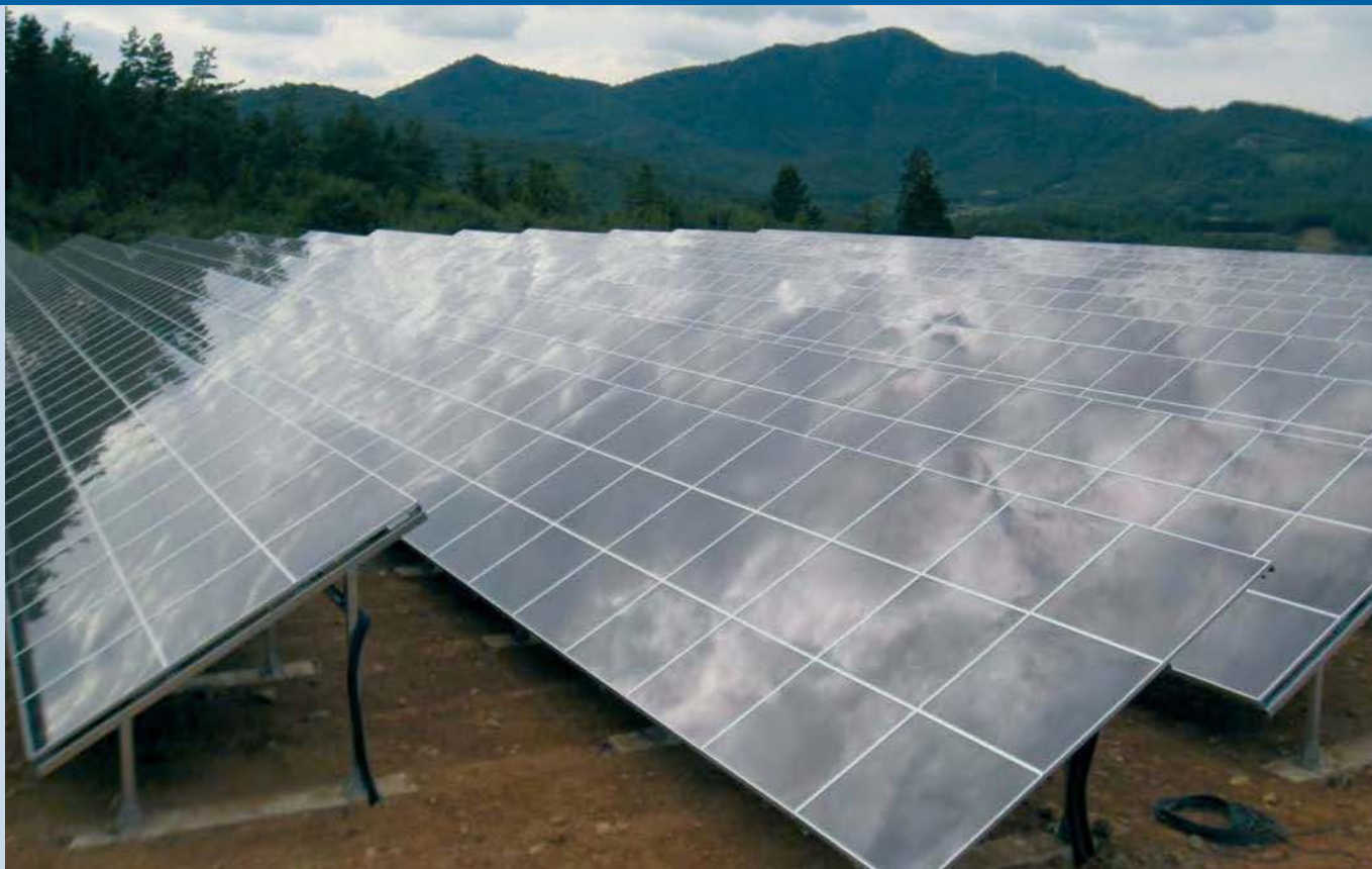
Fig. 1 - The 500 kW a-Si: H modules, produced by KISCO, installed in Haenam, the southern part of Korea.
