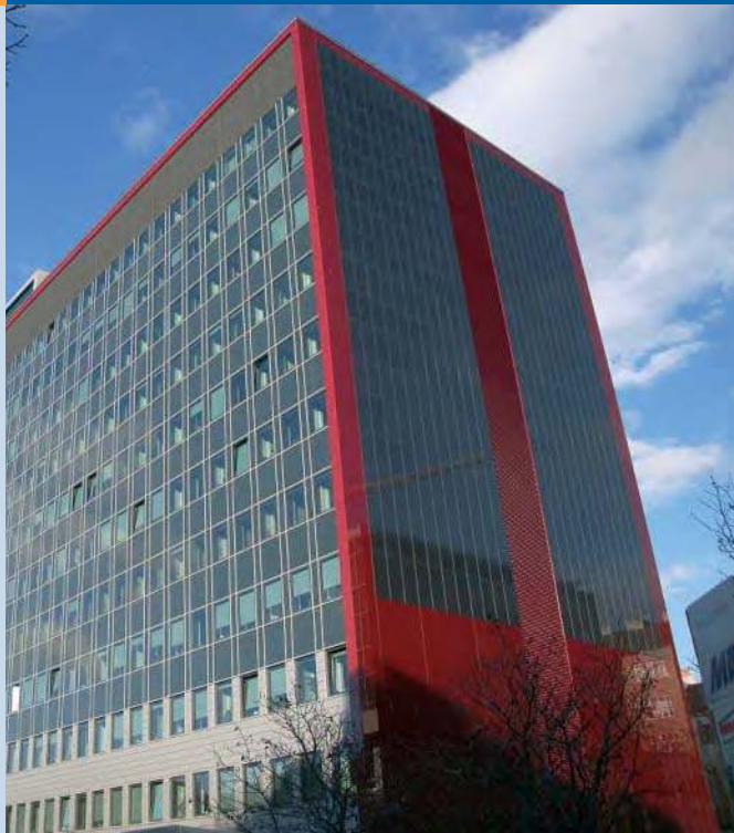
Fig. 2 - Chamber of Commerce, Vienna, 57 kWp PV-System (photo Austrian Chamber of Commerce).
