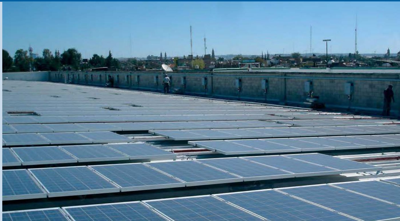
Fig. 1 - 174 kWp PV Grid-Connected system on the roof of a supermarket store (photo Wal-Mart Mexico).
