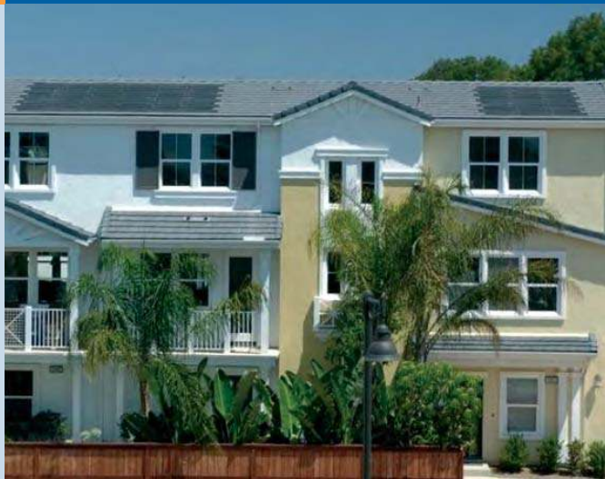
Fig. 5 - Many U.S. homebuilders are using roof-integrated PV systems such as the "solar tiles" shown on the rooftops of this 77-unit solar condo housing development in California. Each system provides owners with about 1 kW of solar energy.
