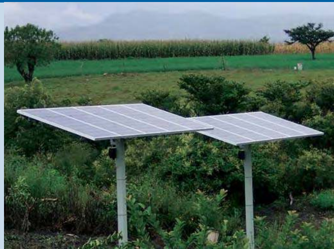
Fig. 3 - Two 0.66 kWp Water pumping systems (photo Cryplant).
