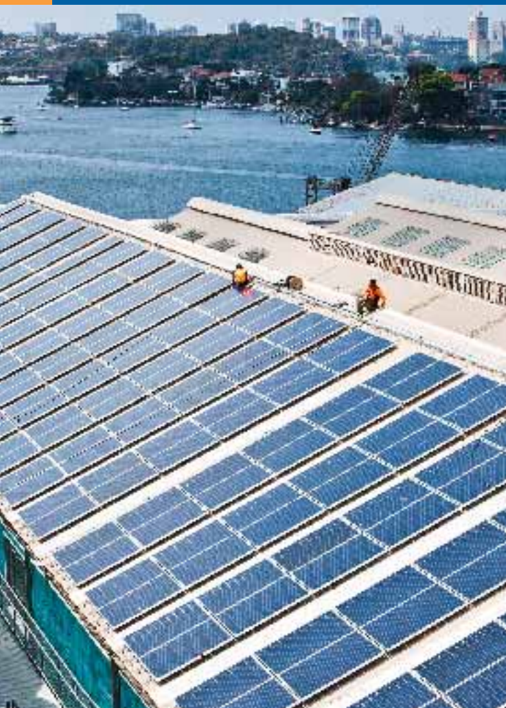
Fig. 2 - 65 kWp PV System on a heritage listed building at Cockatoo Island, NSW, generating 100 MWh/yr (photo: Solgen Energy Pty Ltd).
