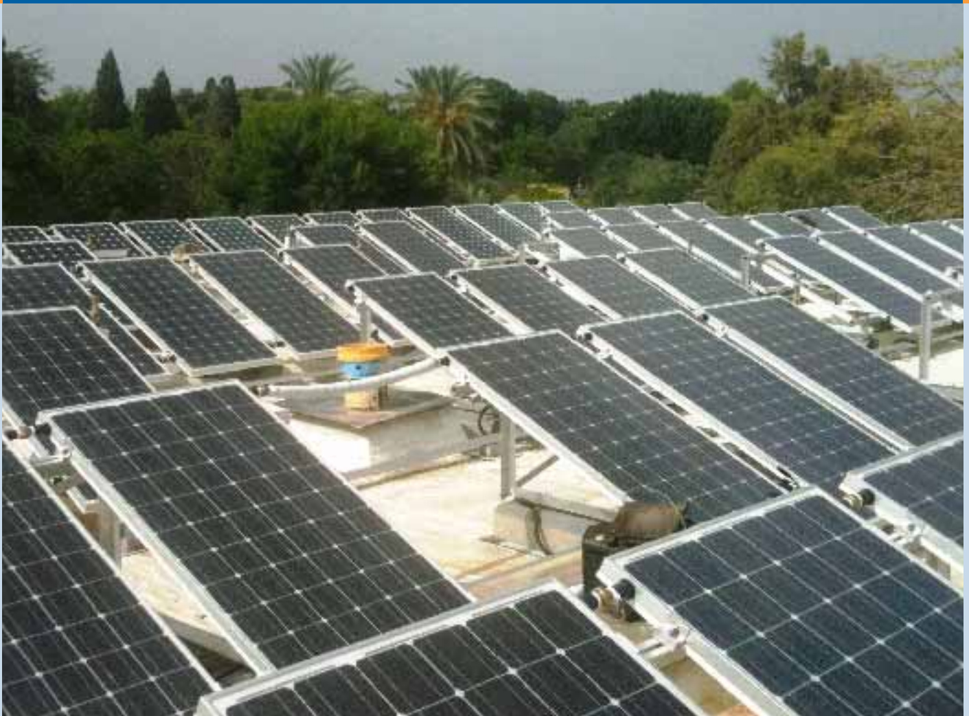
Fig. 7 - PVT plant at kibbutz Yakum, 50 kWp electric and 200 kW thermal (photo: Millennium Electric).
