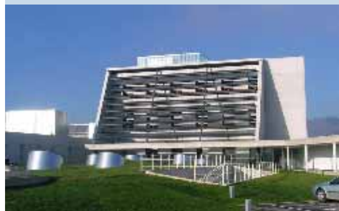
Fig. 8 - PV installation in the façade of CENER building (Sarriena).
