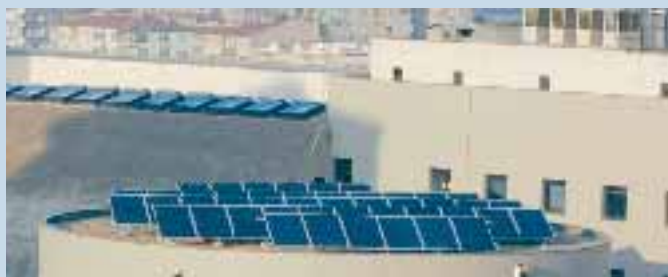
Fig. 4 - 15 kWp grid-connected PVPS by Solimpeks Ltd. at the KCETAS building, Kayseri.
