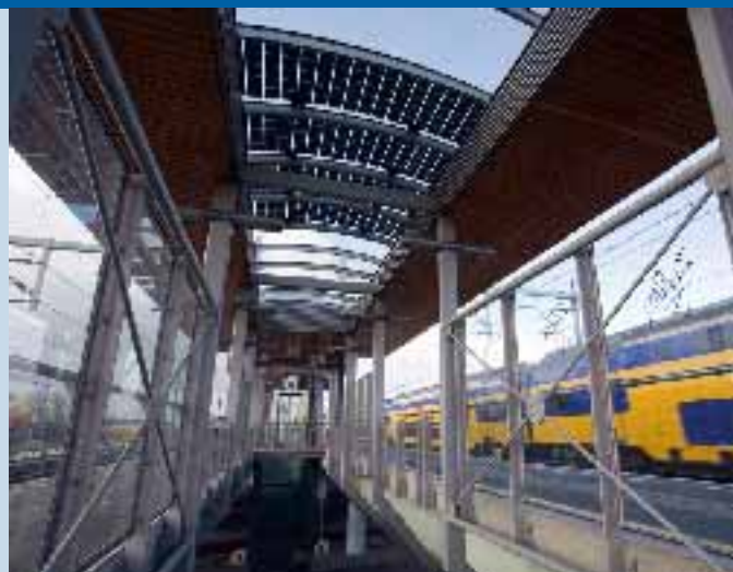
Fig. 1 - PV Cold bended PV modules integrated in roof at the train station Zuilen which is much appreciated by the travellers. Project partners Movares, ECN and BRS Building Systems. This is a SBIR innovation solar program. A study by Ecofys showed that more PV panels along the train tracks would possibly complicate maintenance work and cause longer delays which would not be appreciated by the same travellers.
