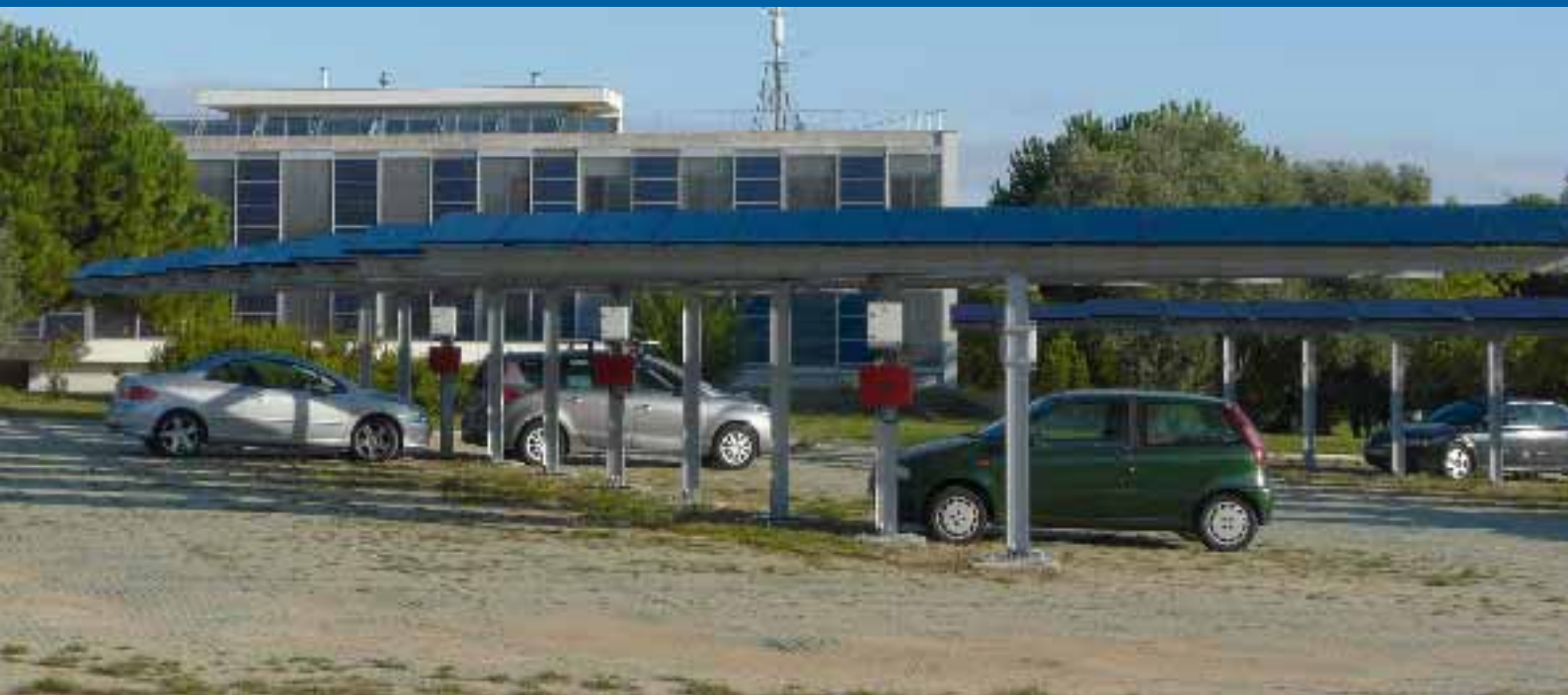
Fig. 1 - 12 kWp CIS array at LNEG parking lot (photo: LNEG).
