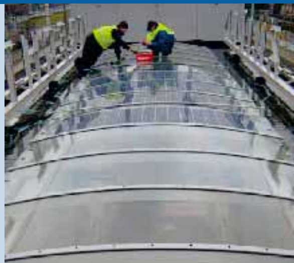
Fig. 2 - Cold bended PV modules at roof train station Zuilen, see also Figure 1. SBIR project partners ECN, Movares and BRS Building Systems. The installation is in process.
