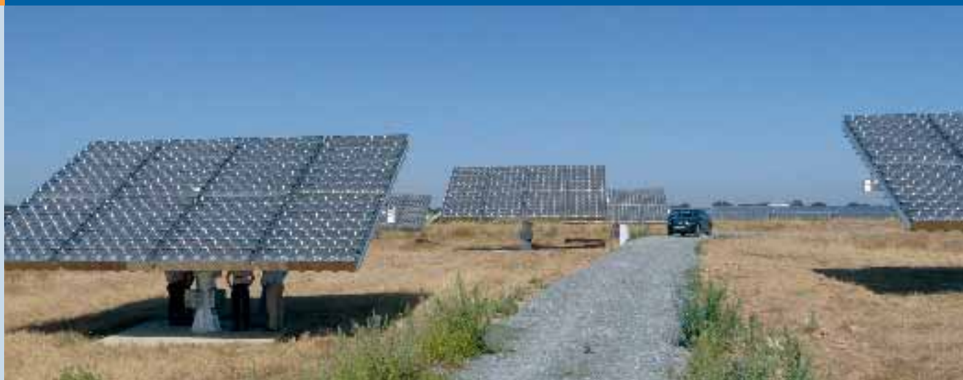
Fig. 2 – 6,6 kWp MagPower CPV – Ferreira do Alentejo (photo: GENERG).
