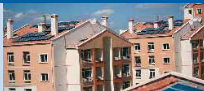
Fig. 5 - 138 kWp PVPS application in TOKI buildings, Kucukcekmece-Istanbul.
