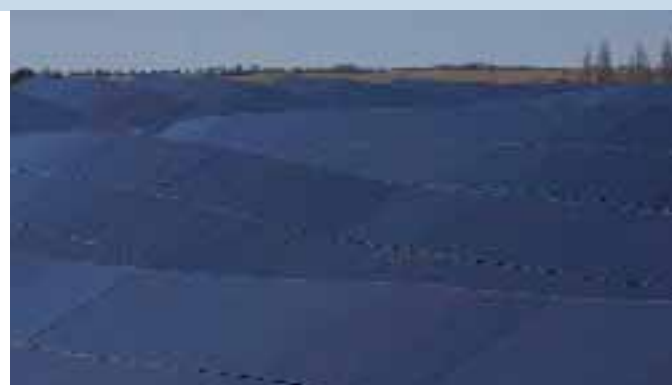
Fig. 6 - 10 MW a-Si PV installation in Saelices (Cuenca) (photo: T-Solar).
