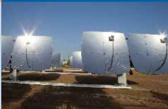
Fig. 3 - ZenithSolar's combined heat and power system at kibbutz Yavne. 32 1000x mirrored dishes generate 64 kWp of electric power plus 160 kW of thermal power in the form of hot water at 75°C.
