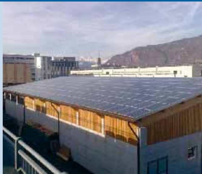
Fig. 3 - Building integrated 65,3 kW PV plant, Bolzano, BZ, Italy (photo: GSE).
