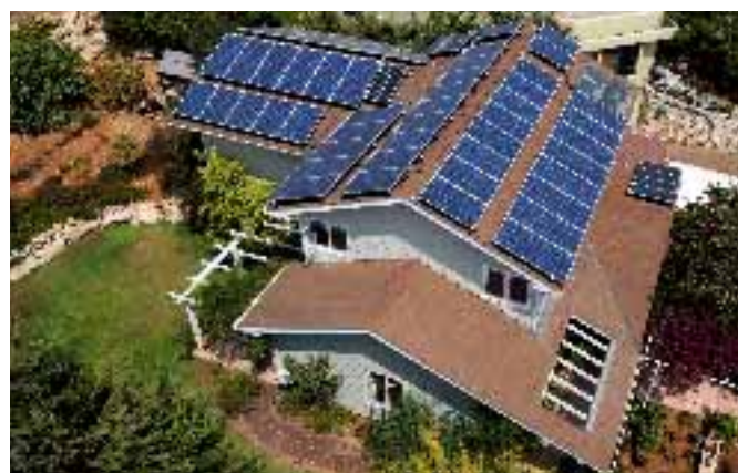
Fig. 6 - A 15 kW p installation on four facets of a roof in Kfar Vradim, enabled by SolarEdge's design flexibility.
