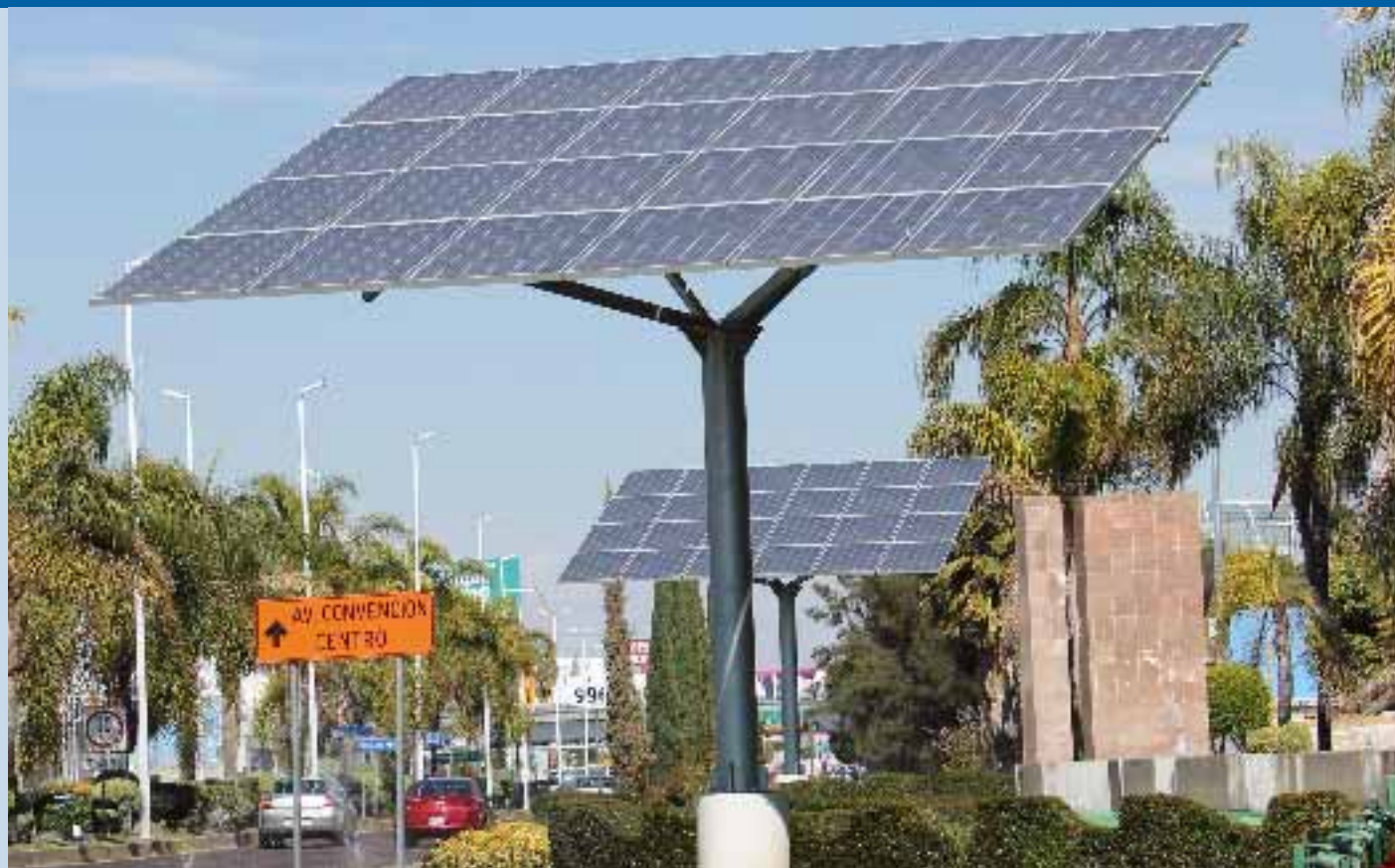
Fig. 1 - PV Grid Connected System for municipal street lighting.
