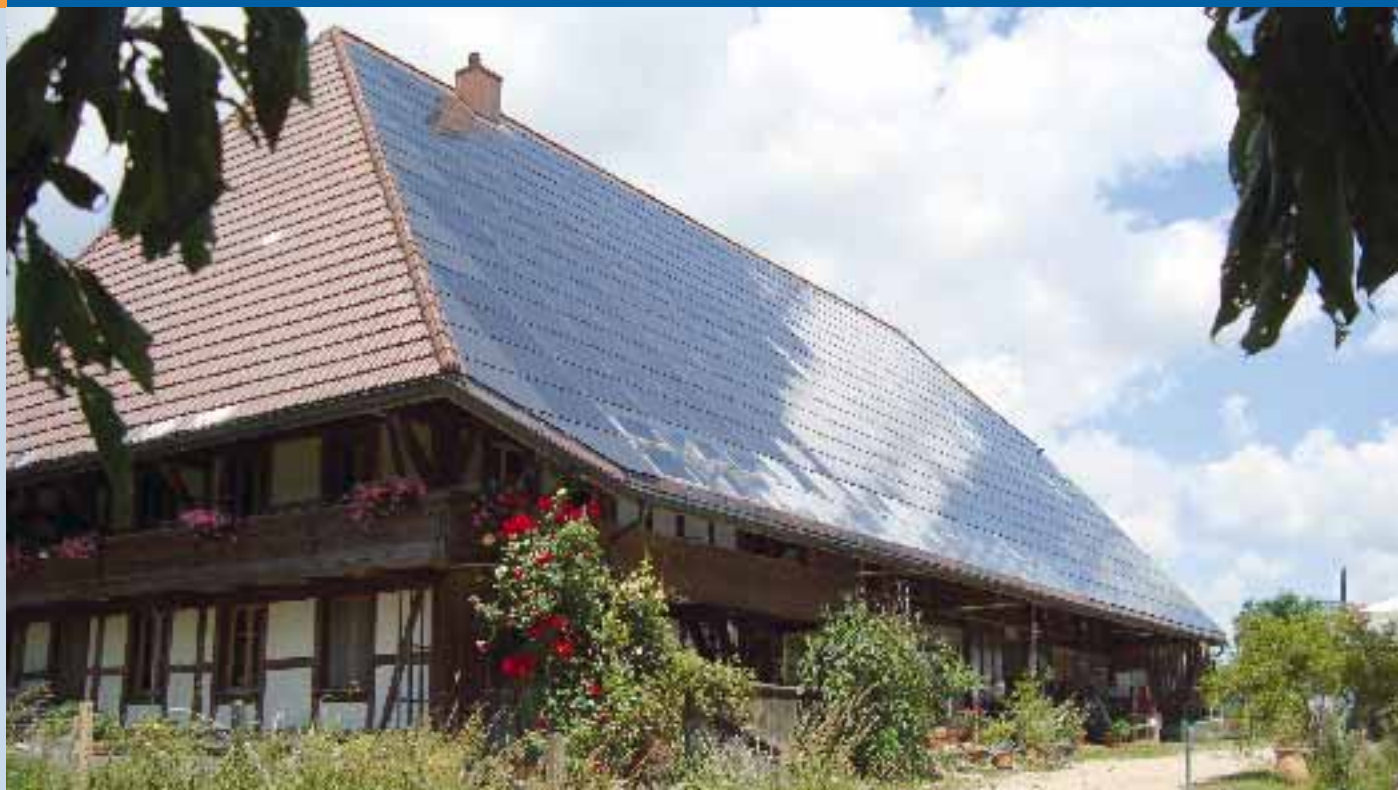
Fig. 4 – Building integrated systems benefit from higher feed-in tariffs and represent 25 % of the systems installed: 46,8 kW system on a farm house in Uettiligen (Berne) (photo: Swiss Federal Office of Energy).
