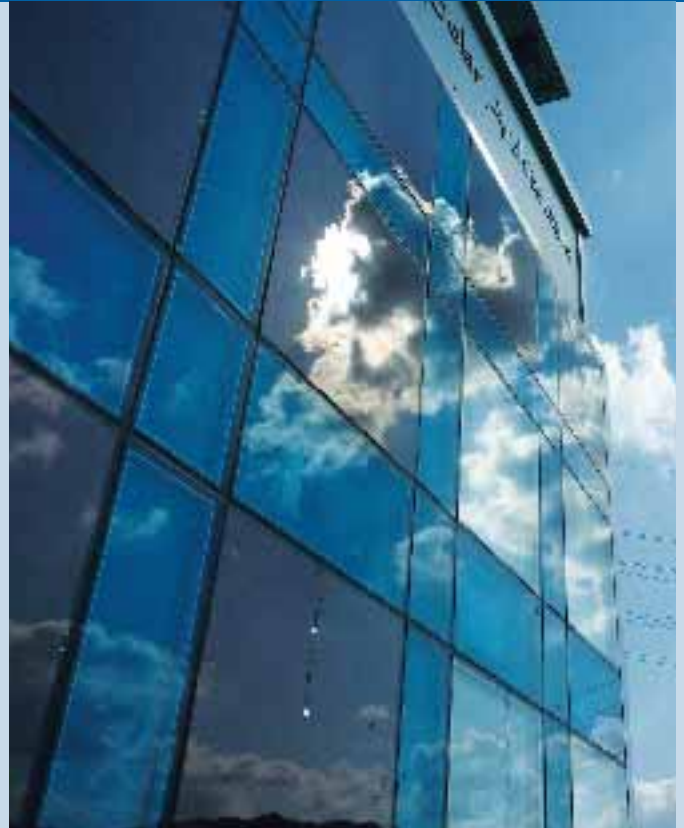
Fig. 2 - SolarCube (2,2 kW BIPV system) at Hanbat National University.
