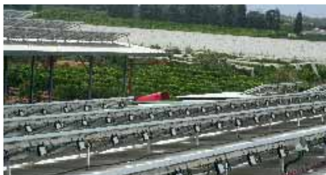
Fig. 5 - A 50 kW p SolarEdge installation on a cowshed in Kfar Vitkin; PowerBoxes are attached to each of the solar modules, for energy maximization.
