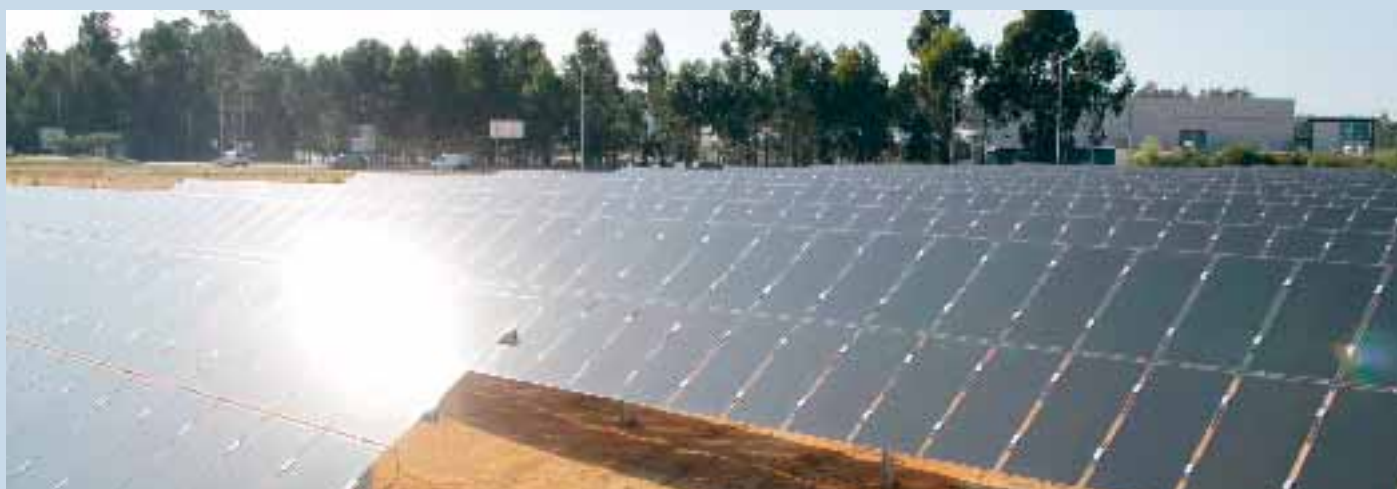
Fig. 3 – 82 kWp a-Si PV System – Oliveira do Bairro (photo: courtesy SolarPlus).
