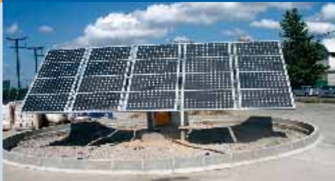
Fig. 7 - 3 kWp Solar Tracking PVPS application in the garden of Kocaeli Metropolitan Municipality.
