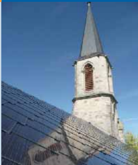
Fig. 5 - PV System integrated to the roof of a church (Alsace department) - 43 kW (photo: Saint Gobain Solar).
