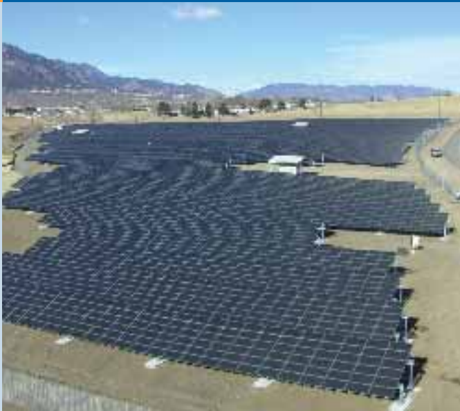
Fig. 2 - WAPA: Western Area Power Authority (WAPA) – new, 2-megawatt, ground mounted solar photovoltaic array occupies the site of a former landfill at Ft. Carson, Colorado. Covering 12 acres, the system will generate 3,200 megawatt-hours of power annually, according to the Department of Energy, or enough to power the equivalent of 540 Fort Carson homes per year.
