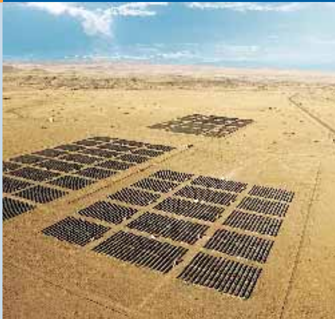
Fig. 4 - 4.6 MW of solar at the Springerville Generating Station Solar System (SGSSS) in northeastern Arizona by Tucson Electric Power. This site generates enough electricity to power about 700 homes. Total array coverage area is 44 acres with 34,980 panels.
