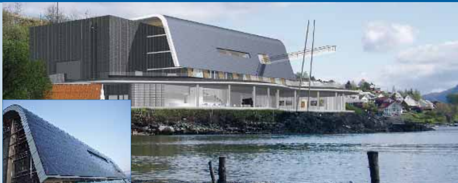
Fig 1. - Oseana: To be finished spring 2011. The building has the largest BIPV system (60 kWp) in Norway so far. The curved wall-roof construction will be covered with PV modules.
