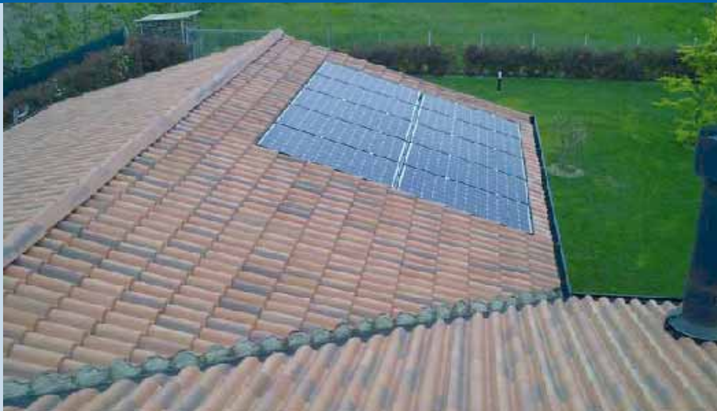
Fig. 1 – Building integrated 2,14 kW PV plant, Villa Bartolomea, Verona, Italy (photo: GSE).
