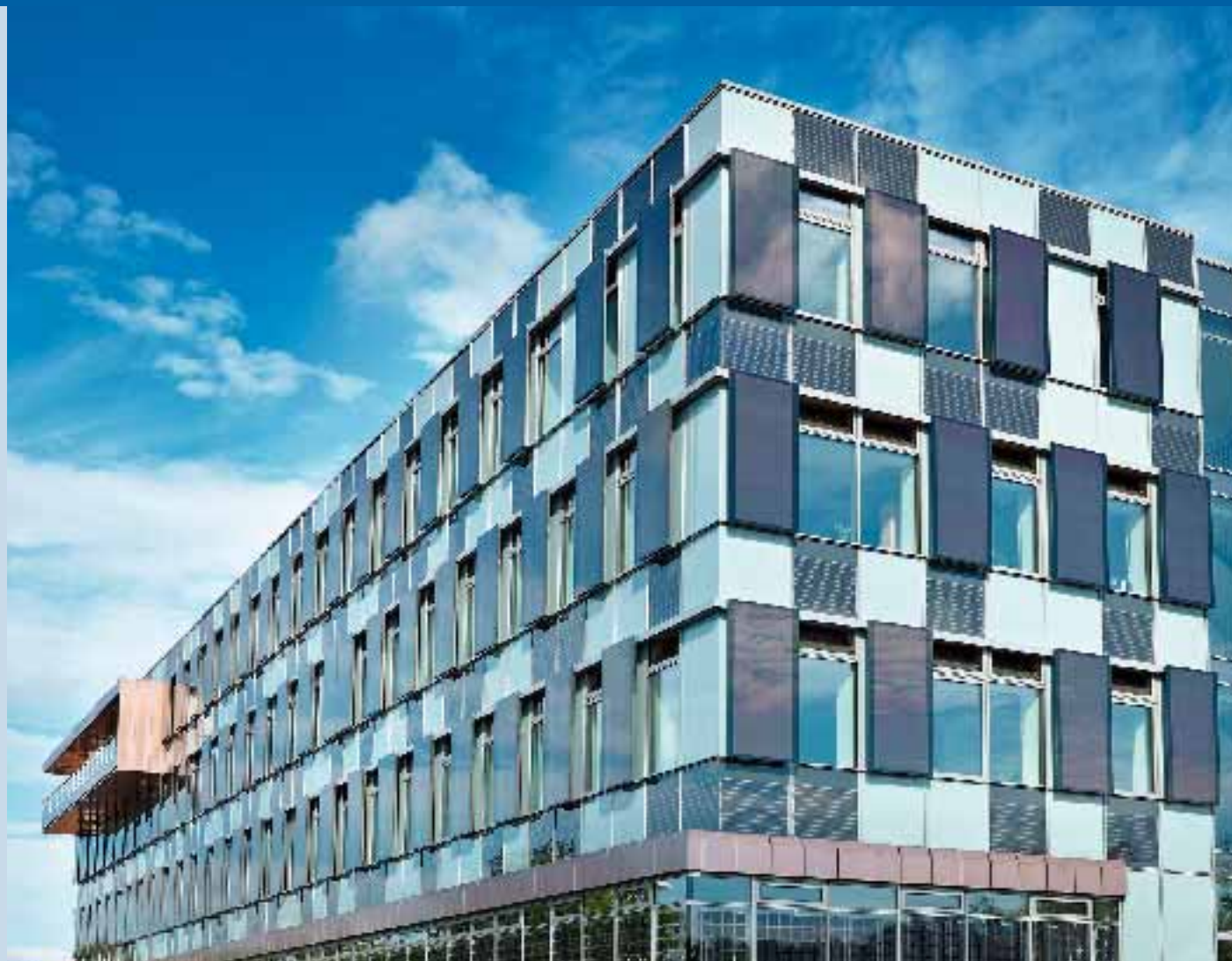
Fig. 1 - New office building at EnergiMidt, Silkeborg, is supplied with 55,5 kWp PV systems. A part of the PV system is constructed as a moveable sunshade with transparent thin film panels. The panels can be controlled individually or automatically. The building is designed as energy class 1 with an estimated total consumption of 27 kWh/m 2 /year.
