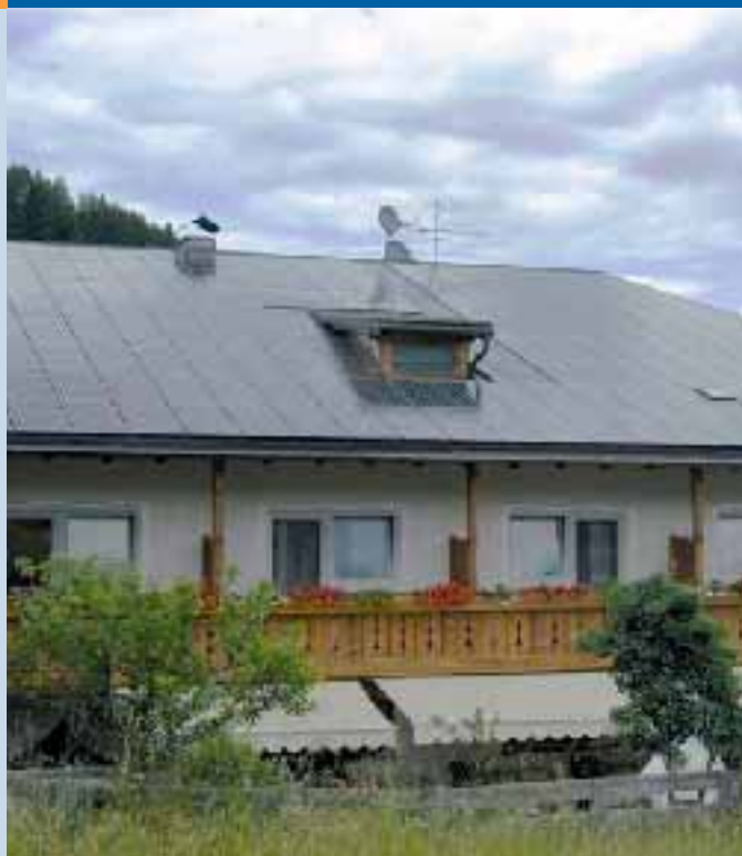
Fig. 4 - Building integrated 33,8 kW PV plant, Bolzano, BZ, Italy (photo: GSE).
