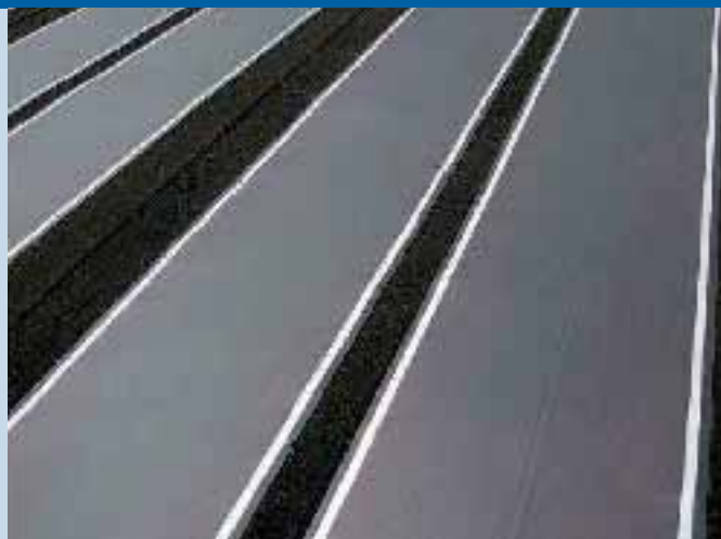
Fig. 6 - HELICO project combining thin film and roof materials for a watertight fit. Project partners Helianthos and ICOPAL. A demonstration project involves IKEA.
