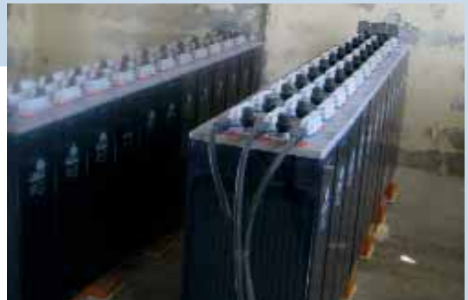
Fig. 1 – A battery bank for a hybrid power plant in Felir, Senegal (photo: IED 2010).
