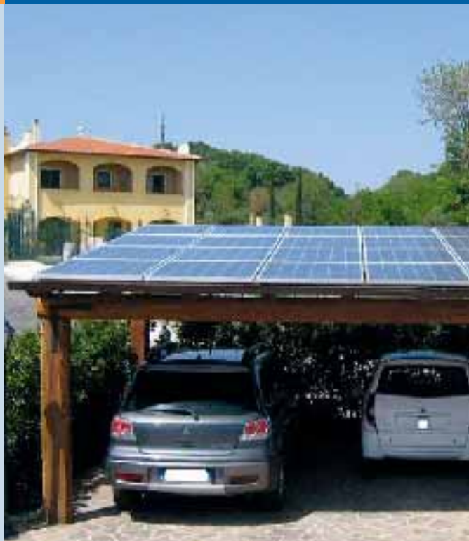
Fig. 2 - Building integrated 6,72 kW PV plant, Formello, Rome, Italy (photo: GSE).
