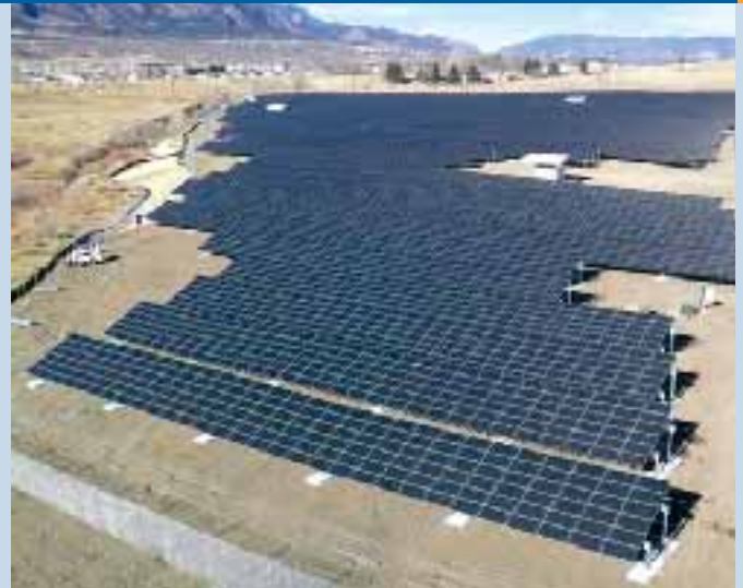
Fig. 3 – 2 MW PV system at U.S. Army Fort Carson, NREL Photographic Information Exchange (photo: NREL).
