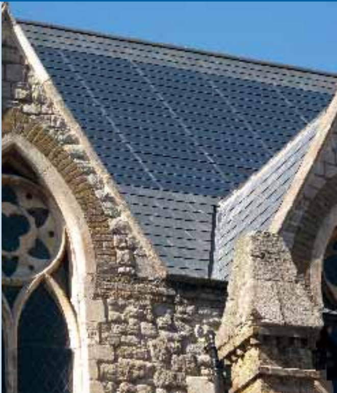
Fig. 1 – 14,84 kWp, St. Silas Church, London by Solar Technologies Ltd.
