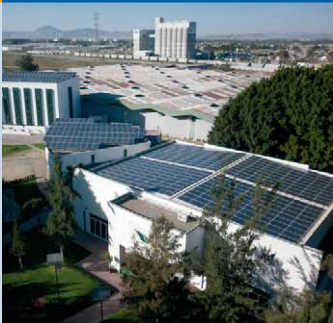
Fig. 3 - 145 kW Roof Mounted PV system (Photo: ERDM).
