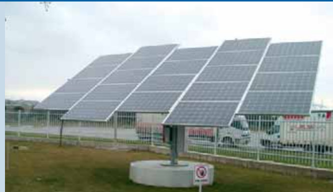
Fig. 4 - 10 kW grid-connected/dual axis tracker PV system by Enisolar Ltd. in the Bosch Factory, Bursa.
