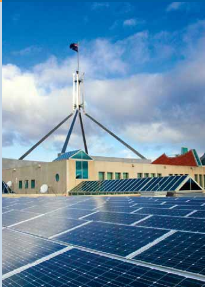
Fig. 2 - 43 kW PV array on the Australian Parliament House, Canberra using Silix Solar PV panels installed by Todae Solar (Photo: Todae Solar).
