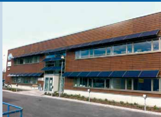
Fig. 4 - The bus depot in Gubbängen has solar cells on the façade as well as on the roof (Photo: Energibanken).
