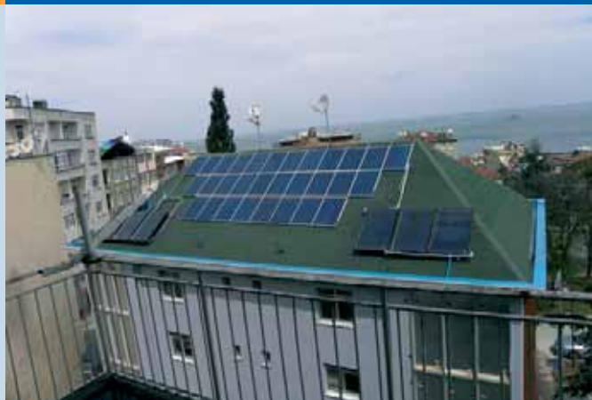
Fig. 5 - 6 kW grid-connected PV system by Motif Proje Ltd. in Samsun.
