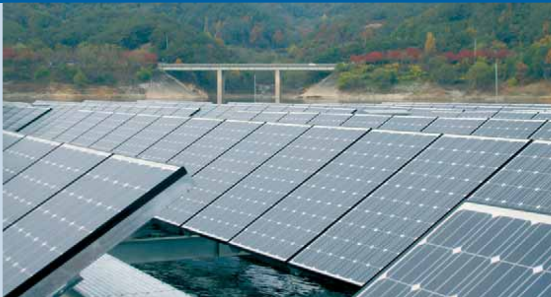
Fig. 1 – 100 kW PV power plant on the water surface at Hapcheon Dam, South Gyeongsang Province.
