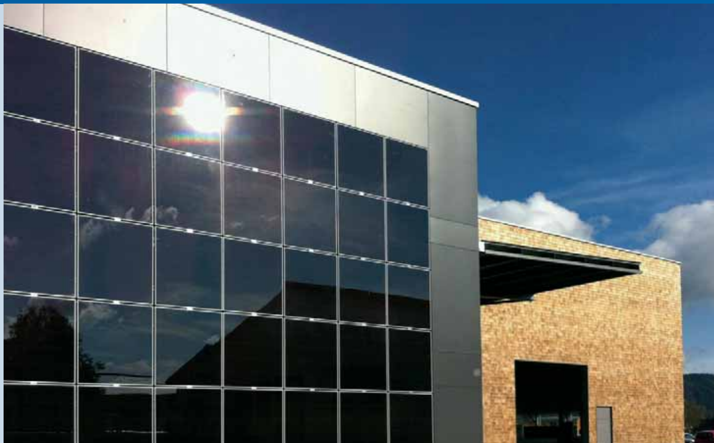
Fig. 1 – 5 kWp PV Façade System. Schötz, Lucerne (photo: Solventure GmbH).
