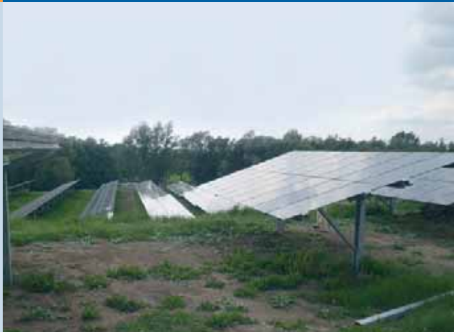
Fig. 3 - Solar Park Azewijn (1,620,000 KWh/year) by project developer Pfixx, on top of a former waste dump.
