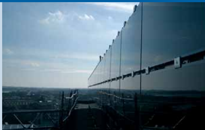
Fig. 4 - Skive Raadhus: CdTe modules used for visual covering of ventilation equipment on the roof of the city hall in Skive.
