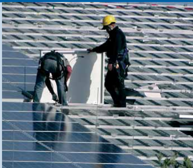
Fig. 1 - Close up installation of nominal DC output 264,74 kWp, Yingli panels, at the district building of the water board Velt & Vecht in Sleen; Project Developer DEC (Photo: Ecofys).
