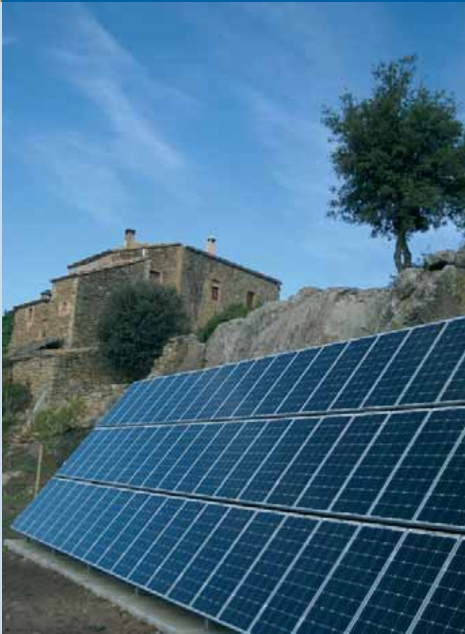
Fig. 2 – Remote hamlet near Manresa (Spain). Three households. Aggregate demand: 12 kWh/day. Solar fraction: 95 %. PV generator capacity (STC): 5760 Wp. Battery Rated Capacity: 72 kWh. Battery Charge controller: 2 X 60A (MPPT). Inverter Capacity: 2 X 3500 VA. Electricity Dispensers: 3 (Photo: TTA (Trama Tecno Ambiental)).
