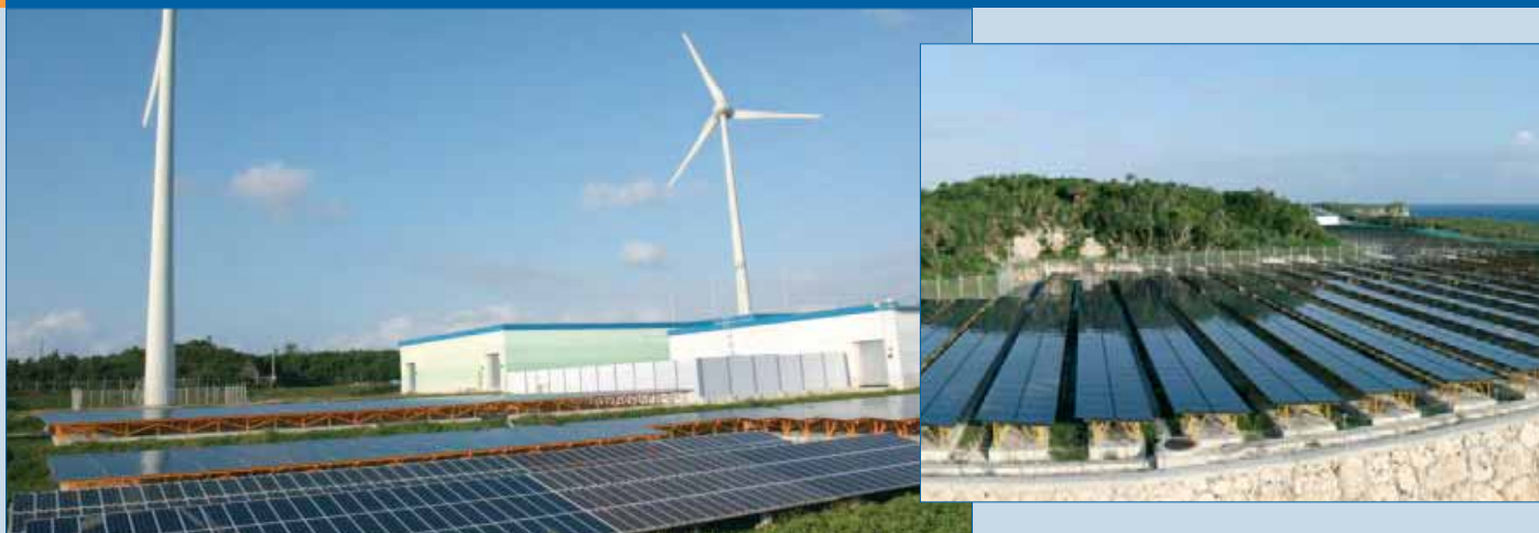
Fig. 4 - Miyako Island Large-Scale Solar Demonstration Research Facility Miyakojima City, Okinawa Prefecture Total 4 MW. Microcrystalline thin-film silicon PV module (by Kaneka). Multicrystalline silicon PV module (by Sharp, Kyocera).
