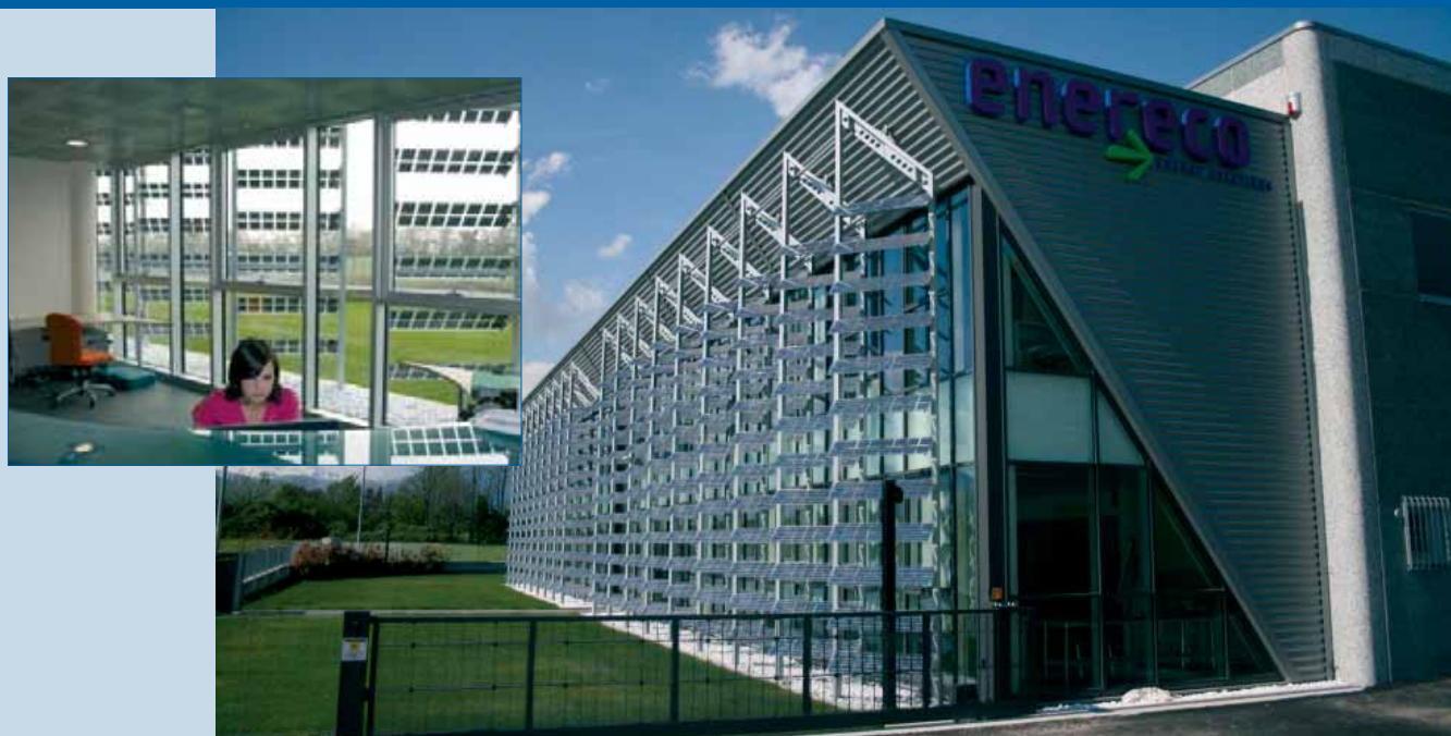
Fig. 1 and Fig 2 – 8,64 kWp PV shields at Sarcedo (VI), Italy.
