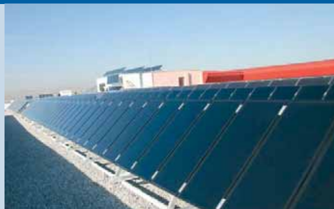
Fig. 2 - 300 kW grid-connected PV system by TEKNOLOGIS in Ankara.
