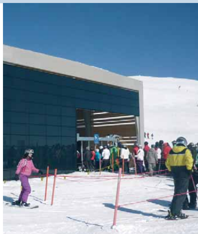
Fig. 6 - 5,1 kWp ARTline PV Façade System, Alp Dado/Laax, Graubünden (photo: SolarMarkt GbmH Aarau).
