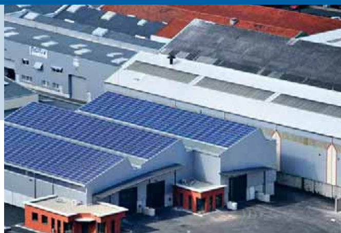
Fig. 2 – PV system integrated into the roof of an industrial building (Loire department) – 111 kW (Photo: Photowatt Bernard & Bonnefond).
