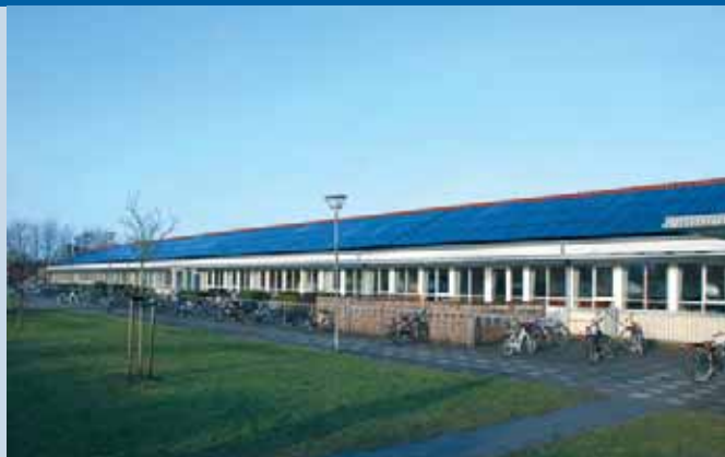
Fig. 1 - A 50 kWp PV-plant on the roof on the public school in Resen in Skive Municipality.
