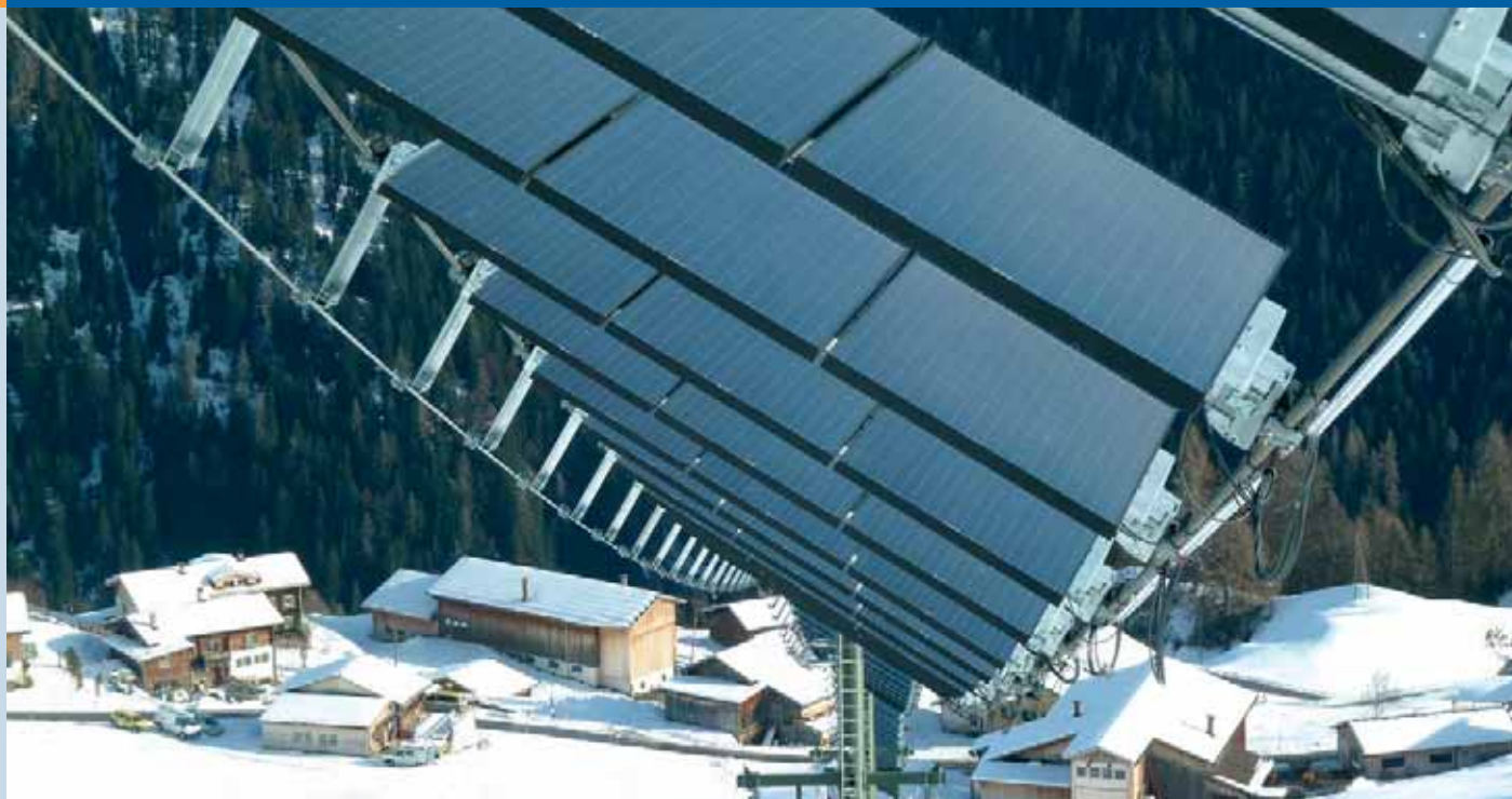
Fig. 4 – 60,3 kWp Single Axis PV Tracker System with Solar Wings on Ski Lift. Tenna, Graubünden (photo: hassler energia alternativa ag).
