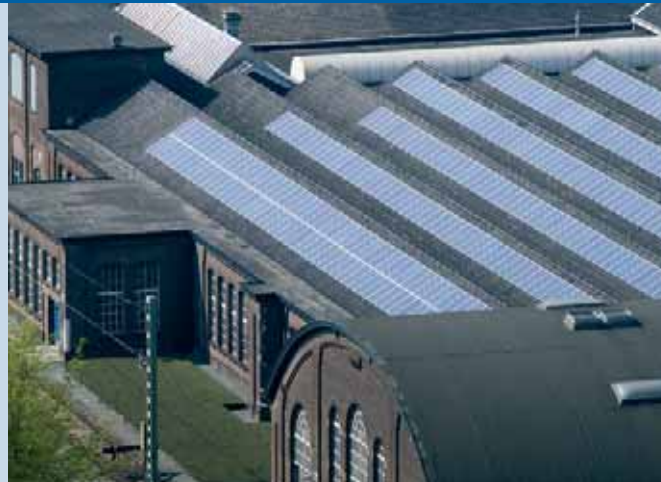
Fig. 4 - Solar modules (189 kWp) on an historical railway workshop in Tilburg. Project Developer: DEC (Photo: Project Developer DEC).
