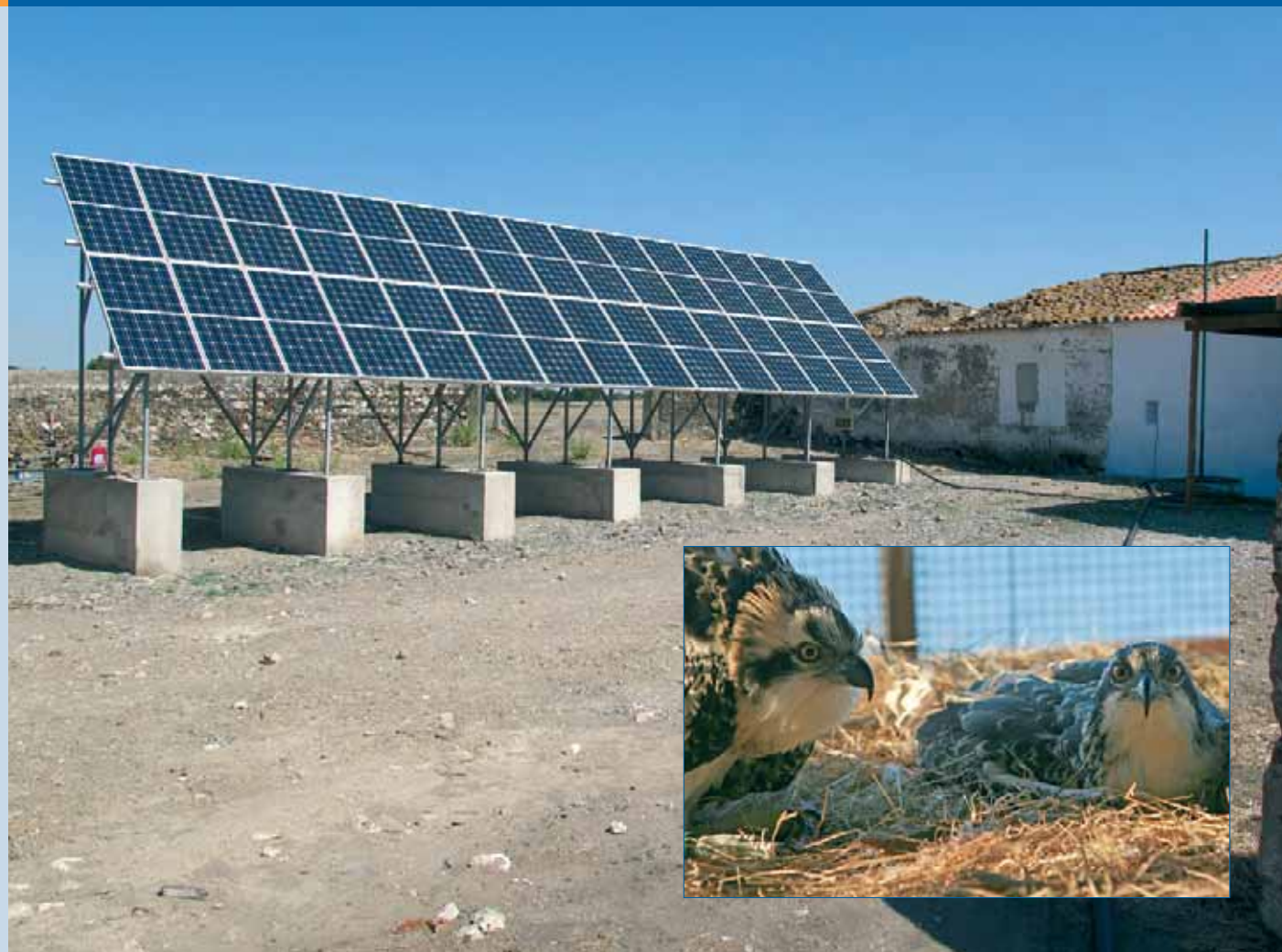
Fig. 3 - Reintroduction of Ospreys in Portugal project - 5,6 kW stand-alone PV system. The system is installed on a private farm in Alentejo and supplies a house-laboratory which has been prepared to monitor the birds (photo: EDP).
