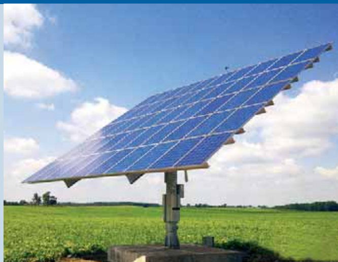
Fig. 1 - Dual Axis solar tracking system developed by Magna Closures Advanced Energy Systems in the province of Ontario, Canada (Photo: Andrew Bowerbank).
