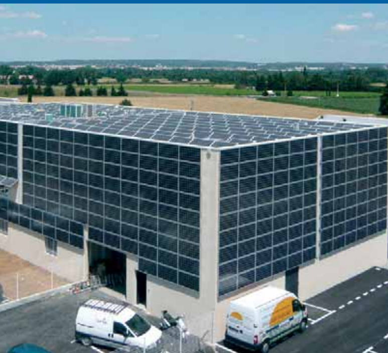
Fig. 1 – PV System integrated to a tertiary building (Gard department) – 86,5 kW (Photo: SETA ENERGIES).
