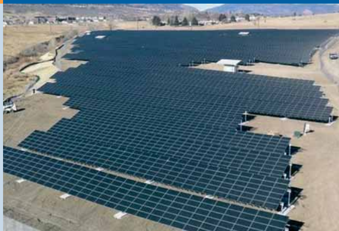
Fig. 5 – 2 MW PV system at U.S. Army Fort Carson, NREL Photographic Information Exchange (Photo: NREL).
