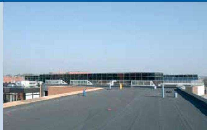
Fig. 2 - Skive Raadhus: CdTe modules used for visual covering of ventilation equipment on the roof of the city hall in Skive.
