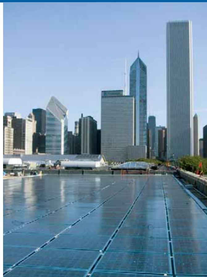
Fig. 1 - 130,6 kW PV system located at Art Institute of Chicago, IL, USA (Photo: Spire Solar Chicago).
