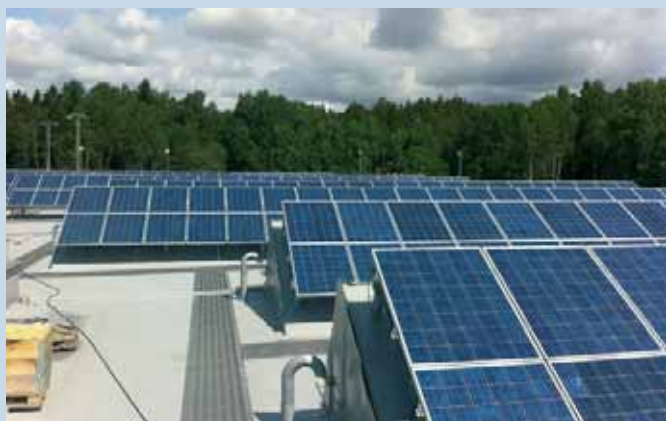
Fig. 3 - Stockholm's largest installation began operating in 2011. 123 kW of solar cells bring extra power to a bus depot in Gubbängen (Photo: Energibanken).
