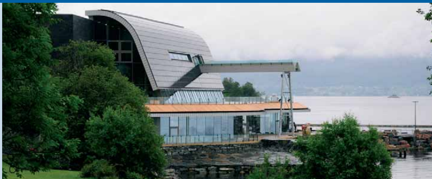
Fig. 1 - Oseana: Inaugurated in June 2011. The building has the largest BIPV system (60 kWp) in Norway so far. The curved wall-roof construction is covered with PV modules (Photo: P. Bernhard).
