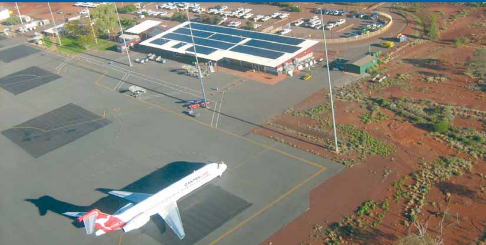
Fig. 1 - 120 kW PV system at Newman Airport, Pilbara, WA, using First Solar modules and installed by Commsolar (Photo: Commsolar).
