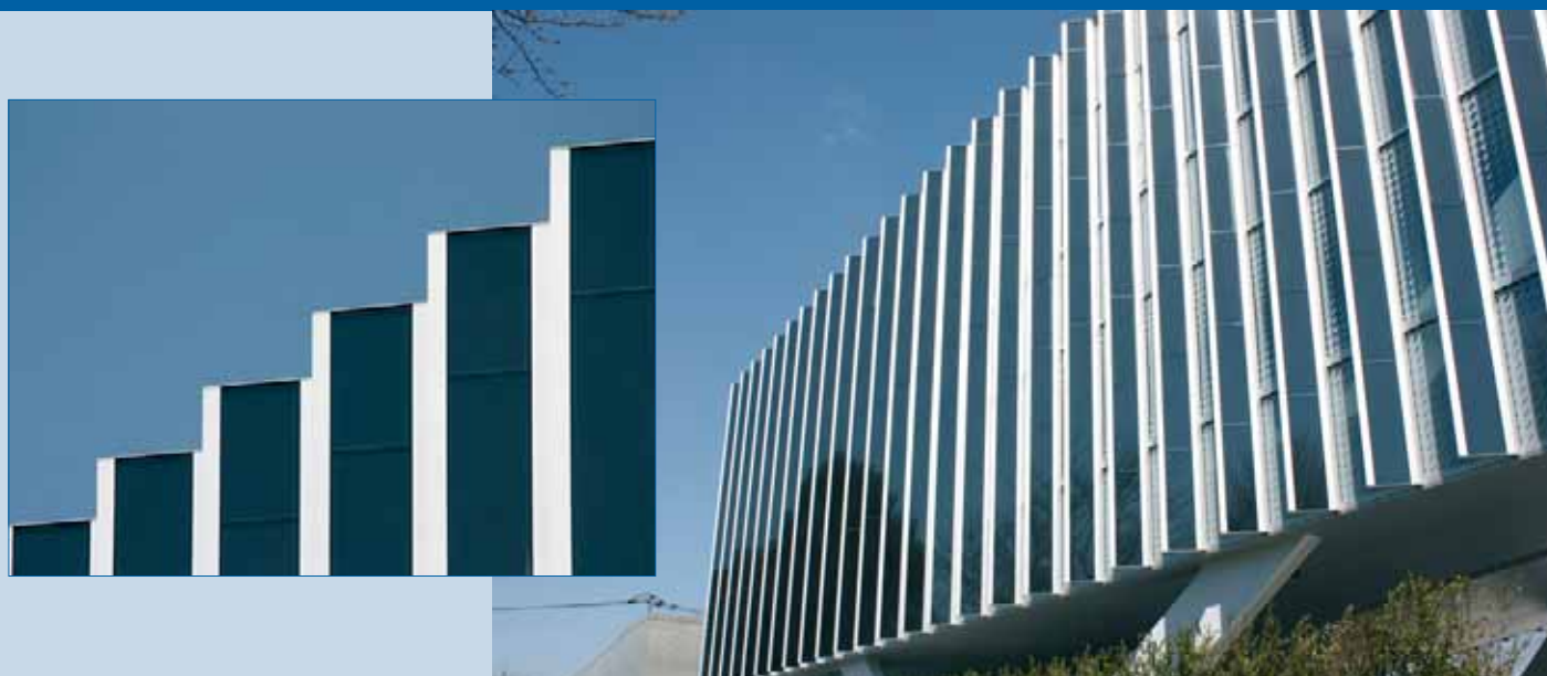
Fig. 1 - Tokyo Institute of Technology Ookayama Main Library (Ookayama, Meguro-ku, Tokyo). Louver: 12 kW, CIS PV module (by Solar Frontier).
