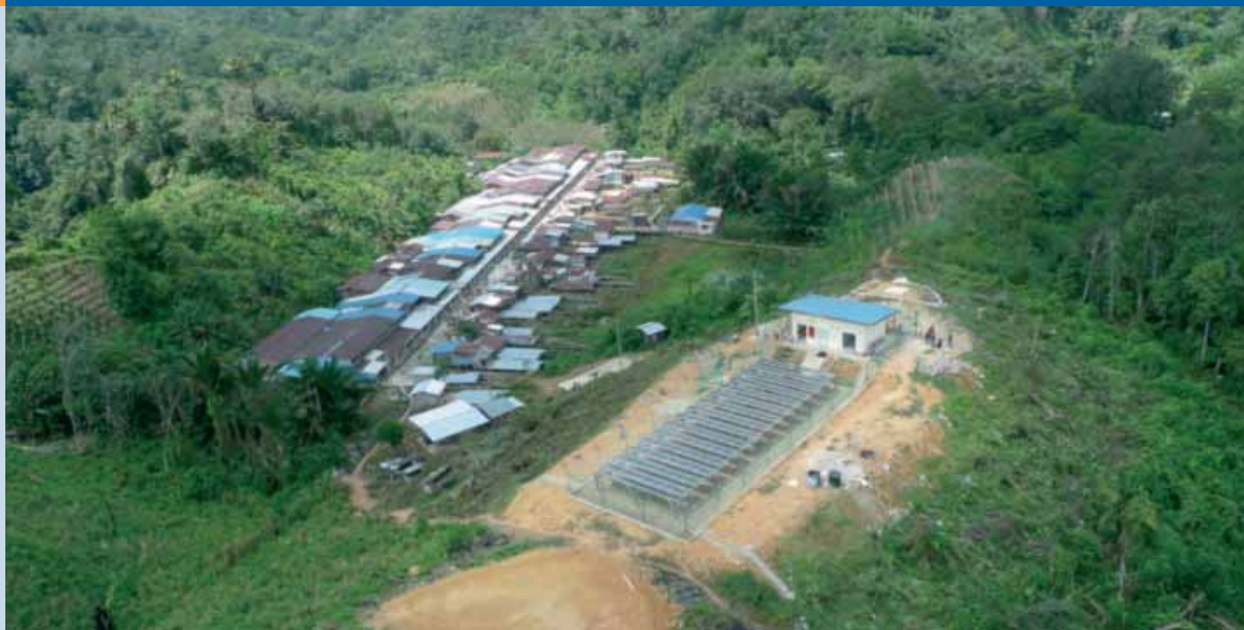
Fig. 3 - PV hybrid system in Kerapa Spak, Malaysia. 21,60 kWp. 3 Sunny Island 5048, 1 Multicluseter-Box, 4 Sunny Boy 5000TL (Photo: SMA Solar Technology AG).
