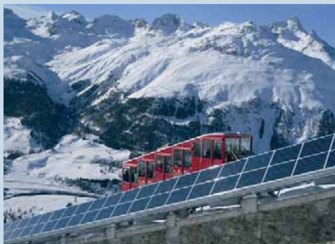
Fig. 3 – 64 kWp PV Installation on the Muottas Muragl Cable Railway. Samedan, Graubünden (photo: gvz-rossat ag/sa).
