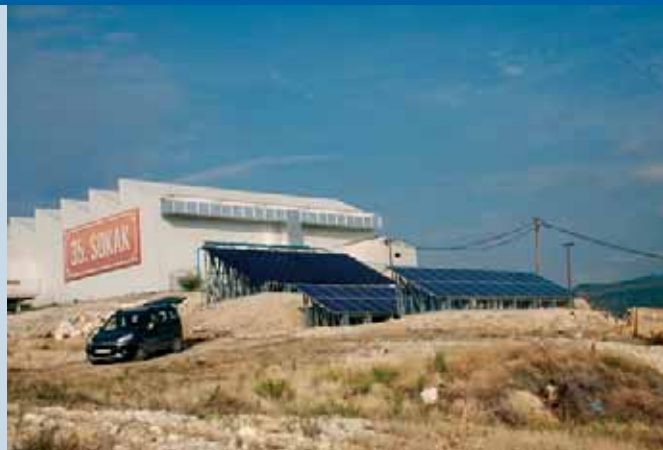
Fig. 6 - 15 kW grid-connected PV system by Girasolar Ltd. in Izmir.
