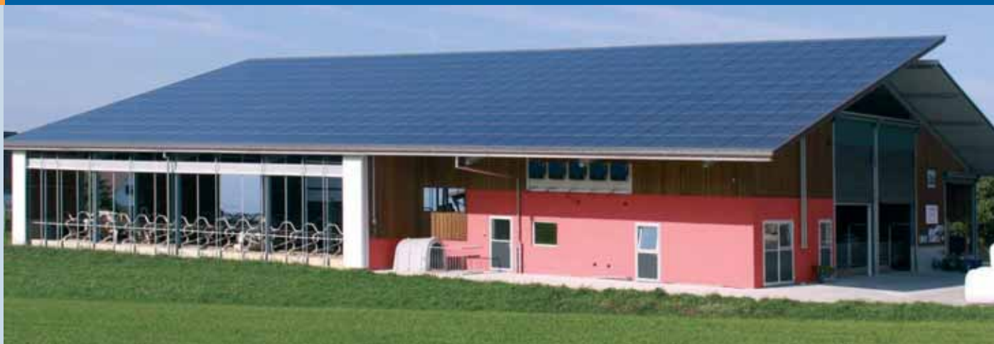
Fig. 2 – 81,18 kWp Integrated PV Trapezoidal Roof System. Mörschwil, St. Gallen (photo: ALUSTAND®).
