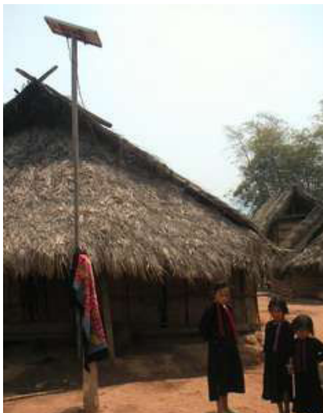
Solar home system in Lao PDR
