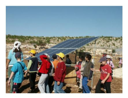
Figure 4: *Environmental-Education Park*, near Modi'in Israel. A hybrid PV-wind system is the sole method of powering inter-active exhibits, in line with their ideology. The systems consists of eight 100 W panels and a small wind turbine (not pictured). [Provided by Solarpower].
