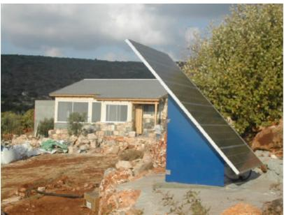
Figure 3: Village of Klil, a solar village established about 20 years ago, was never connected to the grid. The families need to continue adding power for larger families and new needs, with PV still filling a major niche. This new home shows an installation of Wp, 400AH/12V batteries and a 1500W Inverter [Provided by Interdan Co.]
