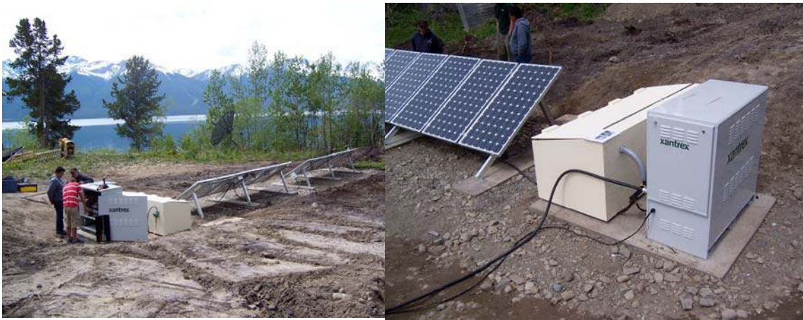
Fig: 3 The Xantrex Hybrid Power System reduces First Nations generator fuel consumption and increases reliability at a remote site (Photo credit Xantrex)
