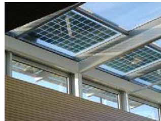
Fig. 2: Skylight systems at the Fred Kaiser Building, UBC, British Columbia, featuring a grid-tie 7 kW BIPV. (Photo credit Carmanah)
