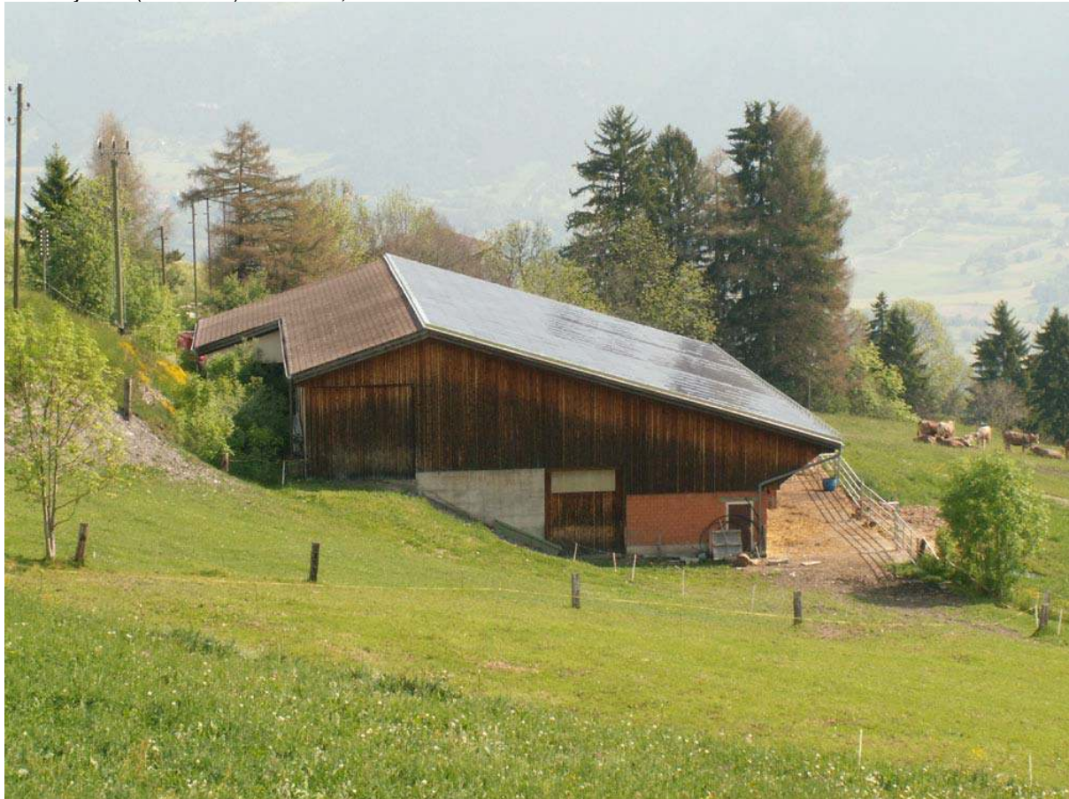
BIPV System (SOLARIF) in Flerden, Switzerland
