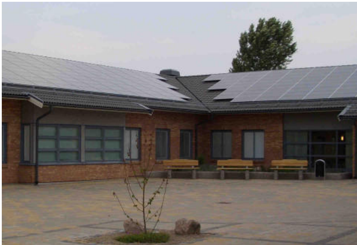
Figure 2: The primary care centre in Fjärås, which was the largest PV system in Sweden when it was inaugurated early in 2006.
