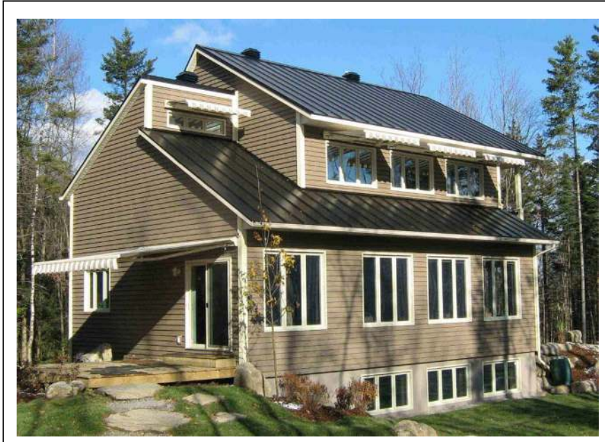
Figure 1: A 3 kW roof-integrated PV system on the ÉcoTerra™ net zero energy house, Alouette Homes, Eastman, Quebec (Photo credit – The Solar Buildings Research Network and Alouette Homes)
