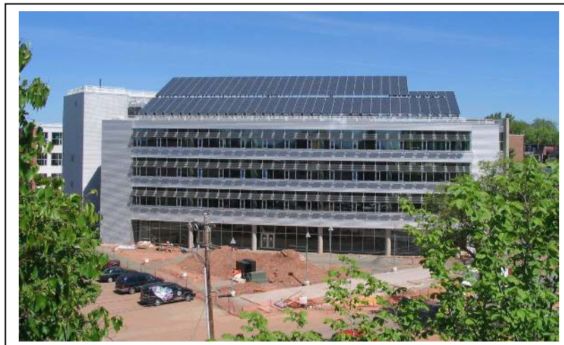
Figure 2: Newly installed 108 kW grid-tie solar power system on the Jean Canfield Government of Canada Building, Charlottetown, PEI (Photo credit – Carmanah Technologies Corp.)
