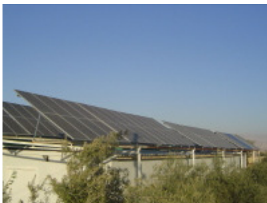
Hazeva, farm for decorative fish. 10 kWp grid-connected system (Photo credit: Interdan Ltd.)
