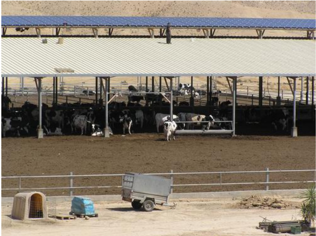
Tene Farm – installation of Israel's current largest grid-connected PV, designed to be 50 Kw. This is an addition to the sun tracking system at the same location reported last year (Photo credit: SolarPower)
