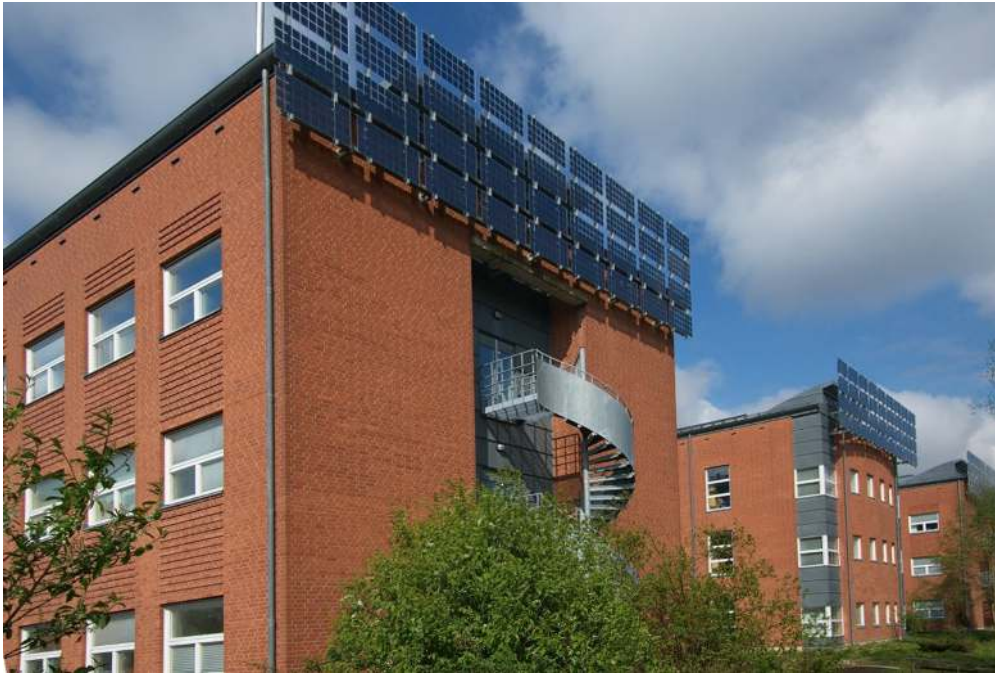
Figure 4: The installation at Ekologihuset, Lund University, comprises PV in several different positions. Here frame-less modules mounted in front of a south-facing façade.
