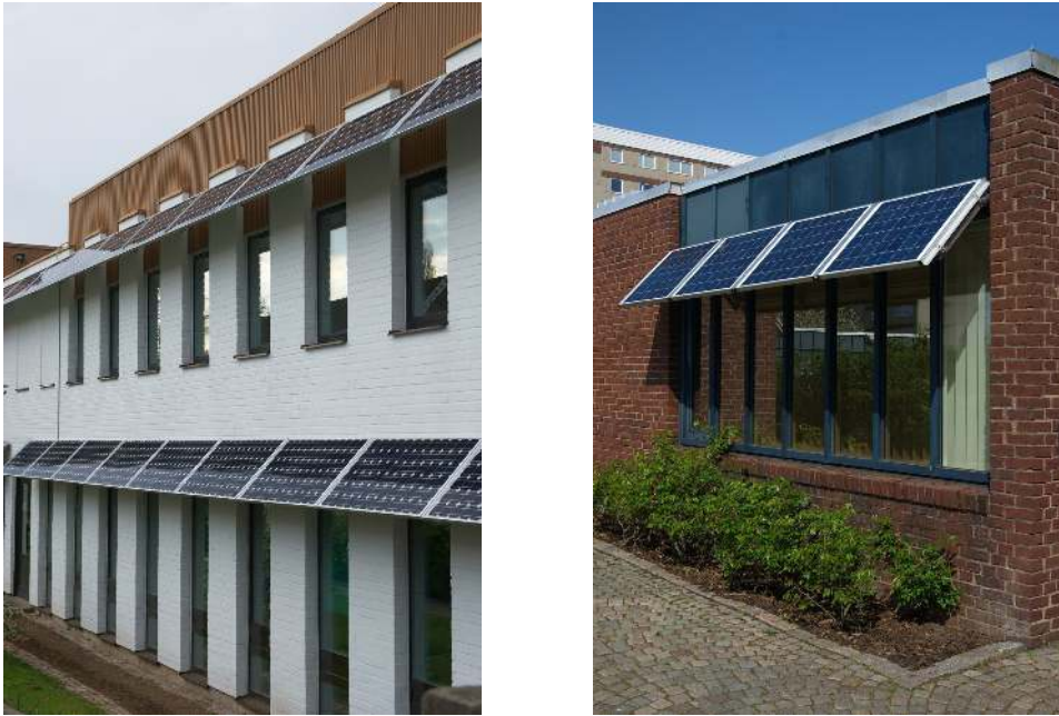
Figure 5: The Swedish Church has installed PV on several congregational buildings; here two examples from Malmö are shown.
