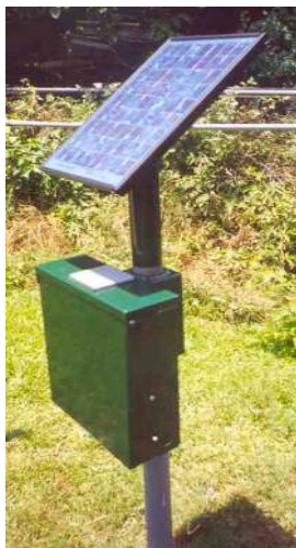
a) Solar electricity used for irrigation control. b) Telecommunications station in Arizona.
