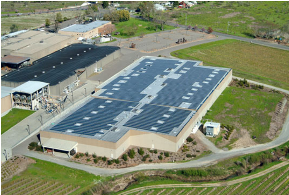
A 766-kW PV system on the roof of the Rodney Strong Vineyards building in California.
