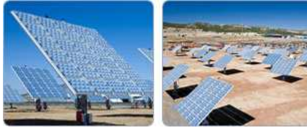
Figure 20 High Concentration PV plant (200 kW) installed in Puertollano for the Institute of Concentration Photovoltaic Systems (ISFOC)
