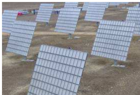
Figure 22 PV plant of 2 MW that consist of both silicon flat modules and concentrator PV modules mounted on tracking systems (Solúcar la Mayor, Seville)
