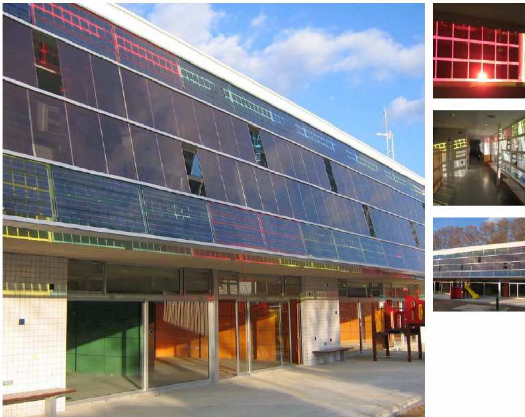
Figure 15 Façade of the a kindergarten, installed in 2008, Sant Celoni (Barcelona) 7,5 KWp
