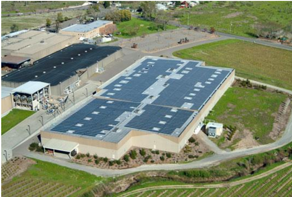
Figure 3: A 766-kW PV system on the roof of the Rodney Strong Vineyards building in California.
