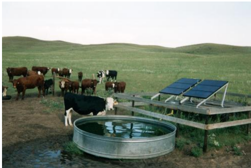
c) PV is often used for water pumping on farms and ranches in the United States.
