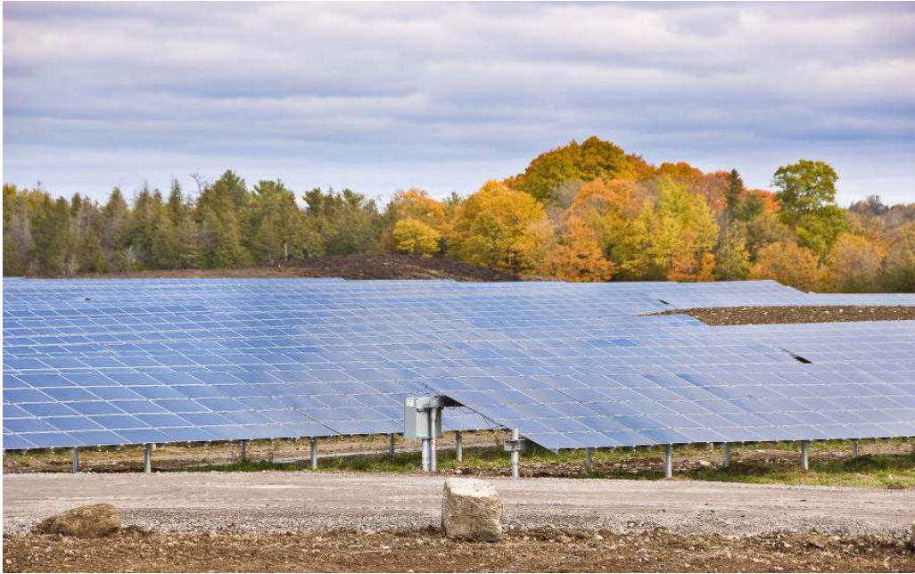
Figure 1: SunEdison's and SkyPower Corporation's 9.1-megawatt (MW) First Light Solar Energy Park in Stone Mills, Ontario, and the largest solar energy park built to date in Canada. (Photo credit: Dave Turcotte, CanmetENERGY)
