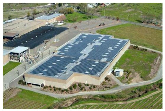
Figure 4. A 766 kW PV system on the roof of the Rodney Strong Vineyards building in California (Photos courtesy of Rodney Strong Vineyards)
