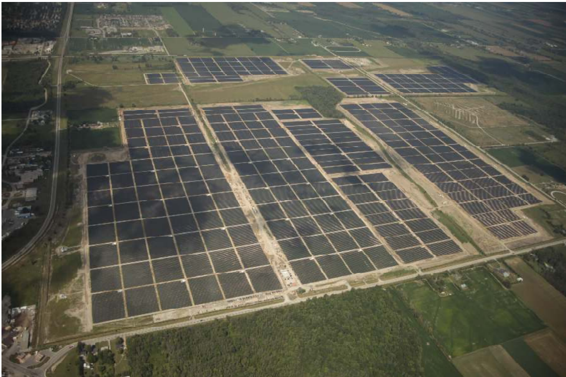
Figure 1: Enbridge and First Solar's 80 MW Sarnia Solar Project, the largest operating photovoltaic facility in the world in 2010 (Photo courtesy of Enbridge Inc.)
