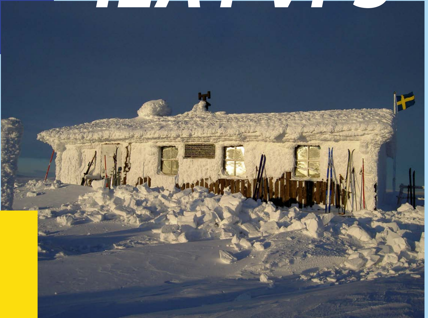
An off grid-system with a module from Eco Supplies AB at Dundret, Gällivare in northern Sweden. Courtesy of Eco Supplies AB
