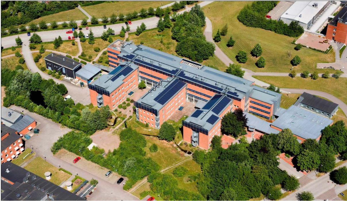
Figure 4: The 767 m 2 big photovoltaic installation on Ekologihuset at Lund University is expected to produce about 70 000 kWh annually and won the award as the photovoltaic installation of the year in 2010. (Courtesy Fojab arkitekter)
