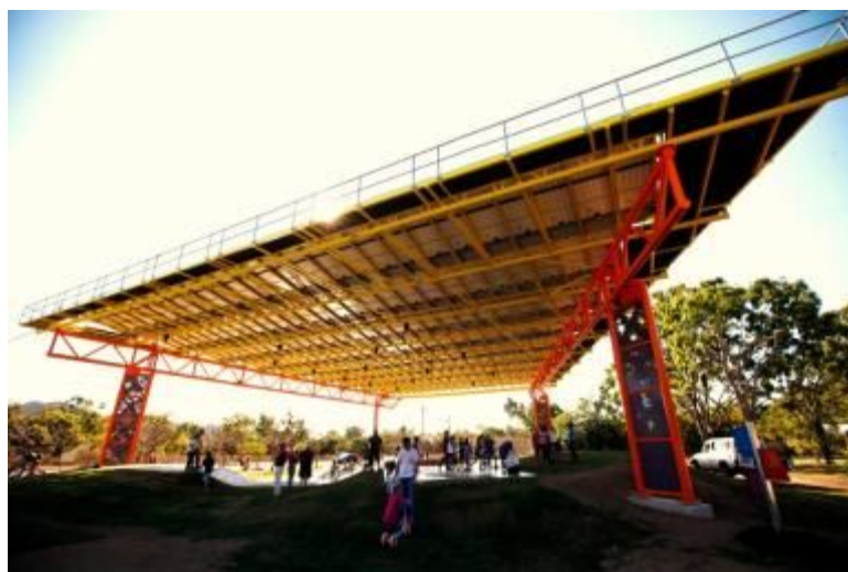
Figure 2: Solar skate park on Magnetic Island with a 100 kW PV array which provides lighting in the evening, but doubles as shade during the day.
