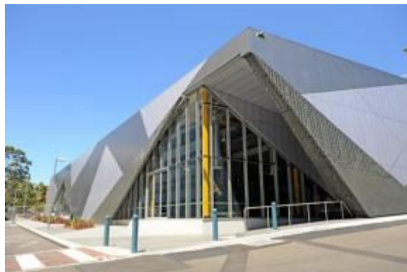
Figure 10: Solar Industrial Research Facility
