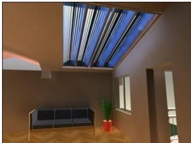
Figure 9: Building Integrated roof-top hybrid concentrators at ANU (courtesy of Chromasun).
