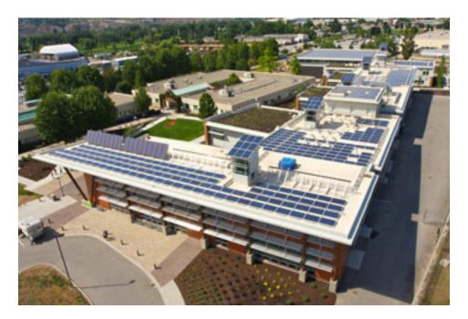
Figure 1. This large 260 kW rooftop solar Photovoltaic system was installed at the Okanogan College in British Columbia in 2011. (Photo: Skyfire Energy)
