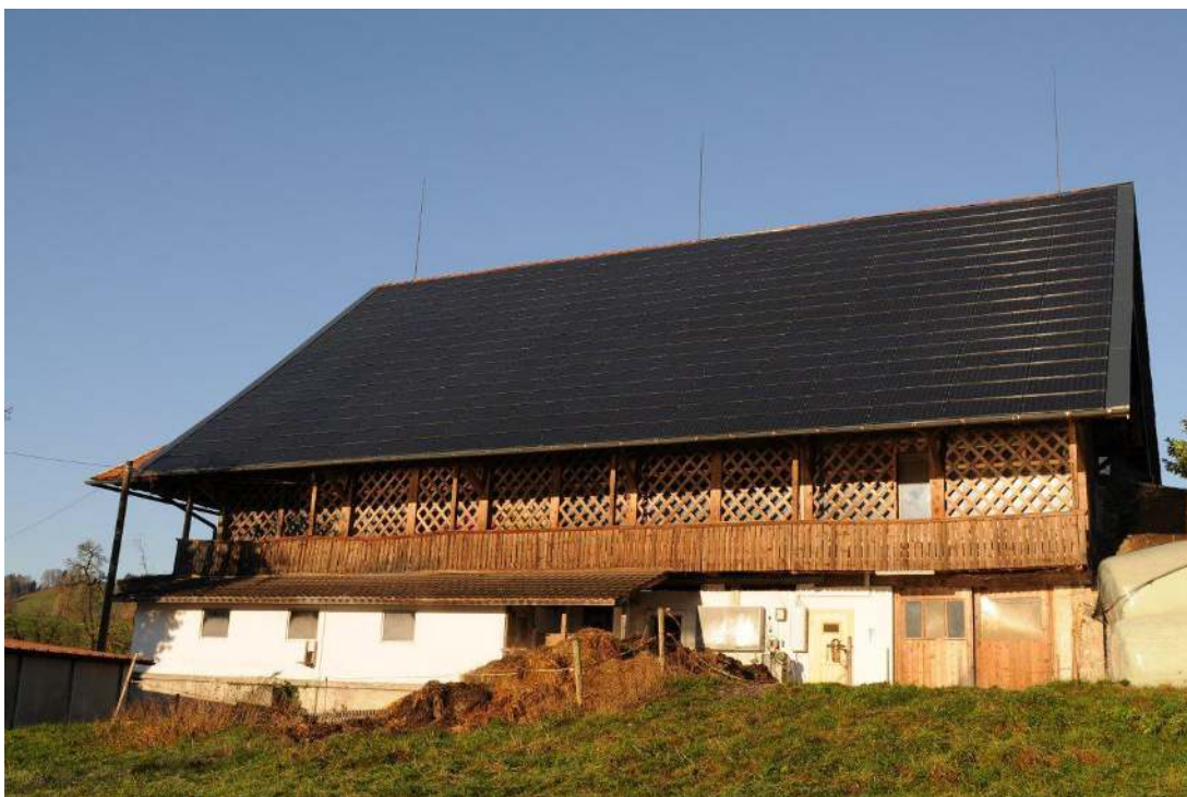
Picture 2 Courtesy BE Netz AG
