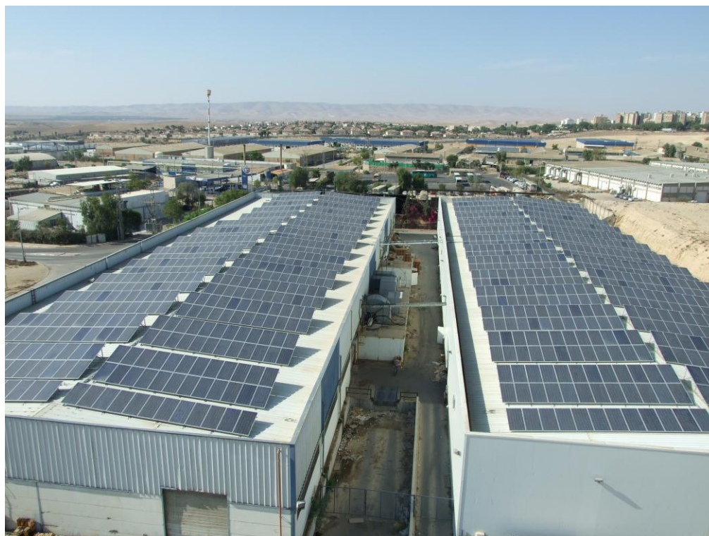
Figure 1: : Faran 400 kWp – roof top system installed on top of a large dairy farm. (Photocredit: Solarpower)
