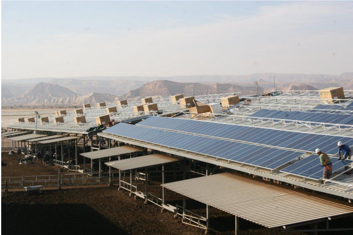
Figure 2: Faran 400 kWp – roof top system installed on top of a large dairy farm. (Photocredit: Solarpower)
